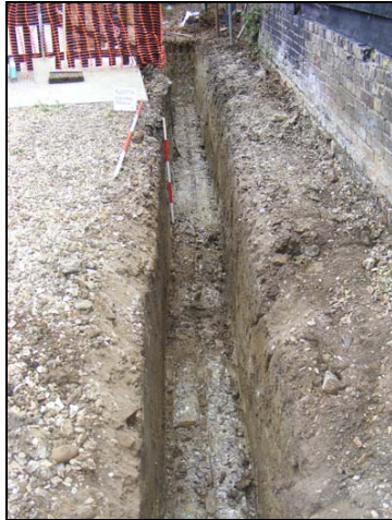
Plate 51: Trench to the rear of the stable
