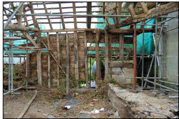
Plate 34: East Barn: west end of south elevation
