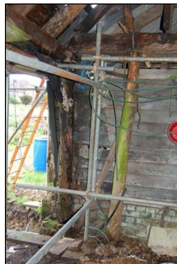
Plate 12: Pole posts in the northeast corner
