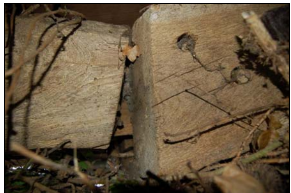
Plate 18: East Barn: bridled scarf joint
