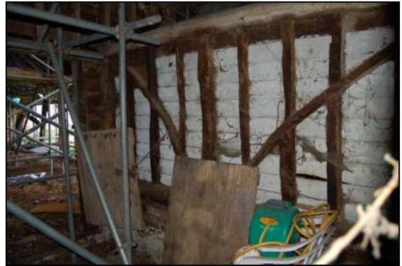
Plate 32: Northern store room: north wall
