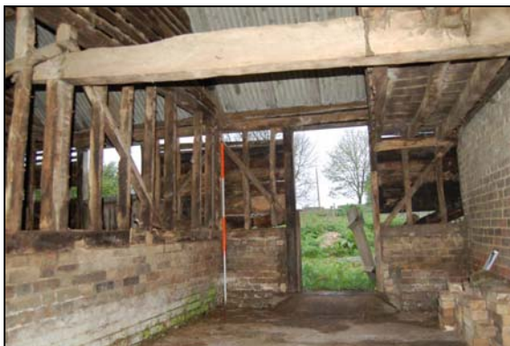
Plate 23: Stable 1: looking north
