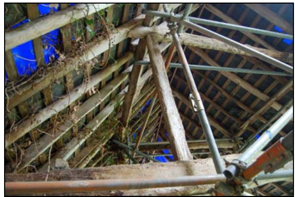
Plate 16: East Barn: queen post & clasped purlin
