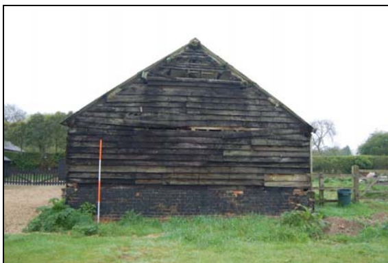
Plate 5: The stables: east elevation
