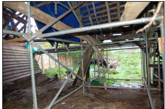
Plate 10: East Barn, Bay 4: looking south
