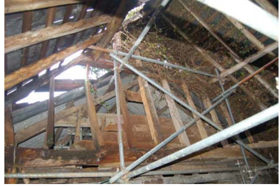
Plate 14: East Barn: east wall
