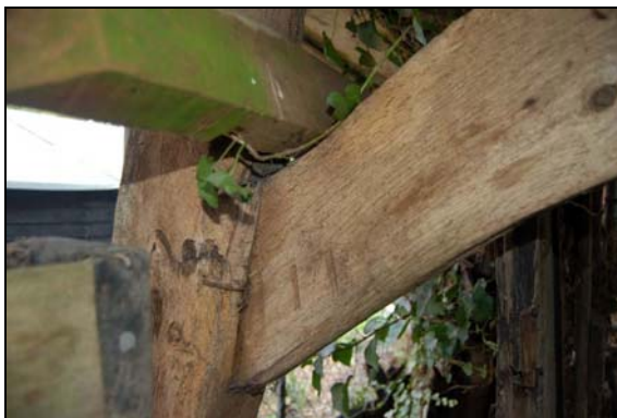
Plate 17: East Barn: carpenters' assembly marks
