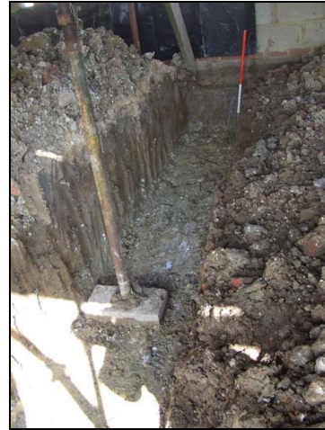
Plate 50: Footing trench in the stable
