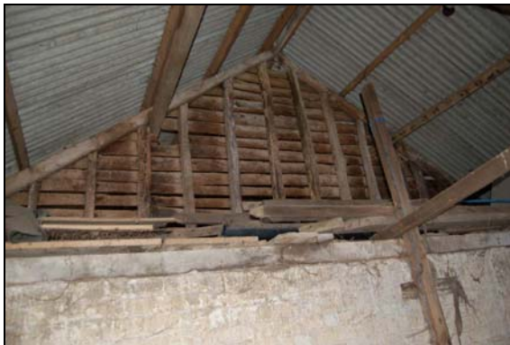
Plate 21: Tack room: west wall
