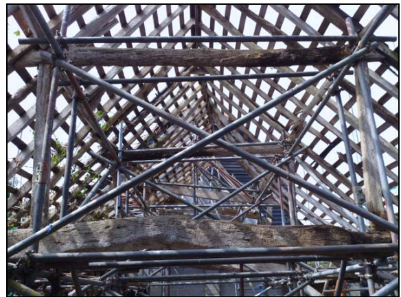
Plate 42: East barn, truss and bare rafters
