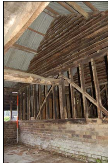
Plate 28: Truss 1 from the northeast
