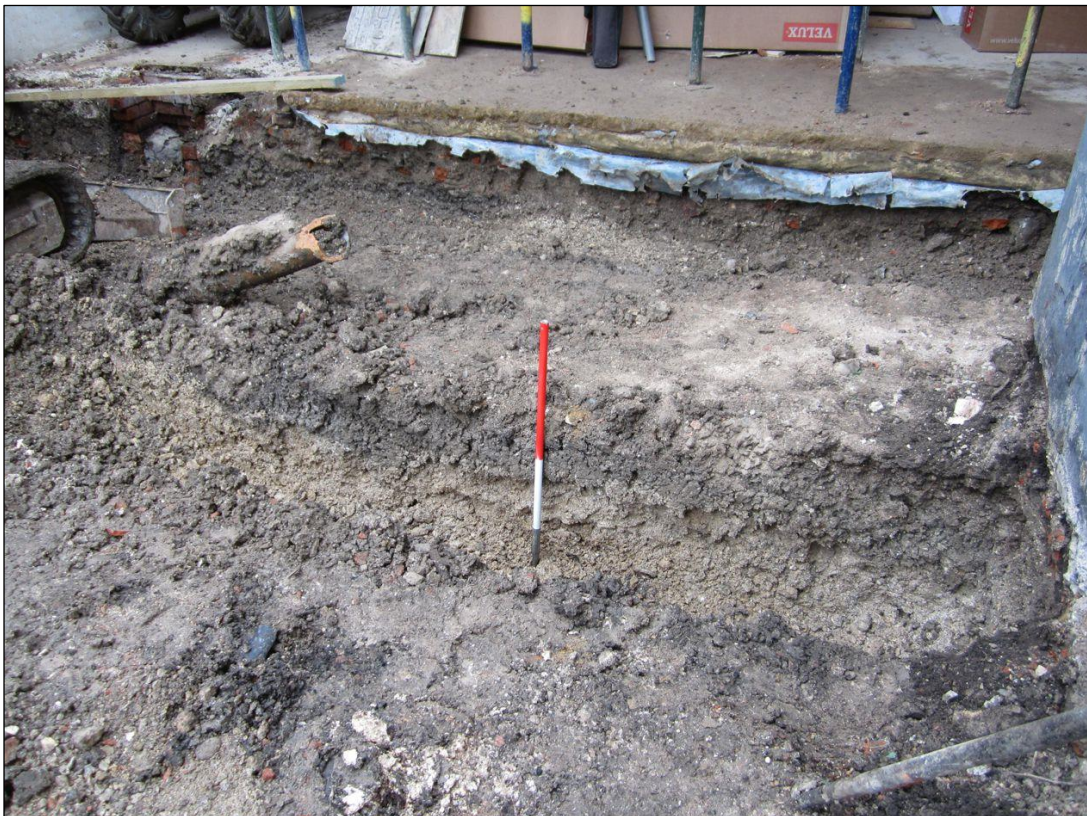
Plate 5: Stratigraphy revealed in footing trench
