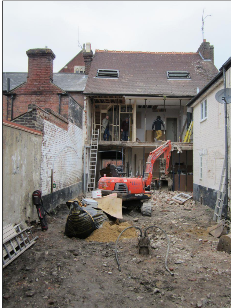
Plate 2: Site at start of watching brief, looking west
