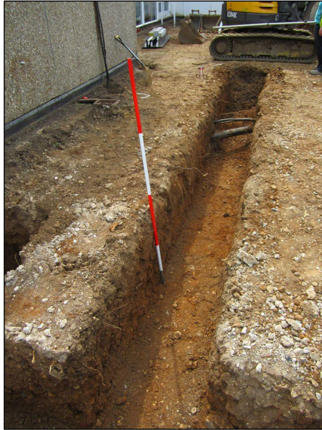
Plate 3: Footing trench for extension
