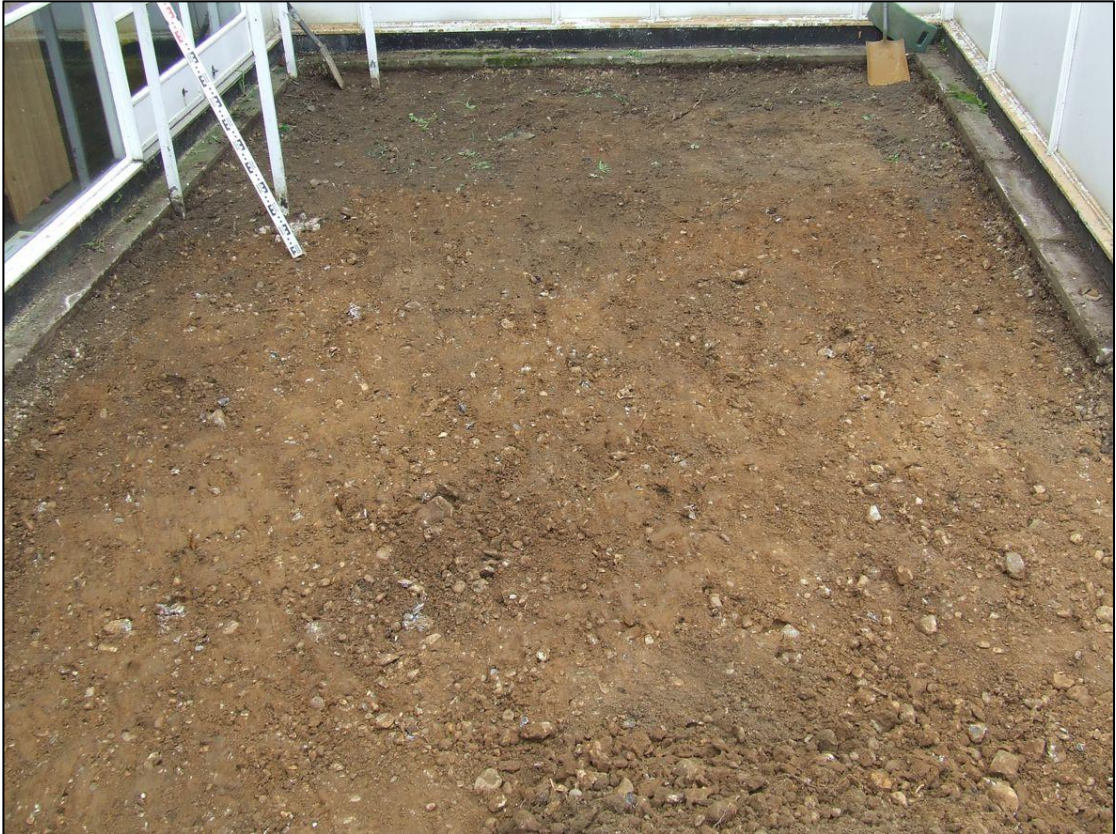
Plate 2: Detail of extension area after stripping
