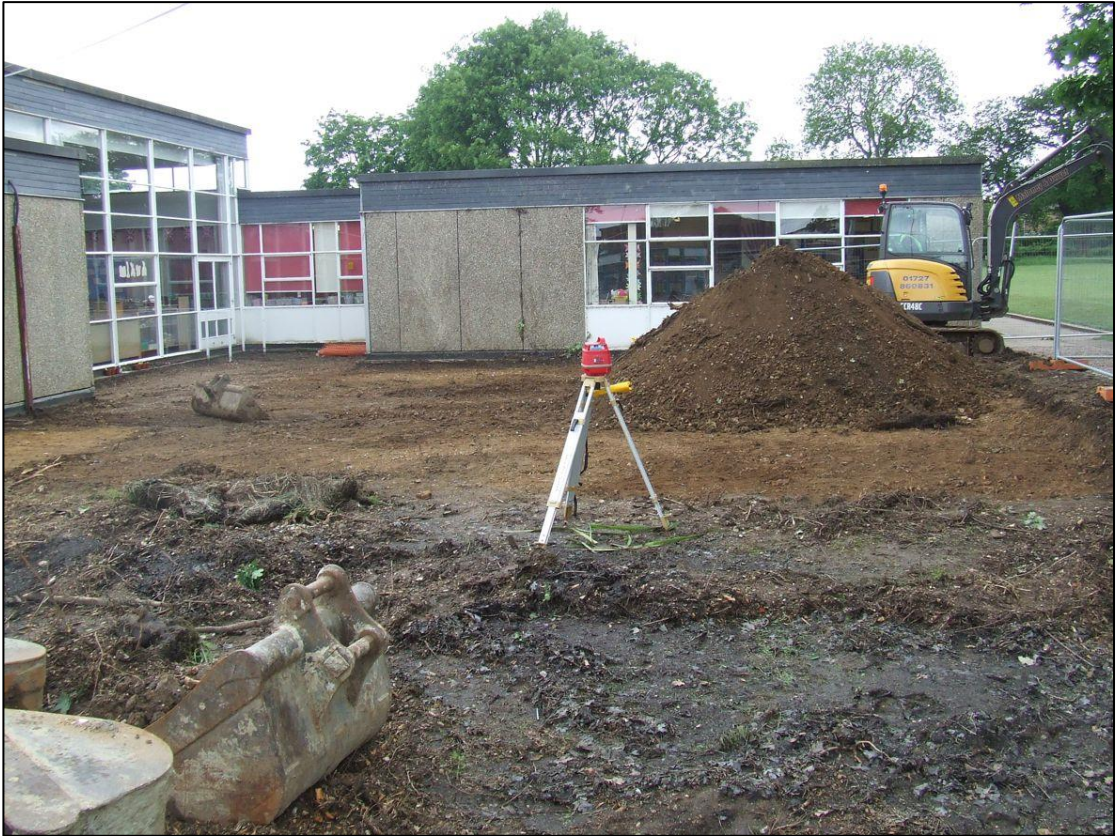
Plate 1: Extension area during stripping
