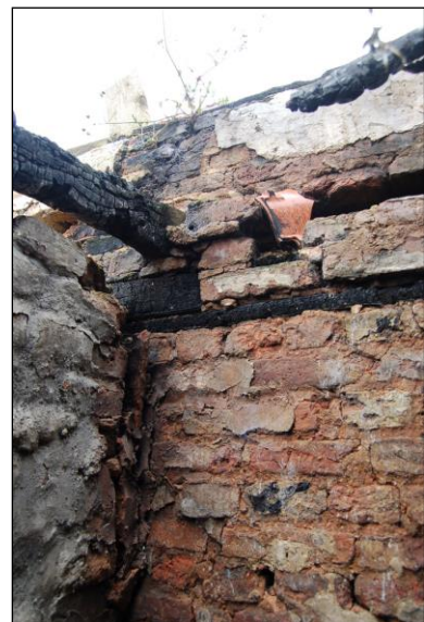
Plate 24: Room G3: northwest corner detail
