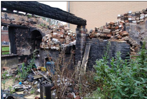
Plate 9: Room G1a: west wall
