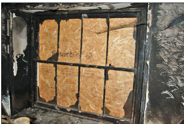
Plate 17: Room G2: window detail
