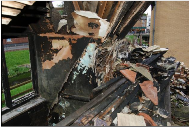
Plate 31: First floor: south wall detail showing dormer timbers & reed packing
