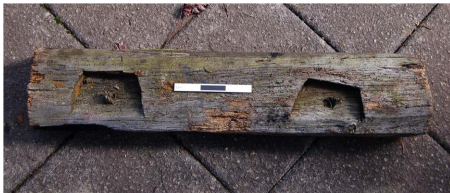
Plate 35: Section of the northern wallplate and rafter seatings
