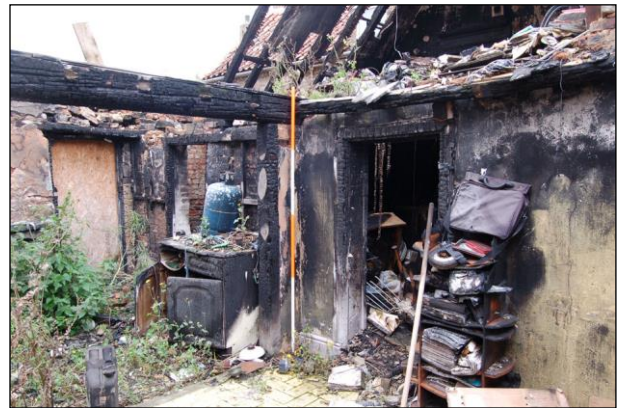
Plate 10: Room G1a: east wall
