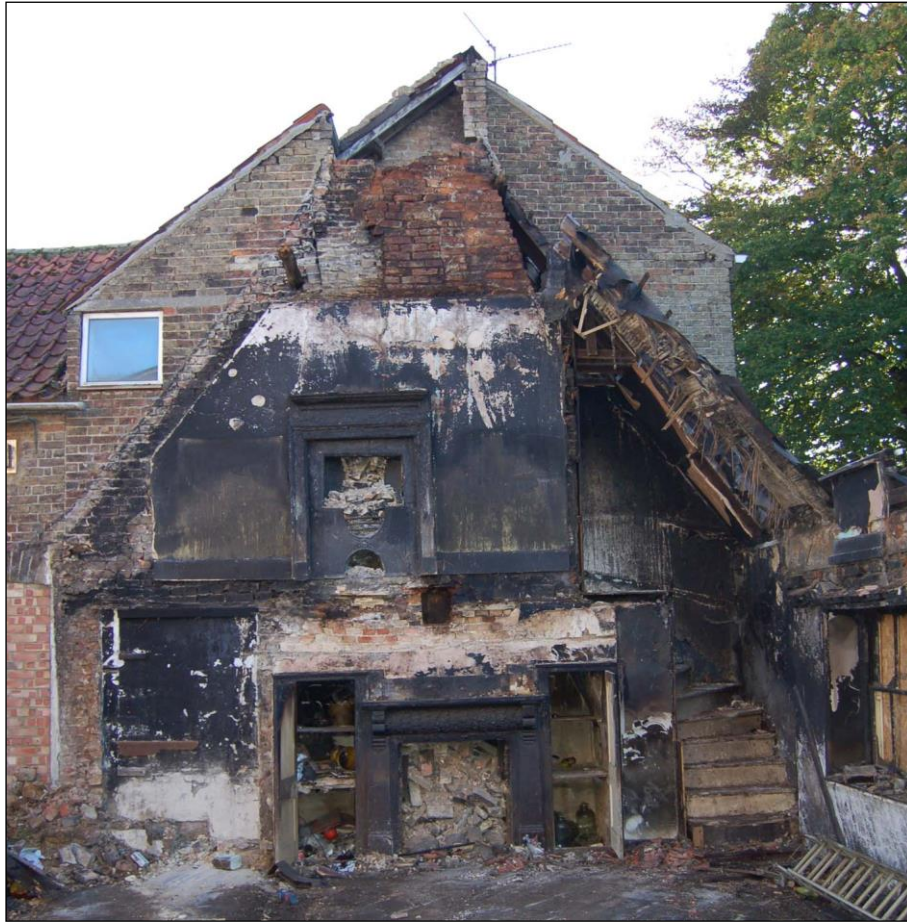
Plate 36: East wall after the first stage of demolition
