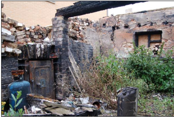
Plate 13: Room G1b: west wall
