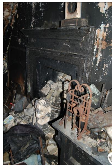
Plate 30: First floor: east detail
