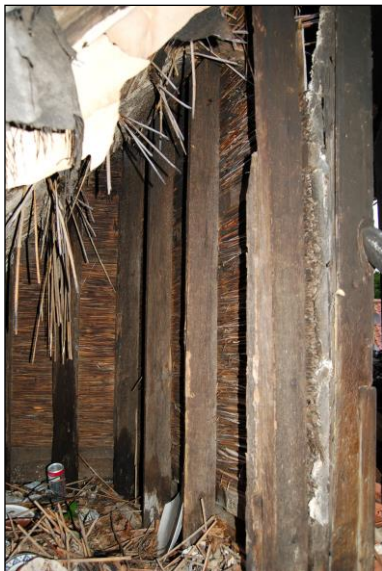
Plate 27: Area above the stairwell
