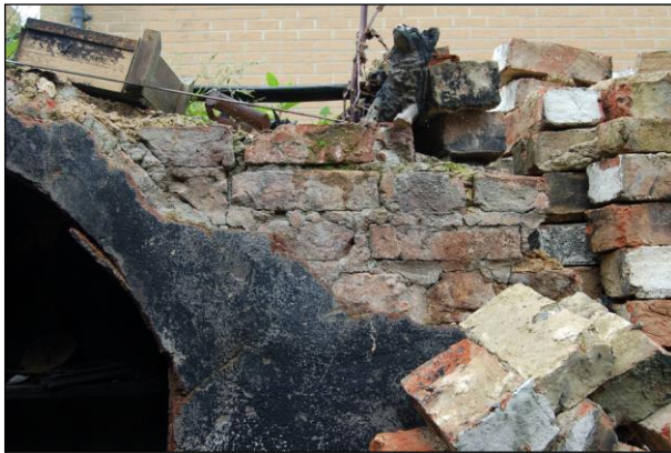
Plate 15: Exposed bricks in the west wall of Room G1a
