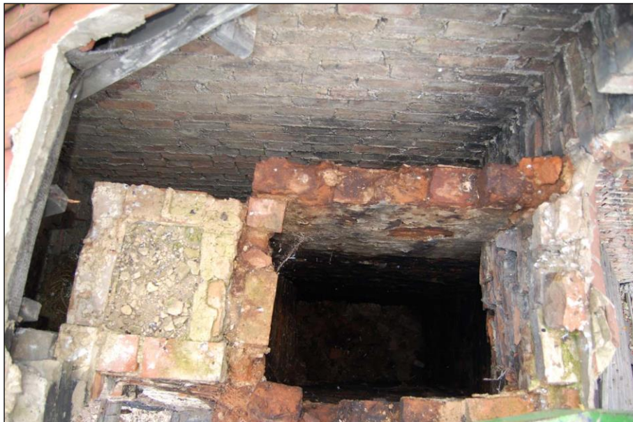
Plate 39: Top of the chimney stacks as seen from a cherry picker
