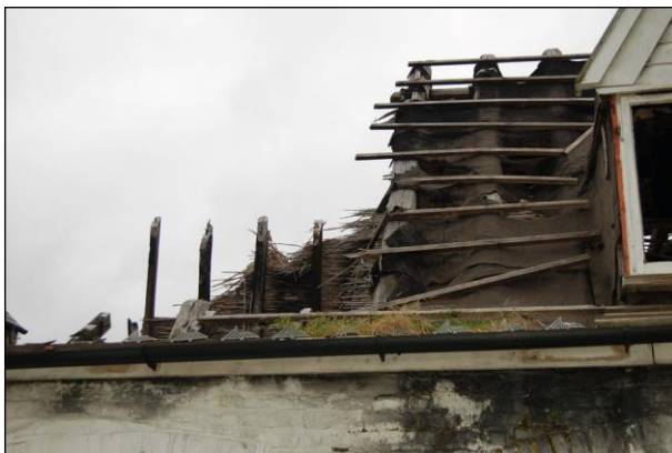
Plate 33: Rafters on south side of the building
