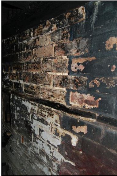
Plate 25: Room G3: south wall detail
