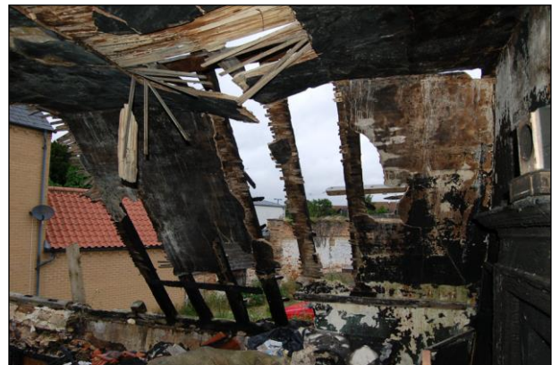
Plate 28: First floor: looking north
