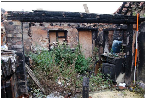
Plate 11: Room G1b: north wall
