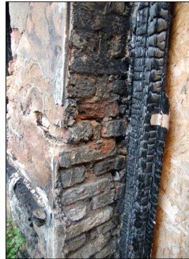
Plate 16: Brickwork in the north wall of Room G1b
