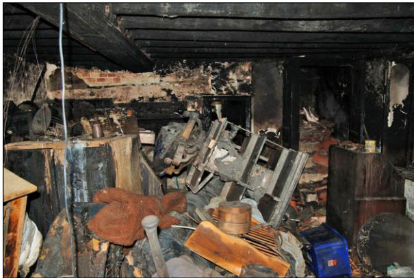
Plate 21: Room G2: east wall
