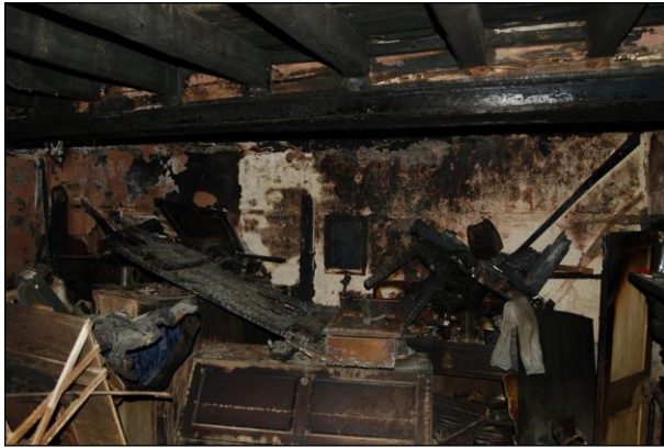
Plate 19: Room G2: north wall and ceiling joists
