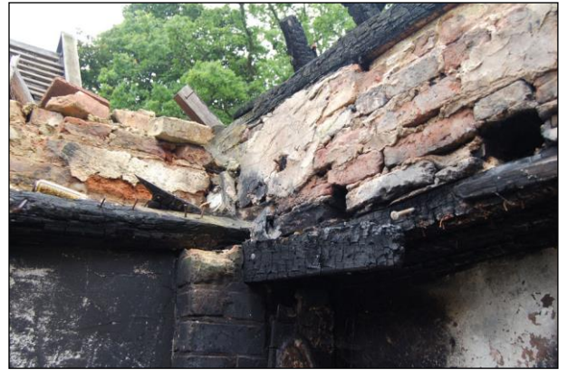
Plate 14: Exposed brickwork in the southeast corner of Room G1a
