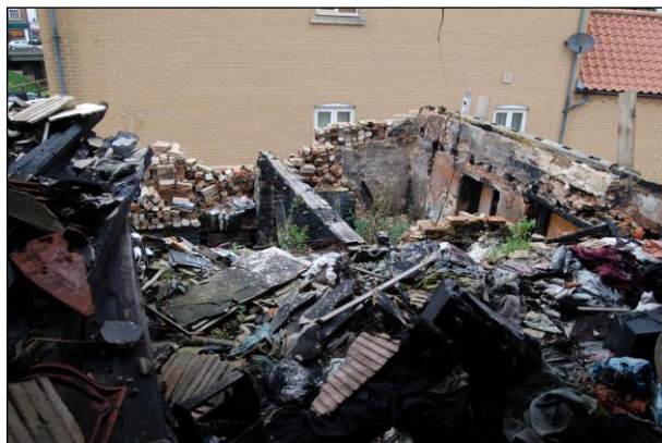
Plate 29: Western end of former first floor
