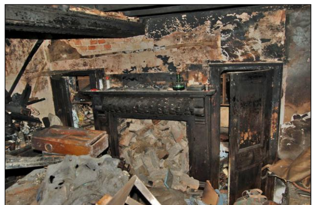
Plate 18: Room G2: east wall
