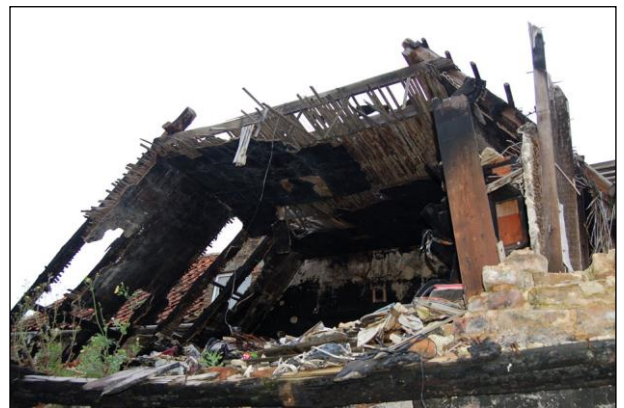
Plate 34: View of the first floor from G1
