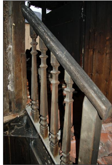
Plate 26: Stair to first floor
