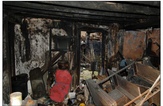
Plate 22: Room G2: west wall
