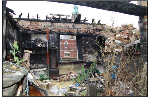
Plate 8: Room G1a: south wall
