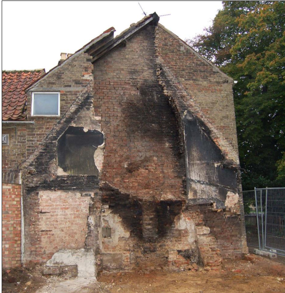
Plate 38: East wall after the final stage of demolition
