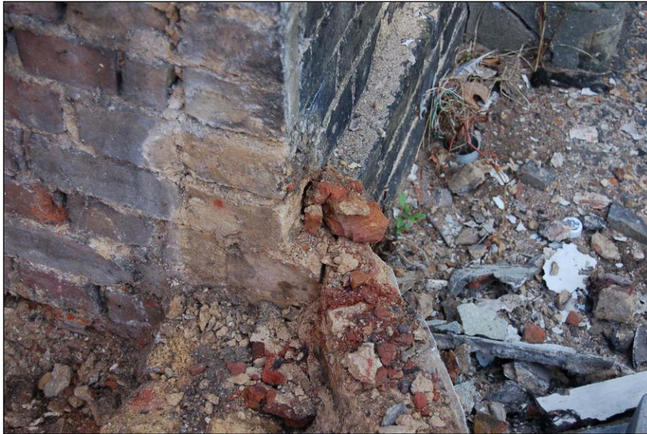
Plate 42: Detail of the south wall overlapping the southwest corner of number 8
