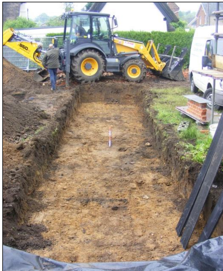
Plate 5: Trench 3, facing north-east
