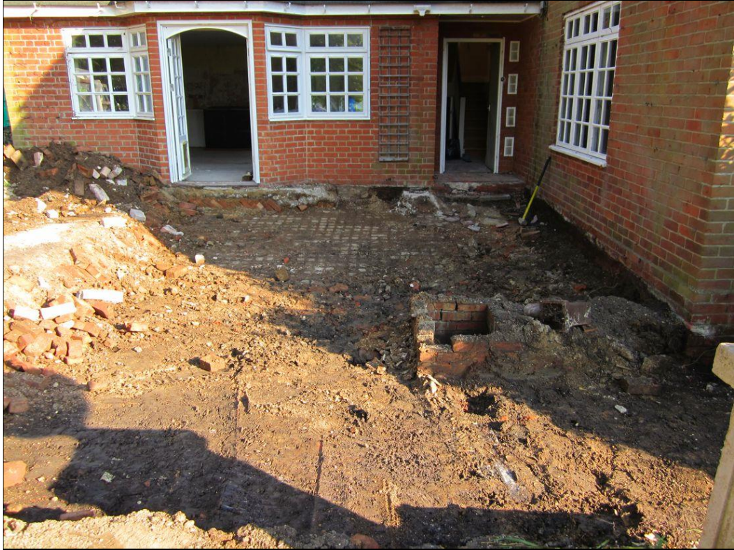
Plate 1: Development area after removal of turf & modern surfaces
