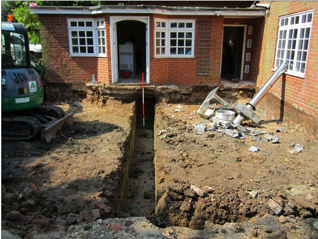
Plate 3: General view of the site on completion of footing trenches
