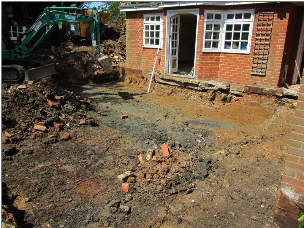
Plate 2: Ground reduction in progress, looking north-west
