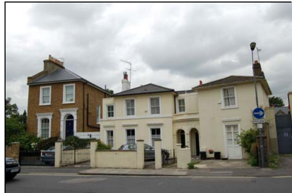
Plate 40: Houses to the north of 6 Lime Grove
