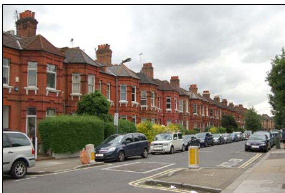
Plate 41: Street view of the east side of Lime Grove
