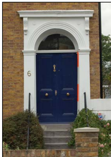
Plate 3: Front door detail
