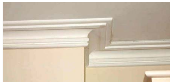
Plate 34: Room S4: cornice detail
