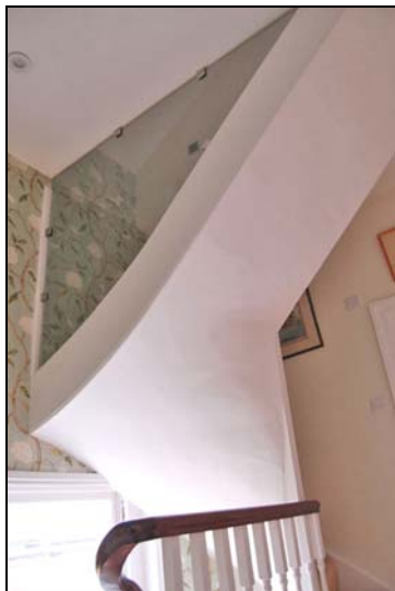
Plate 29: Room S2: upper stair
