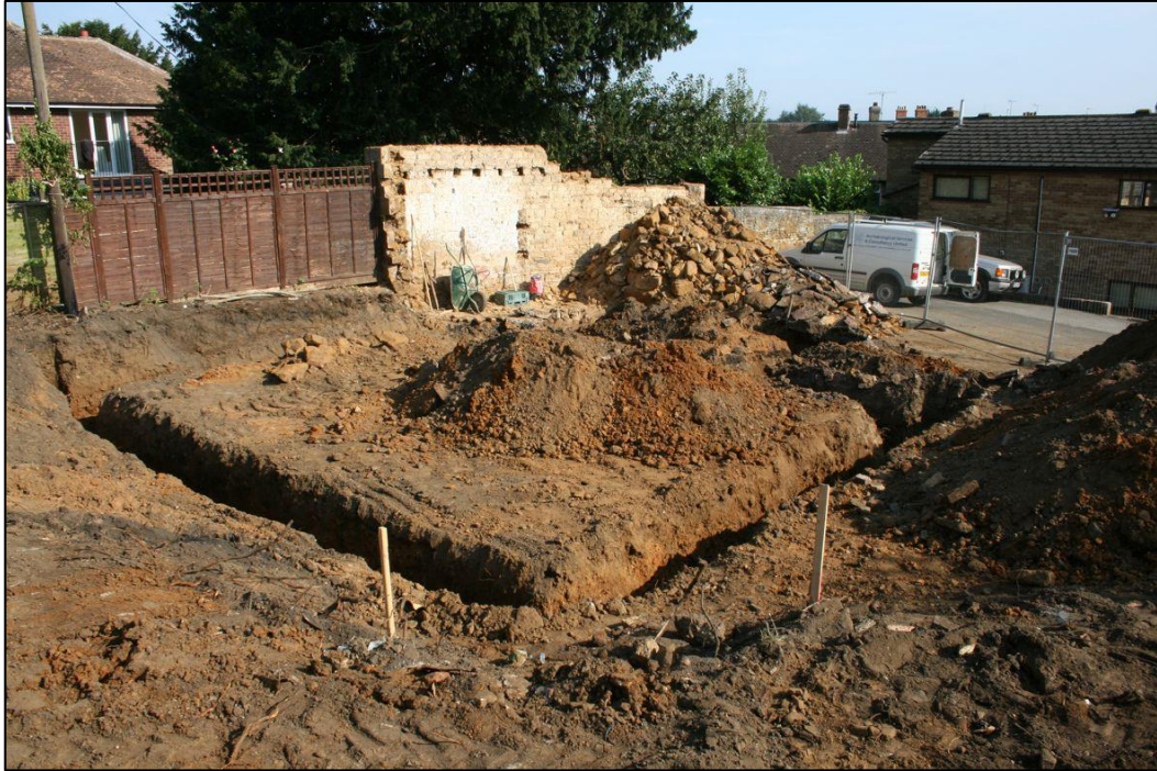
Plate 14: Watching brief: general view of site
