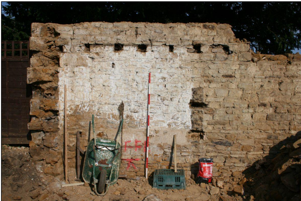
Plate 6: North-west wall: interior elevation, showing row of joist holes
