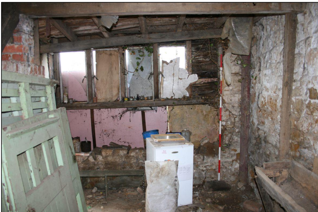
Plate 12: Room 2, looking south-east
