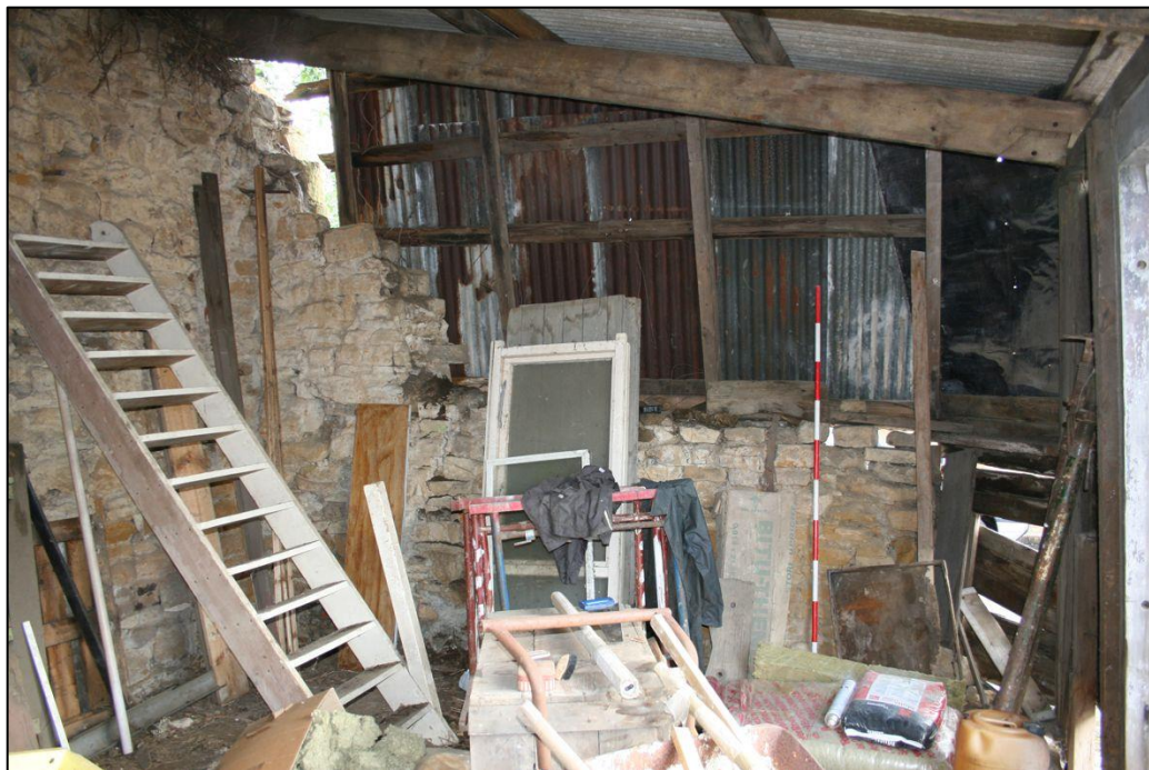
Plate 8: Room 1, looking north-east
