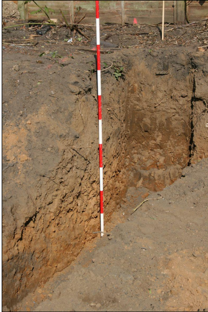
Plate 16: Watching brief: soil profile in footing trench, west corner of new build
