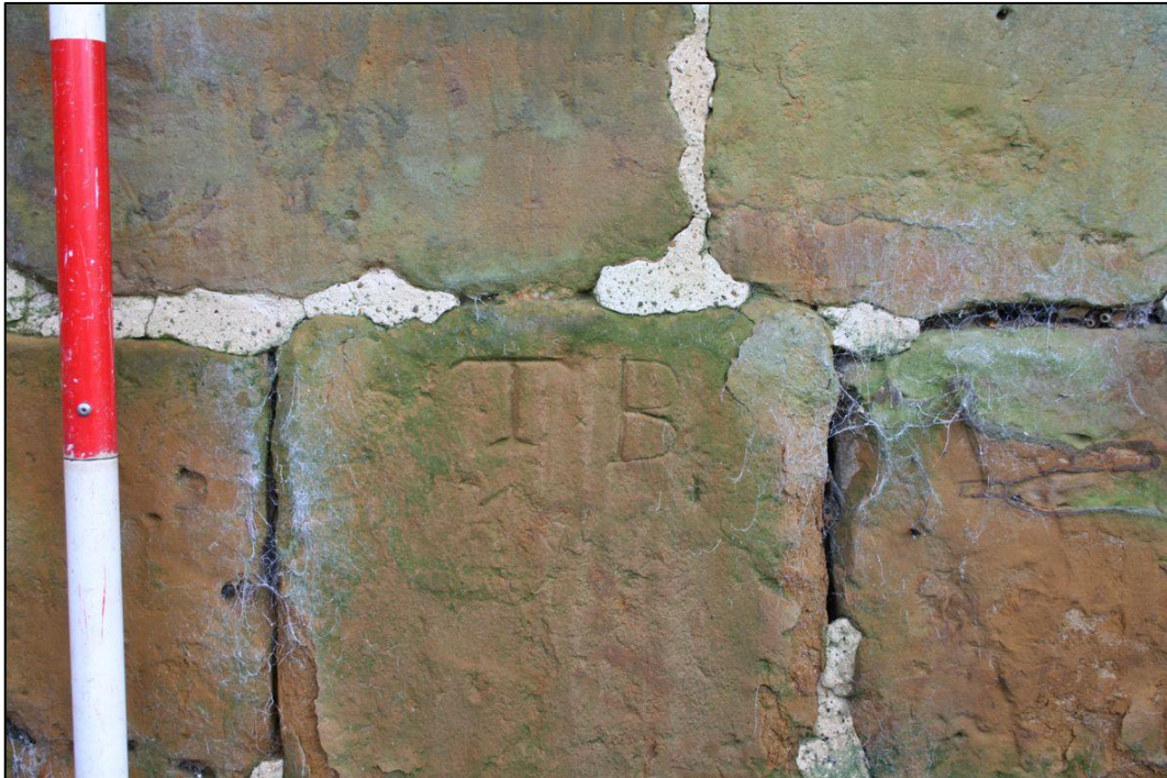
Plate 3: South-west elevation, detail of graffito 'T × B'
