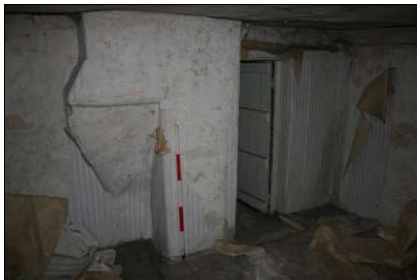
Plate 26: F5, chimney stack by door, looking south-west
