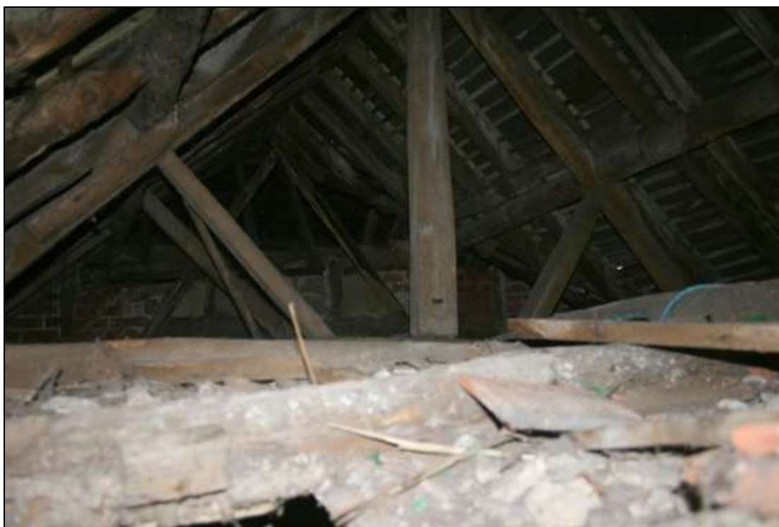
Plate 30: Roof, through ceiling of F5, looking north
