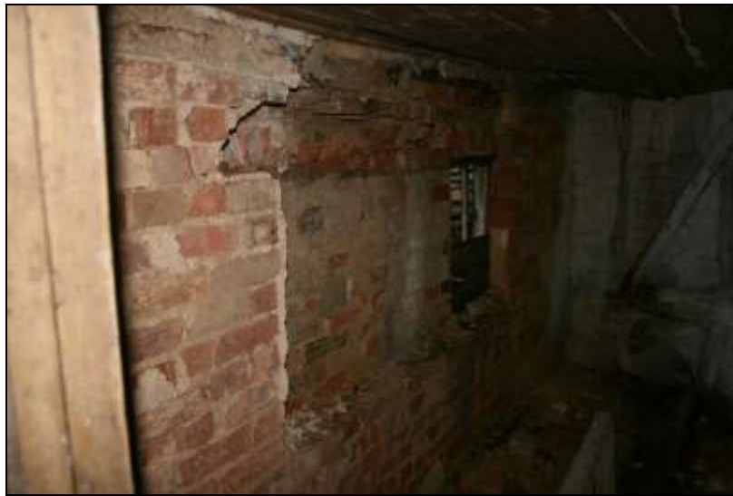
Plate 25: F4, west wall looking north
