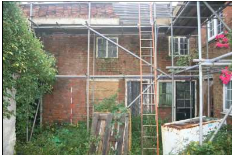
Plate 4: Woodbine Cottage, north end of east elevation
