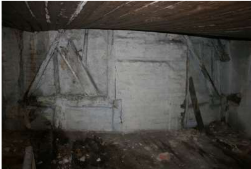
Plate 24: F4, north wall
