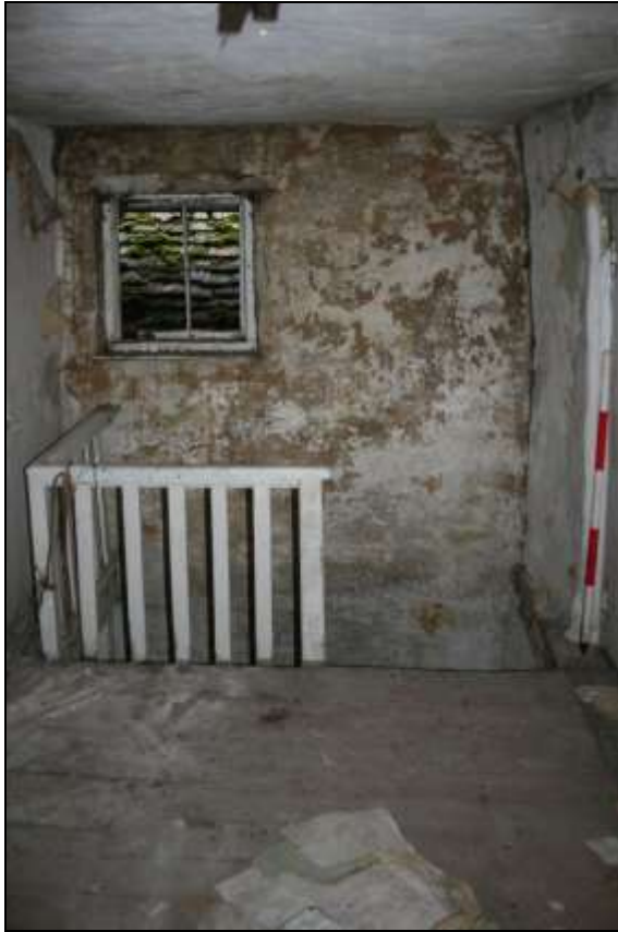
Plate 27: F6, looking west
