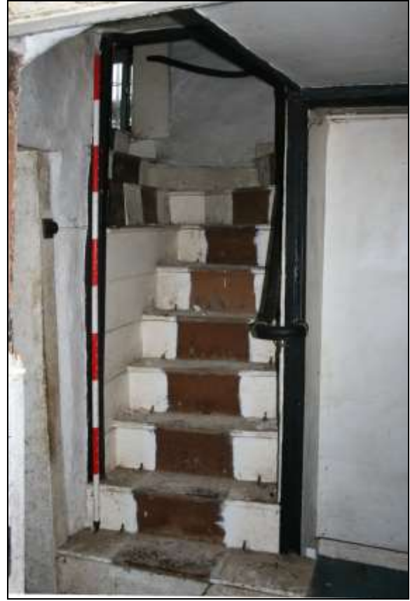
Plate 11: G4, view northward of stairs
