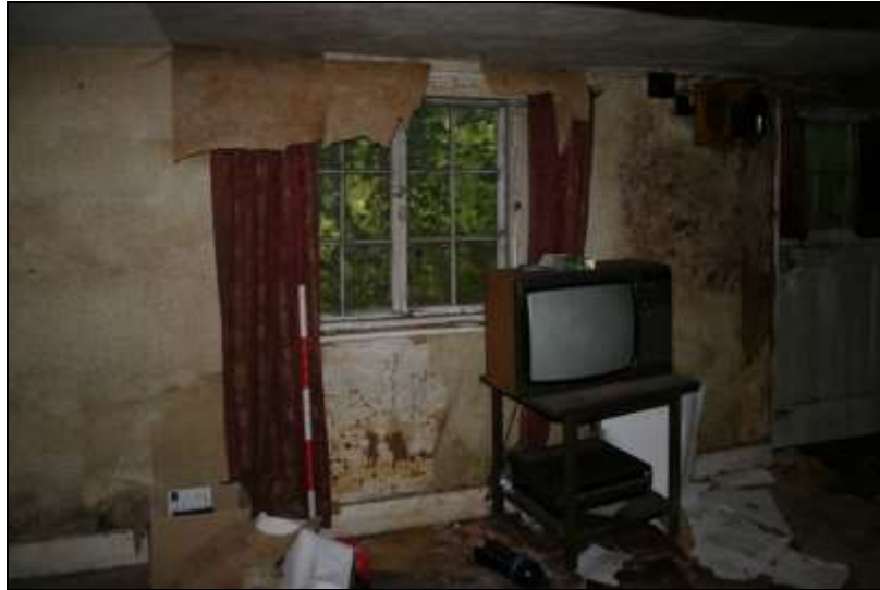
Plate 7: G1, window looking north
