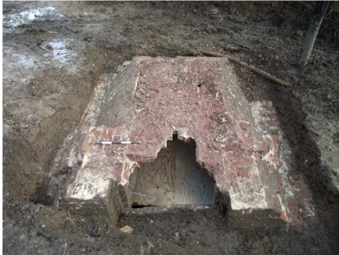
Plate 13: Vault 261: top of vault removal, looking E ( scale 500mm )
