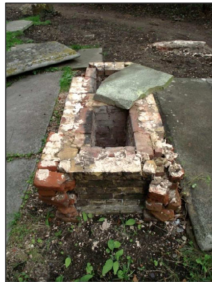
Plate 2: Repair work to monument 193
