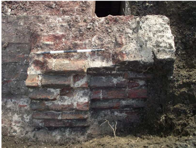
Plate 14: Vault 261: stepped brickwork either side of vault entrance, looking S ( scale 500mm )
