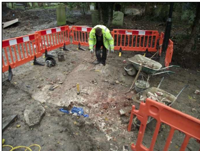
Plate 12: Vault 261: top of vault removal, looking E
