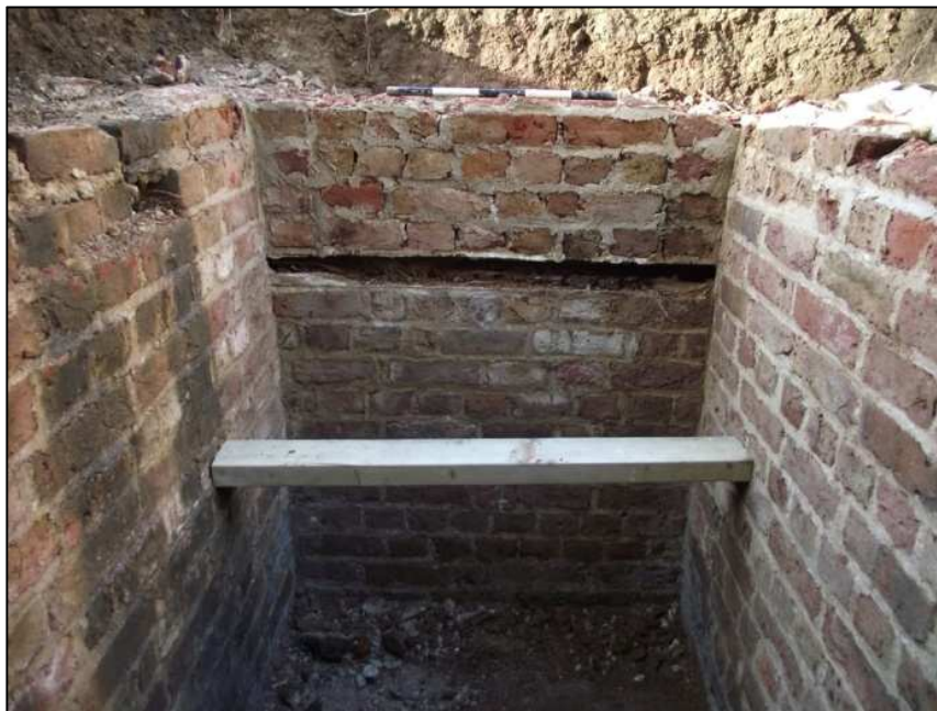
Plate 37: Western wall of vault 262 with opening in brickwork
