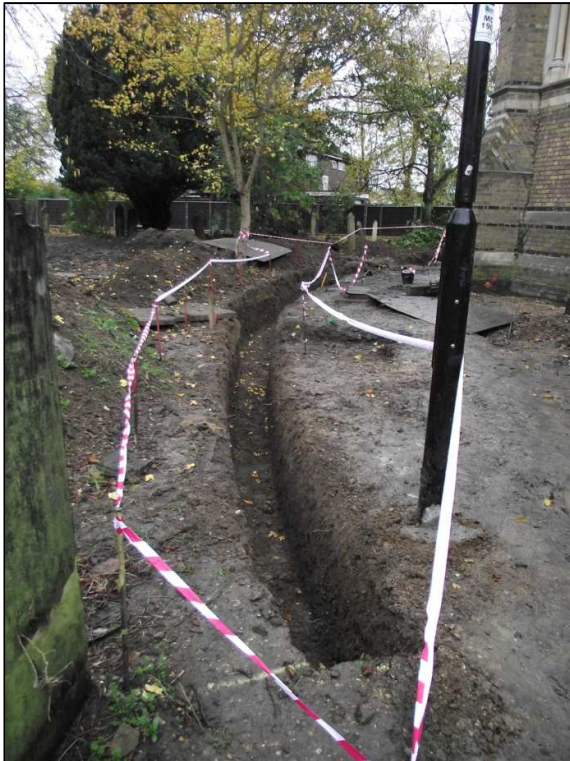
Plate 50: Footing trench for new wall, looking S
