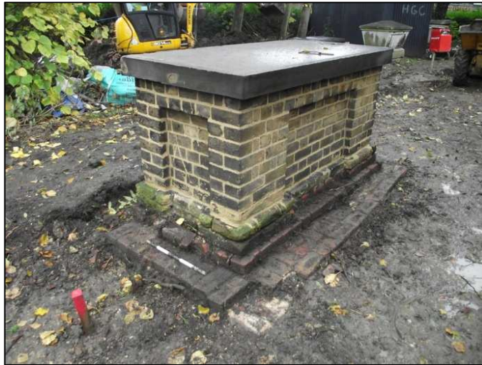
Plate 8: Vault underlying monument 175, looking SW (scale 500mm)
