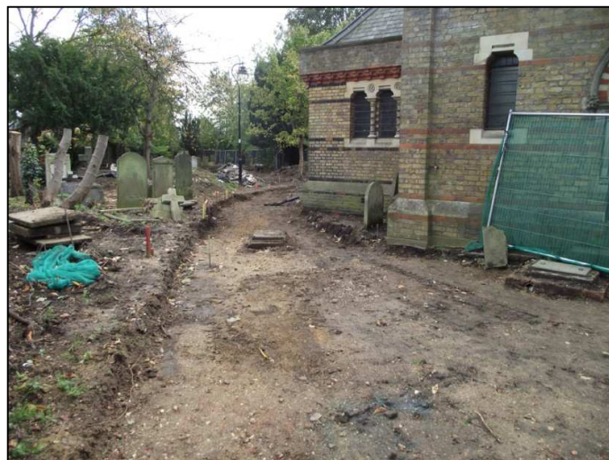
Plate 3: Ground reduction for new pathway, looking SE
