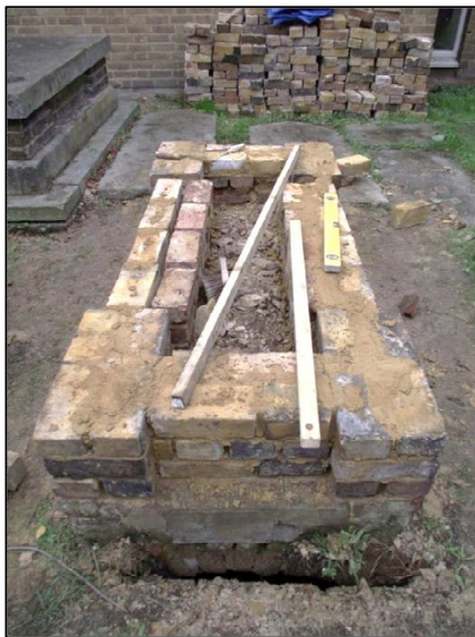
Plate 1: Repair work to monument 183
