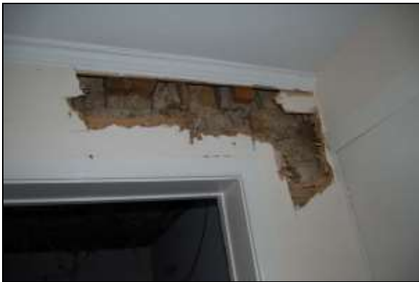
Plate 107: Room F6: partially exposed tiebeam
