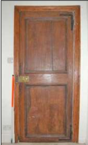
Plate 89: Door between landing and bedroom F5
