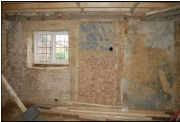
Plate 101: Room G1: north wall during building works
