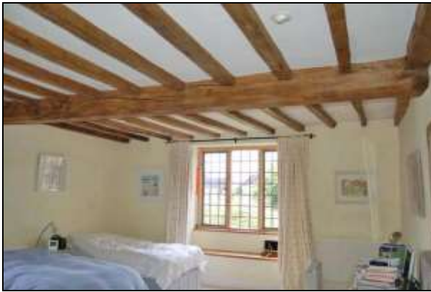
Plate 67: Room F11: south wall
