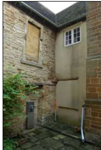
Plate 4: Internal courtyard: southeast corner
