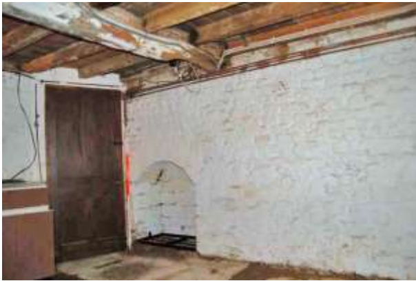
Plate 19: Cellar 2: southeast corner
