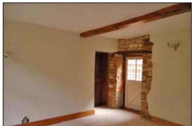
Plate 24: Room G2: northeast corner
