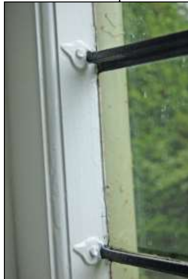
Plate 96: Room F4: window detail
