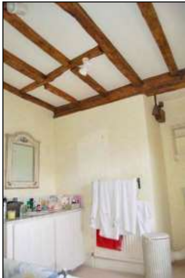
Plate 69: Room F12: looking north
