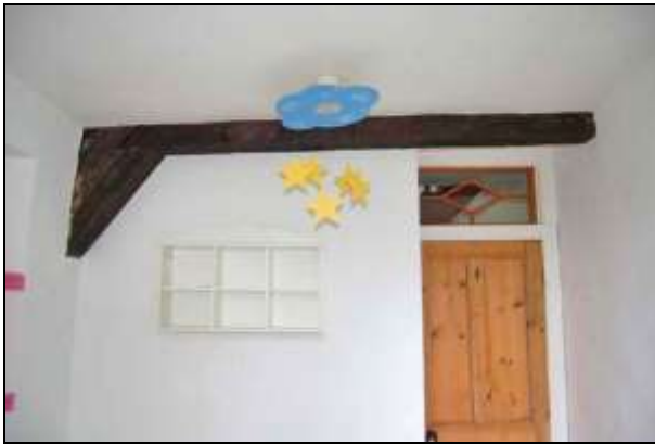
Plate 49: Room F2: east wall
