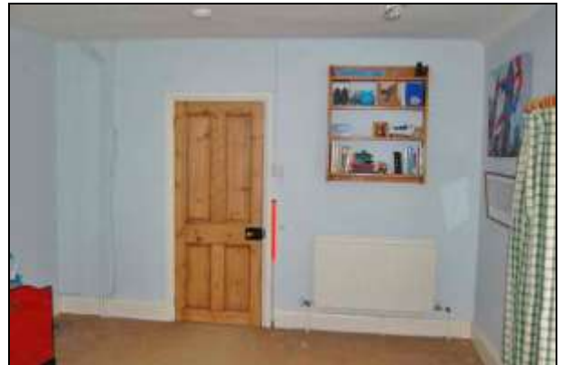
Plate 46: Room F1: west wall
