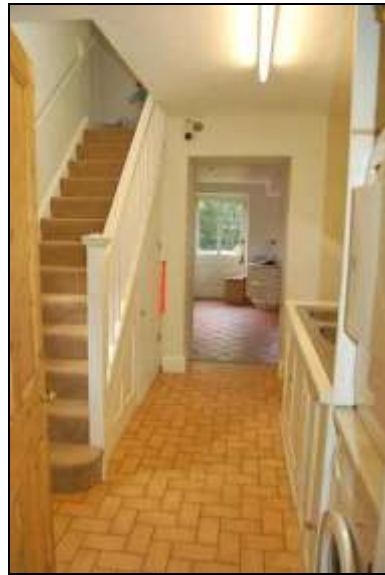
Plate 28: Room G3: looking west
