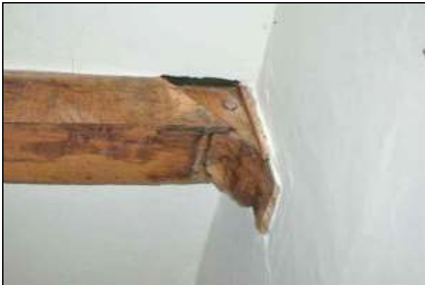
Plate 57: Room F5: timberwork detail
