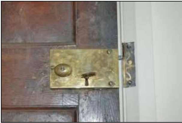
Plate 55: Room F5: door furniture detail
