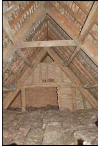
Plate 80: Roofspace east of S4
