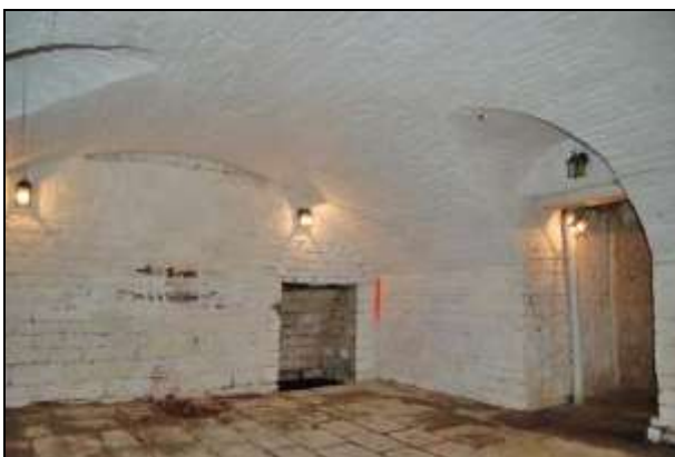
Plate 17: Cellar 1: southeast corner
