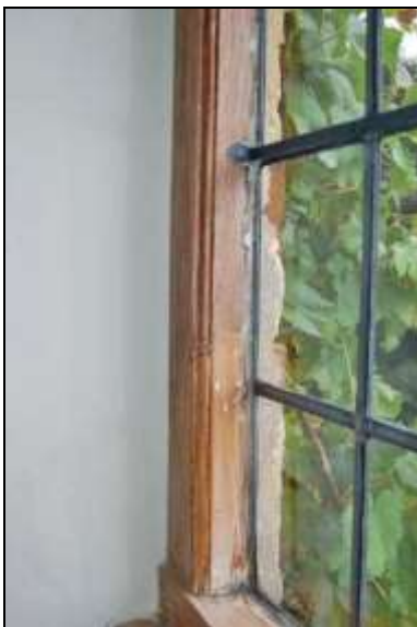
Plate 97: Room F5: window detail
