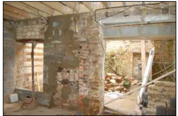
Plate 102: Room G2: extensive modern building fabric revealed in the east wall
