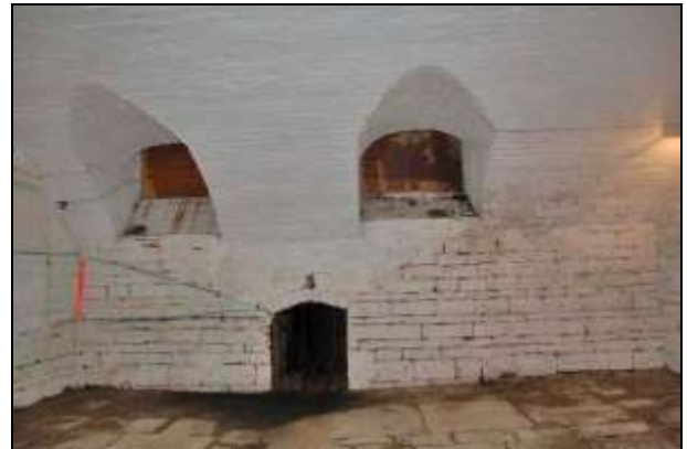
Plate 16: Cellar 1: north wall
