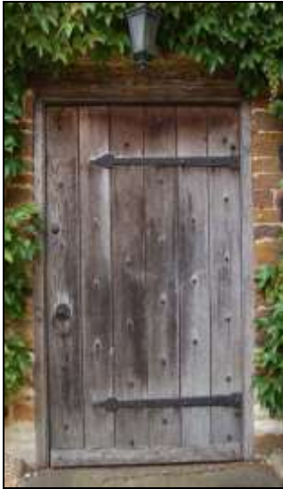
Plate 13: West Range: door detail
