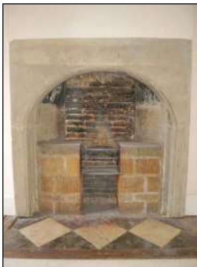
Plate 59: Room F6: fireplace detail
