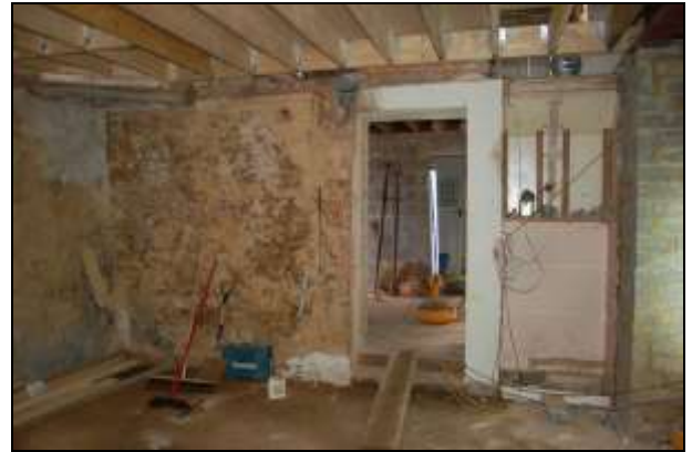
Plate 100: Room G1: east wall during building works
