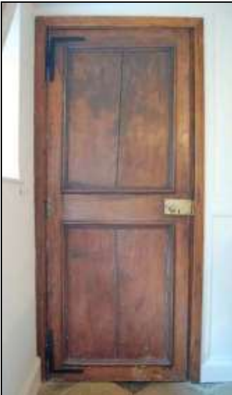
Plate 85: Door below the hall stairs
