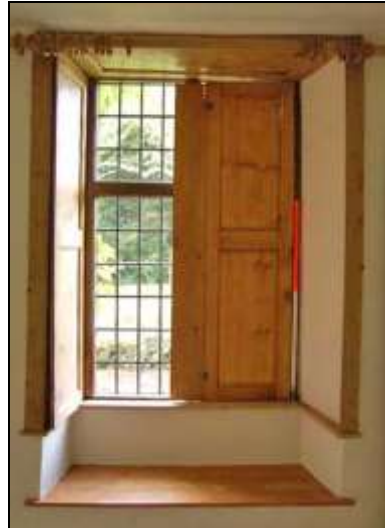
Plate 26: Room G2: window detail
