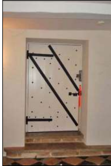
Plate 84: Internal face of front door
