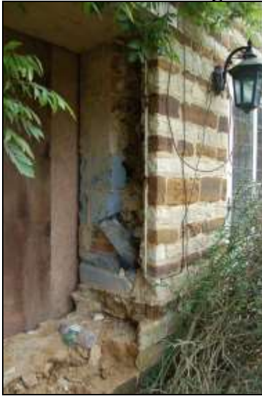
Plate 99: Room G1: window opening in west
