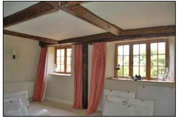
Plate 38: Room G10: southeast corner
