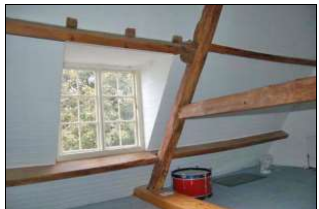
Plate 72: Room S1: north wall
