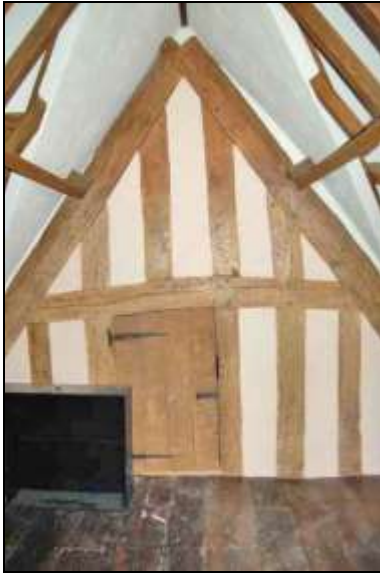
Plate 79: Room S4: eastern gable
