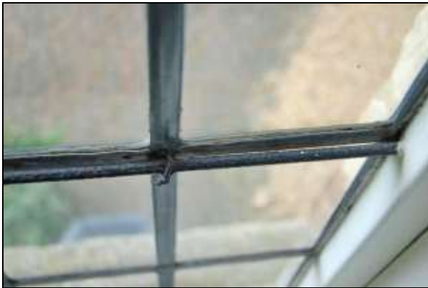
Plate 95: Room F1: window detail
