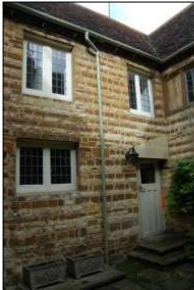
Plate 15: Internal courtyard: north wall
