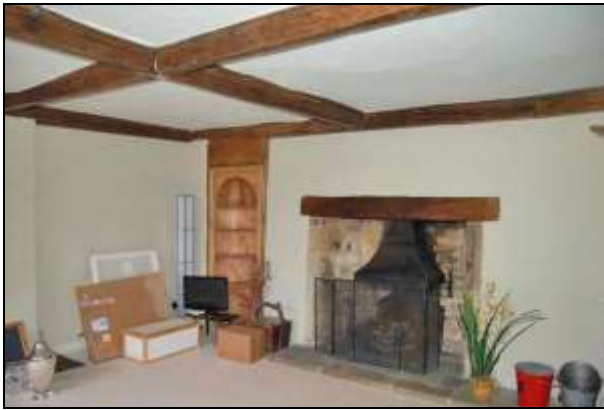
Plate 37: Room G10: northwest corner
