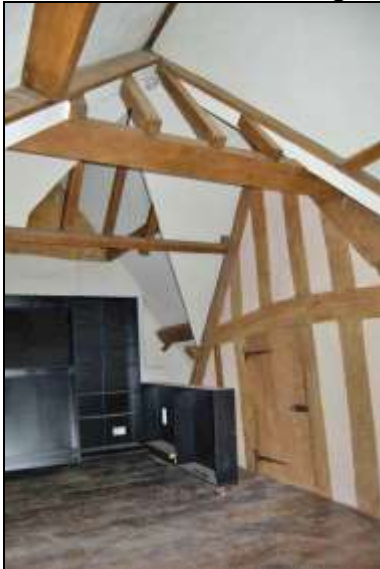
Plate 81: Room S4: looking northeast
