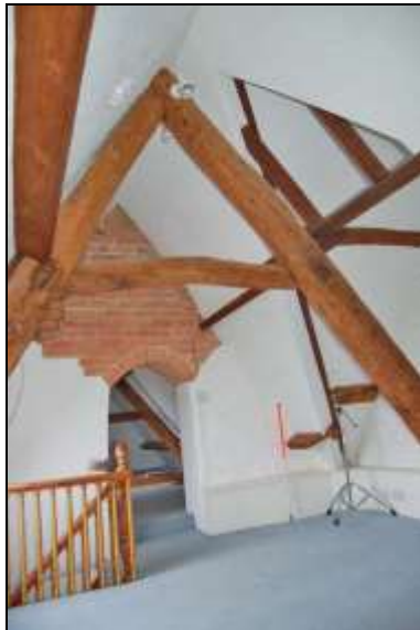
Plate 75: Room S2: east wall
