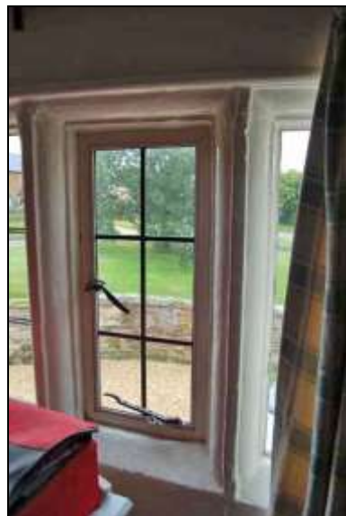
Plate 98: Room F10: window detail
