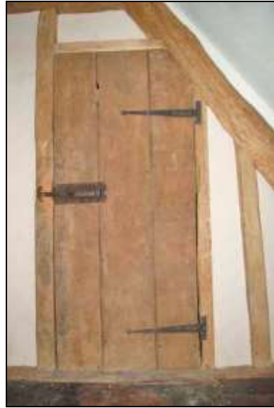
Plate 94: Door to roofspace south of S4
