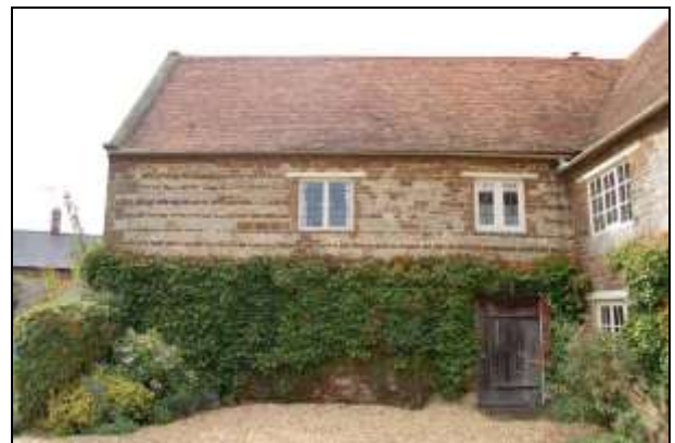
Plate 12: West Range: east elevation
