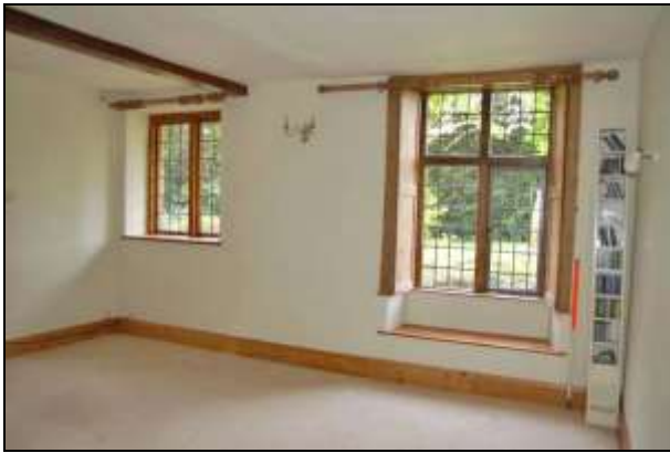
Plate 25: Room G2: west wall
