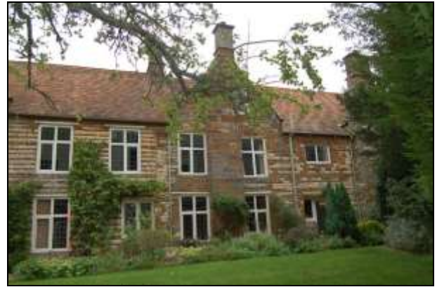
Plate 8: West elevation: central section
