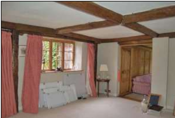
Plate 39: Room G10: southwest corner
