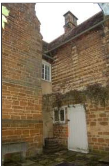
Plate 5: Internal courtyard: southwest corner
