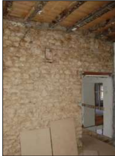
Plate 106: Room F5: bonding and end of ceiling beam in north wall
