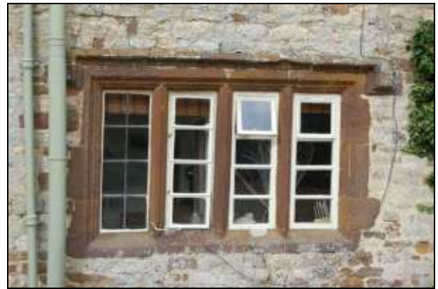
Plate 2: South elevation: stone window
