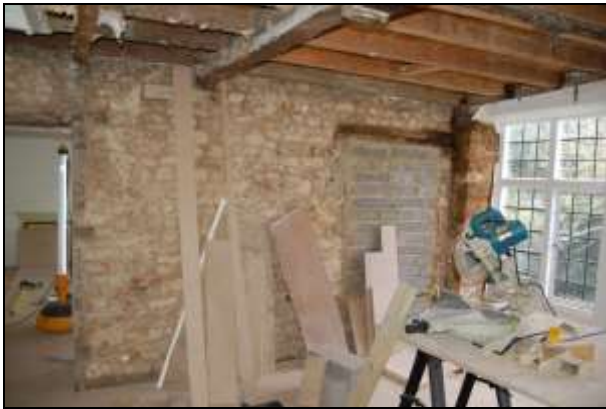
Plate 105: Room F4: blocked door in south wall
