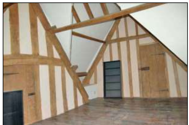
Plate 78: Room S4: looking southeast
