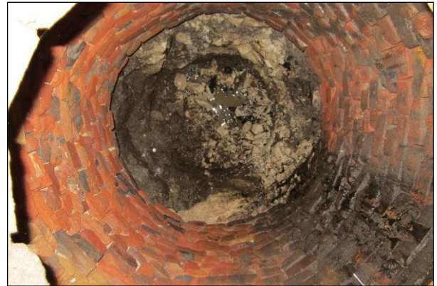
Plate 10: Interior of soakaway showing character of brickwork
