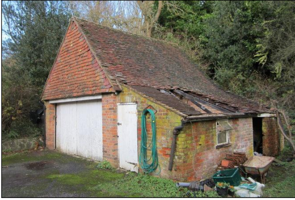
Plate 1: Garage and adjoining outhouse looking north east
