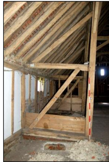
Plate 28: Eastern aisle, Truss 5, looking south
