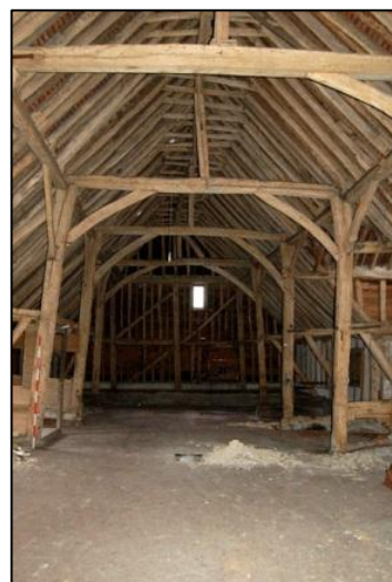
Plate 36: Truss 7, looking south
