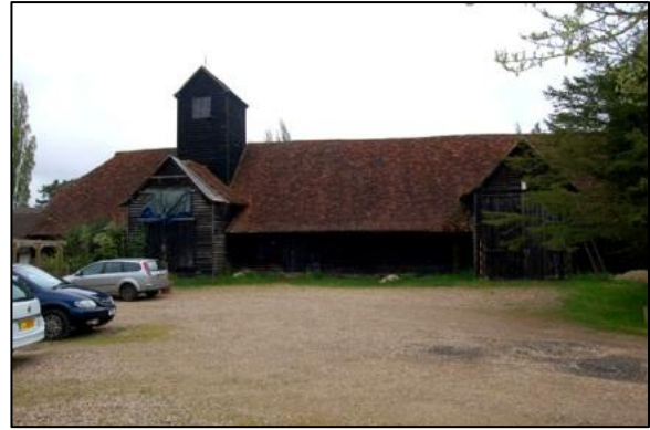
Plate 2: West elevation, looking east
