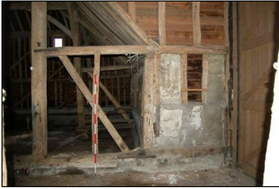
Plate 37: Bay 7, south elevation of south midstrey, looking south
