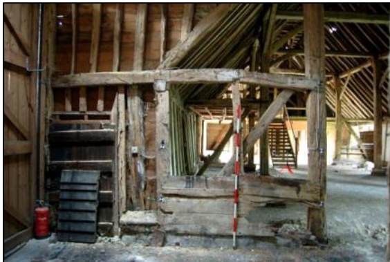
Plate 33: Bay 7, north elevation of south midstrey, looking north
