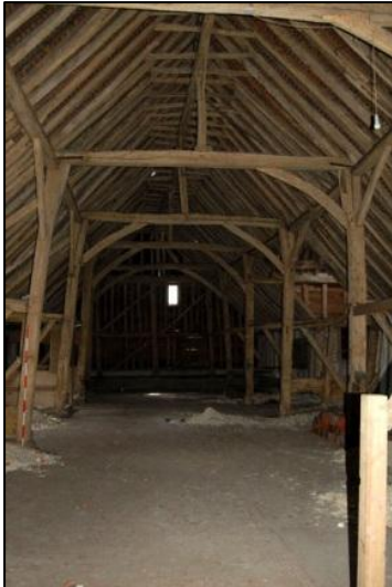
Plate 31: Truss 6, looking south
