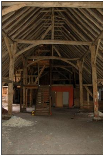
Plate 21: Truss 4, looking north
