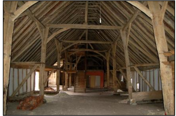
Plate 26: Truss 5, looking north
