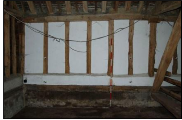
Plate 44: Bay 9, west elevation, looking west
