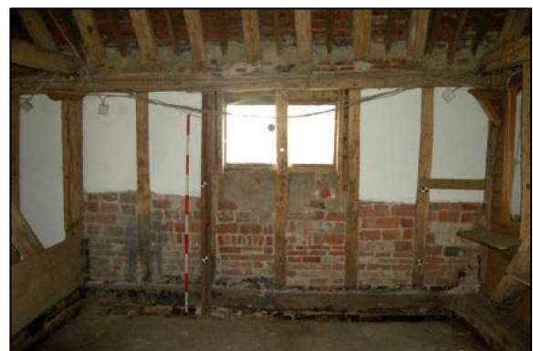
Plate 30: Bay 6, east elevation, looking east
