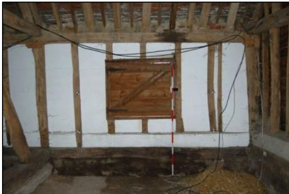
Plate 45: Bay 9, east elevation, looking east
