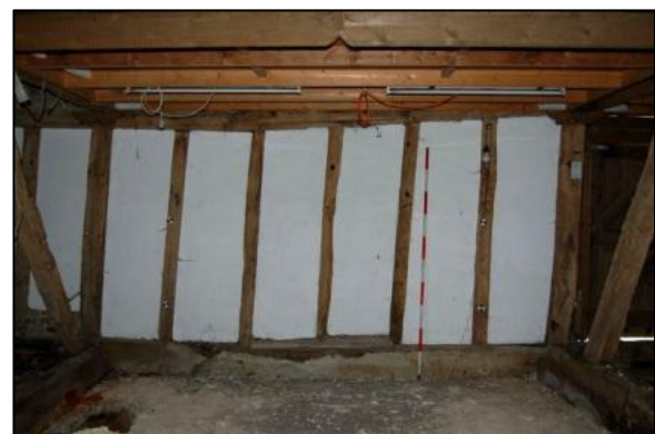
Plate 24: Bay 5, west elevation, looking west
