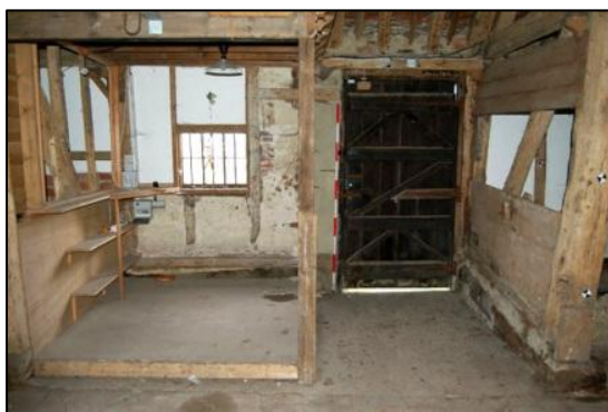
Plate 35: Bay 7, east elevation, looking east
