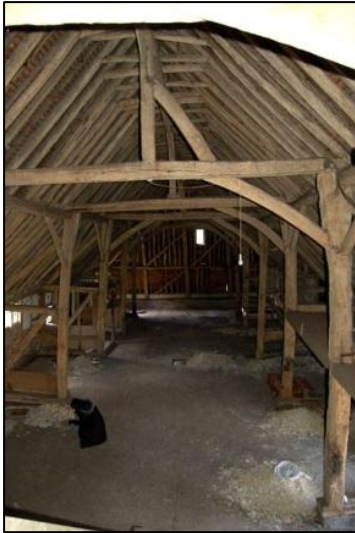
Plate 1: General interior view, looking south from platform
