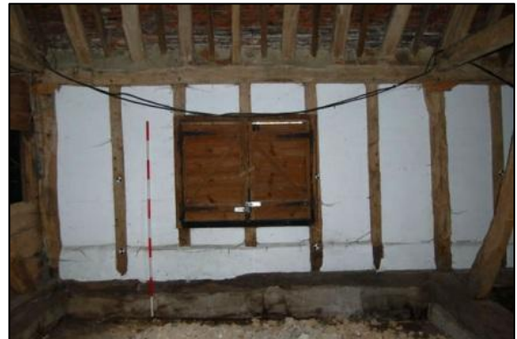
Plate 40: Bay 8, east elevation, looking east
