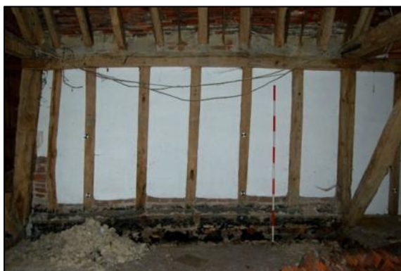
Plate 29: Bay 6, west elevation, looking west
