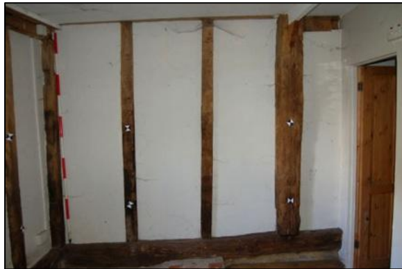
Plate 9: Bay 1, north elevation, looking north
