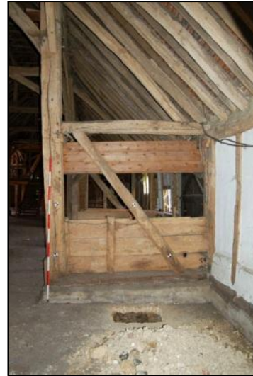
Plate 38: Eastern aisle, Truss 7, looking north
