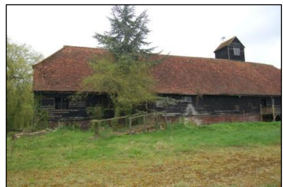
Plate 6: South end of east elevation, looking north west
