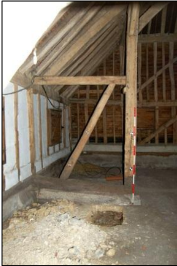
Plate 43: Eastern aisle, Truss 8, looking south
