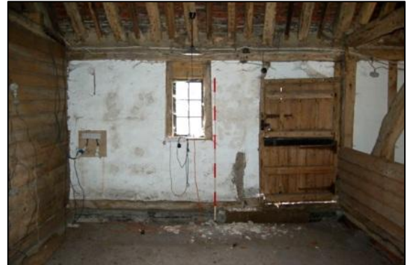
Plate 16: Bay 3, east elevation, looking east
