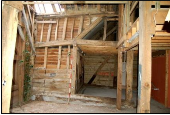
Plate 13: Bay 3, north elevation of midstrey, looking north
