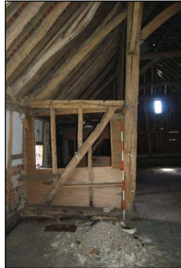
Plate 32: Eastern aisle, Truss 6, looking south
