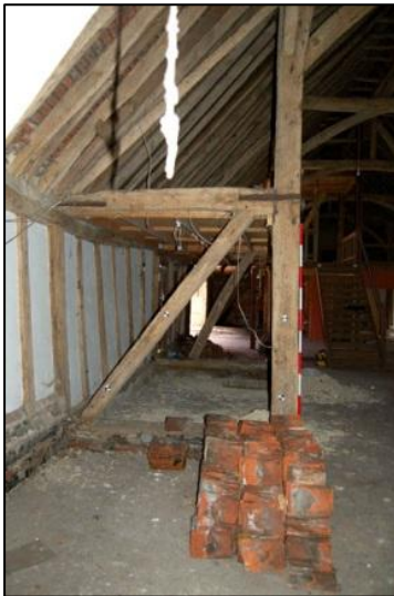
Plate 27: Western aisle, Truss 5, looking north
