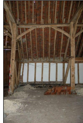
Plate 50: Bay 6, showing face halved scarf joint in purlin, looking west
