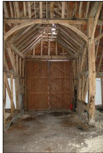
Plate 34: Bay 7, midstrey, looking west
