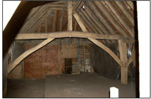
Plate 8: Truss 2, looking north
