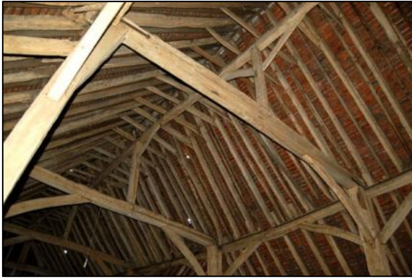
Plate 7: Roof detail of Trusses 4 and 5, looking southwest
