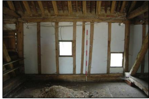
Plate 20: Bay 4, east elevation, looking east
