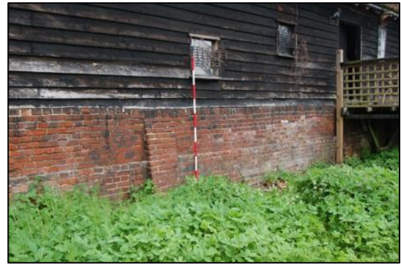
Plate 4: East elevation: detail of brick buttress, looking north west
