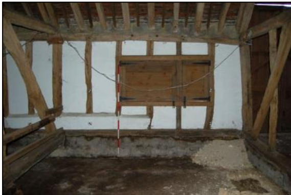
Plate 39: Bay 8, west elevation, looking west
