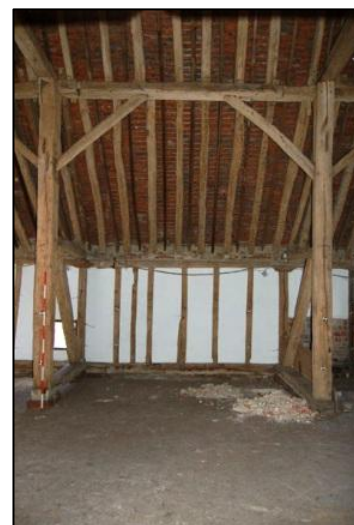
Plate 48: Bay 5, showing face halved scarf joints in purlin, looking east
