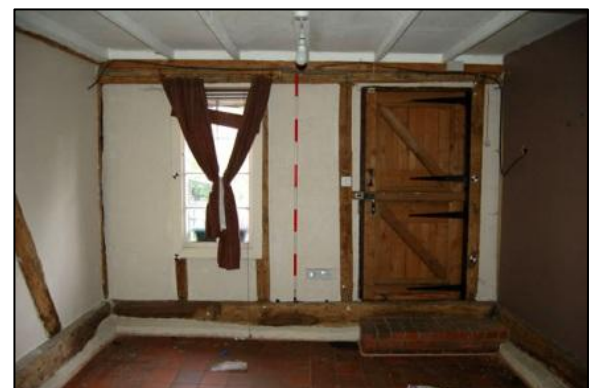
Plate 12: Bay 2, east elevation, looking east
