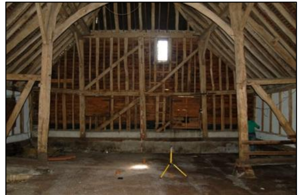
Plate 46: Southern gable end, looking south
