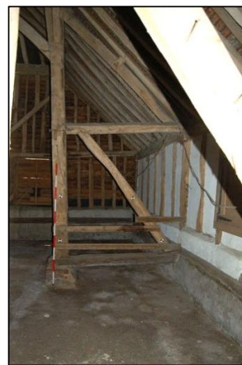
Plate 42: Western aisle, Truss 8, looking south
