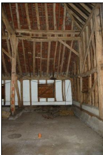
Plate 47: View of extra purlin above Bay 9, looking east
