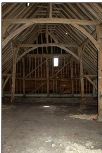
Plate 41: Truss 8, looking south
