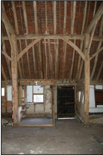
Plate 49: Bay 7, showing face halved scarf joint in purlin, looking east
