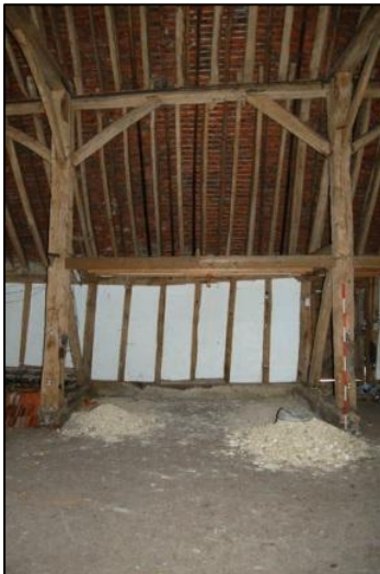
Plate 51: Bay 5, showing face halved scarf joint in purlin, looking west
