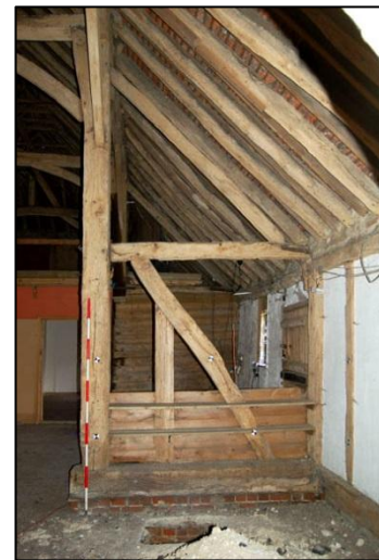
Plate 18: Eastern aisle, Truss 3, looking north
