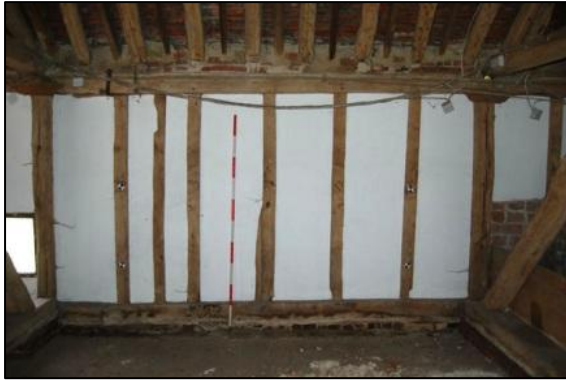
Plate 25: Bay 5, east elevation, looking east
