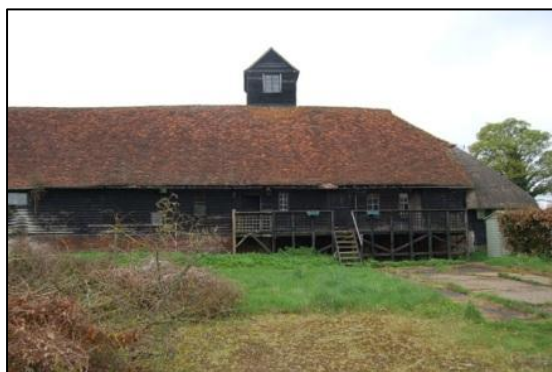
Plate 5: North end of east elevation, looking west
