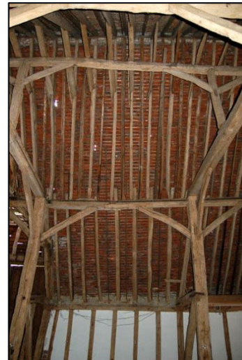
Plate 52: Bay 6, roof construction, looking west
