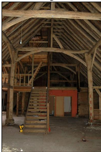
Plate 17: Truss 3, looking north
