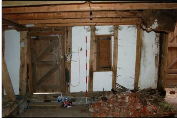
Plate 19: Bay 4, west elevation, looking west
