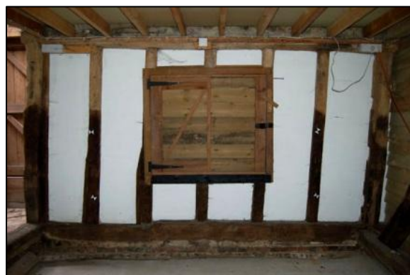
Plate 11: Bay 2, west elevation, looking west
