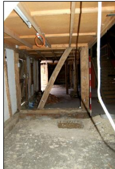
Plate 22: Western aisle, Truss 4, looking north
