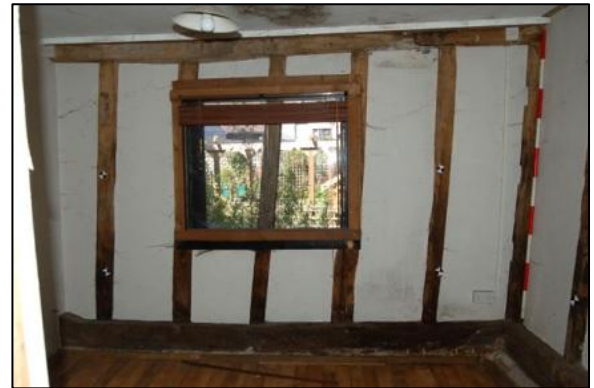
Plate 10: Bay 1, west elevation, looking west
