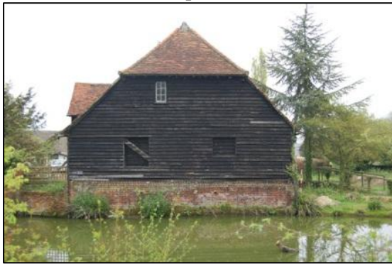
Plate 3: South elevation, looking north
