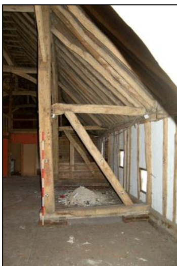
Plate 23: Eastern aisle, Truss 4, looking north
