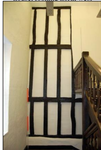
Plate 10: Close studding on north east external wall of crosswing, looking south
