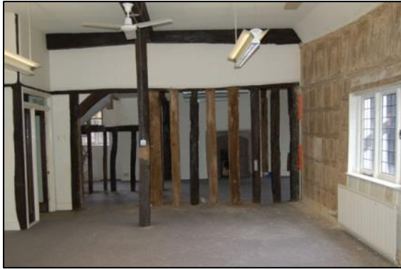
Plate 13: Exposed timbers in northern part of Studio 1, looking south
