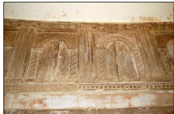
Plate 12: Detail of stripped panelling in Studio 1
