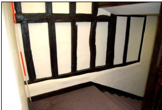
Plate 9: Close studding on north east external wall of crosswing, looking south
