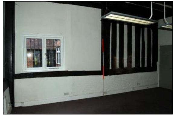
Plate 2: Conference Room, looking north east
