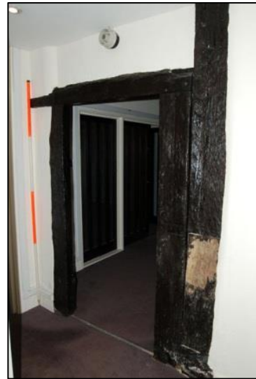
Plate 8: Door between cross-wing and main house, looking north west
