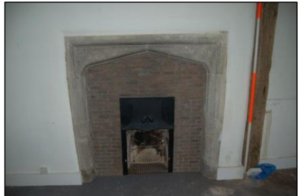
Plate 16: Fireplace with stone surround and Brocket Arms in south wall of Studio 1
