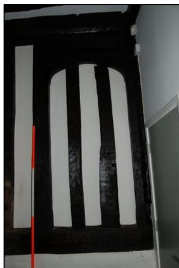
Plate 5: Detail of inserted doorframe, north wall of Conference Room
