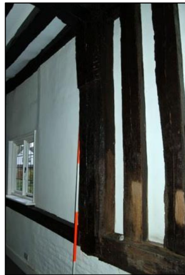
Plate 4: Detail of principal post, north wall of Conference Room
