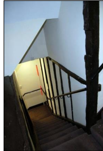
Plate 20: Close studding on stairs to second floor, looking east
