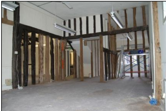
Plate 15: Exposed timbers in western part of Studio 1, looking north east
