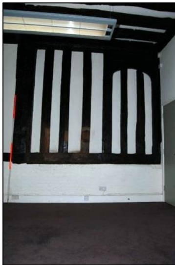
Plate 3: Close studding and inserted doorframe in north wall of Conference Room
