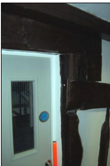
Plate 29: Timbers surrounding inserted door from cross-wing to Office 5, looking north east
