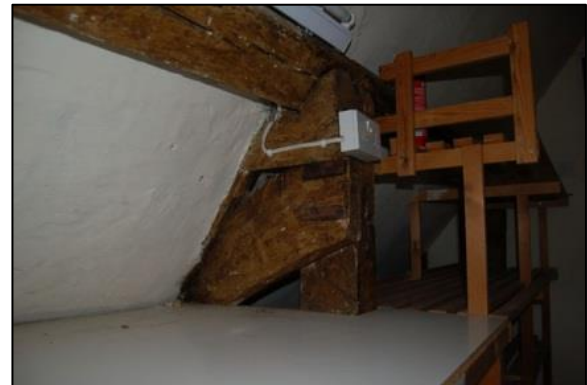
Plate 28: Cut clasped purlin, north side of Archive Store, looking east
