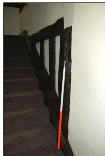
Plate 30: Close studding on northern wall of cross-wing, second floor, looking north east
