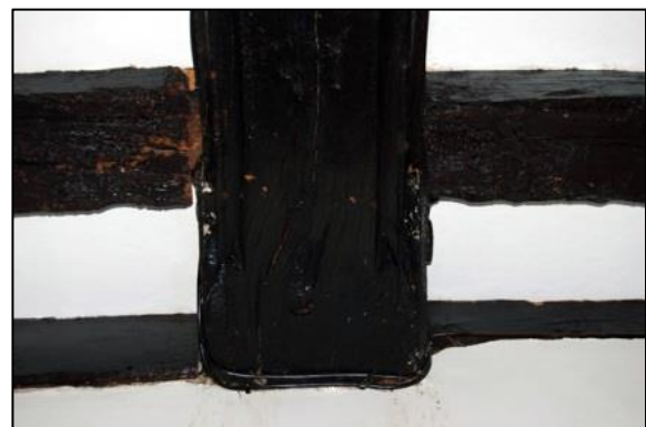
Plate 6: Detail of bridging beam in Conference Room, with pyramid chamfer stop
