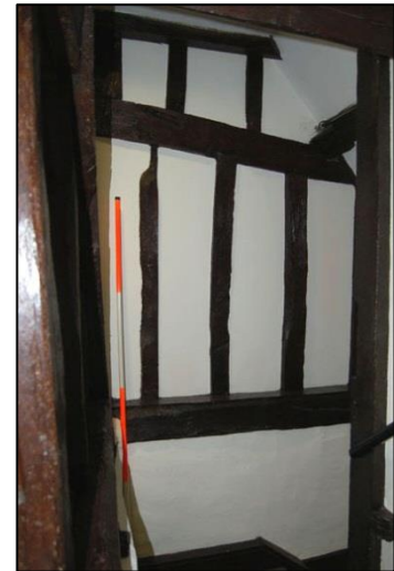
Plate 22: Close studding on northern wall of stairwell, second floor, looking north
