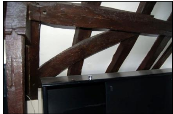
Plate 26: Wind brace, south side of Office 4, looking south
