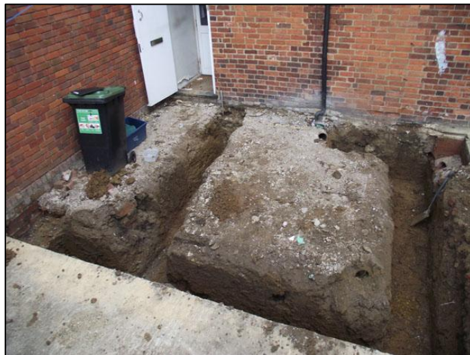
Plate 3: General footing shot, looking north
