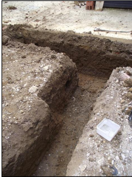
Plate 1: Footing trench with modern intrusion, looking south
