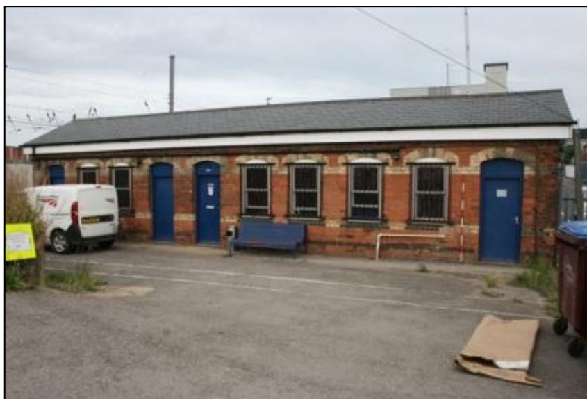
Plate 21: Building 3, east elevation looking west
