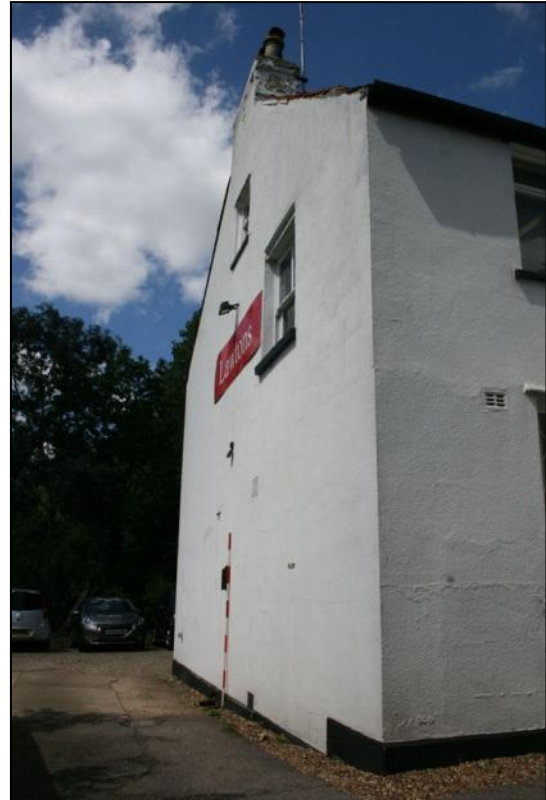
Plate 6: Station House, south elevation of main building, looking north-west
