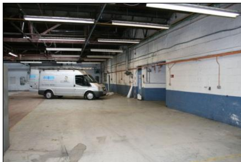
Plate 36: Cougar Garage, central bays, looking south-east
