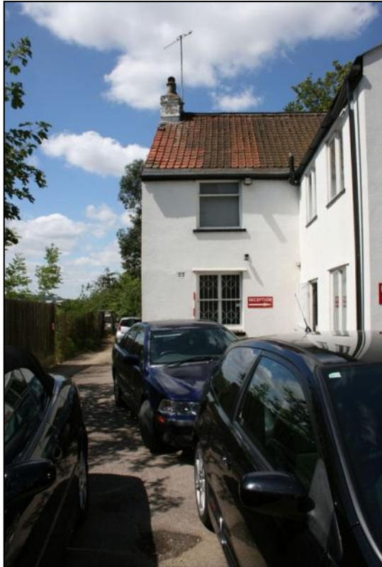
Plate 5: Station House, east elevation of main building, looking west
