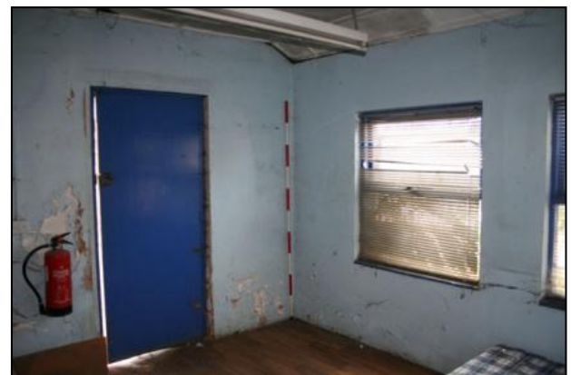
Plate 20: Building 2, interior, looking south east
