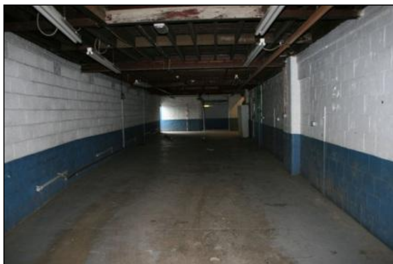
Plate 39: Cougar Garage rear extension, looking north-west
