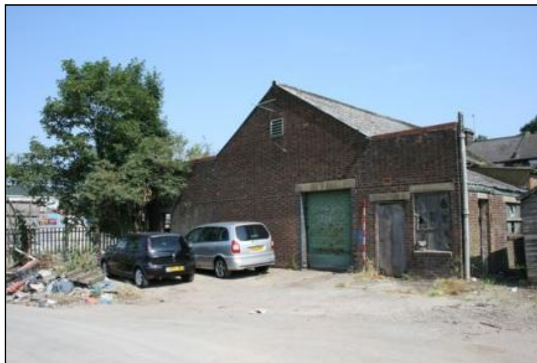
Plate 9: Building 1, south elevation looking north-west
