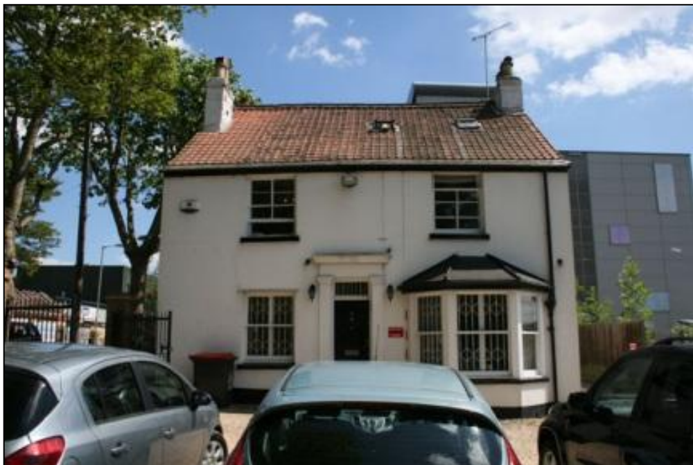
Plate 1: Station House, west elevation looking east
