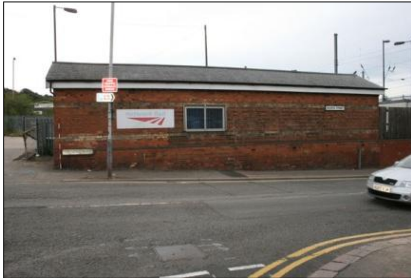
Plate 23: Building 3, west elevation looking east
