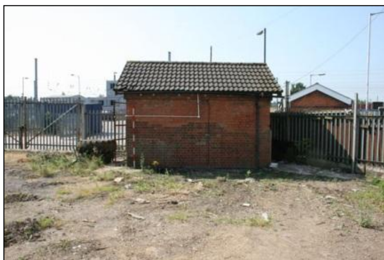
Plate 16: Building 2, north elevation looking south
