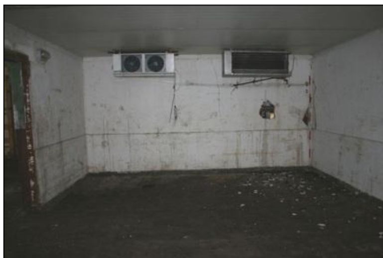
Plate 14: Building 1, cold store looking south
