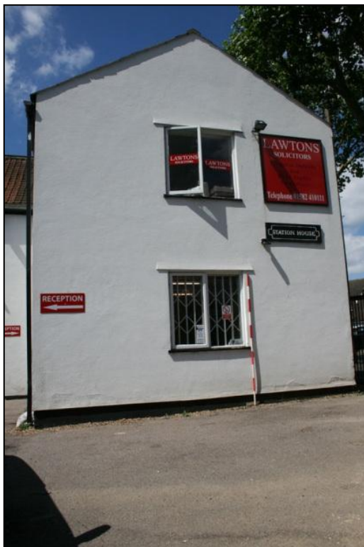
Plate 3: Station House, east elevation of extension, looking west
