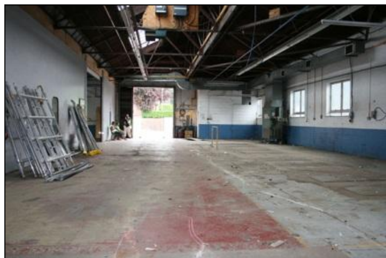
Plate 33: Cougar Garage, easternmost bay, looking north-east
