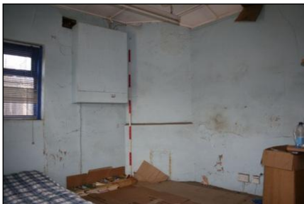
Plate 19: Building 2, interior, looking north west
