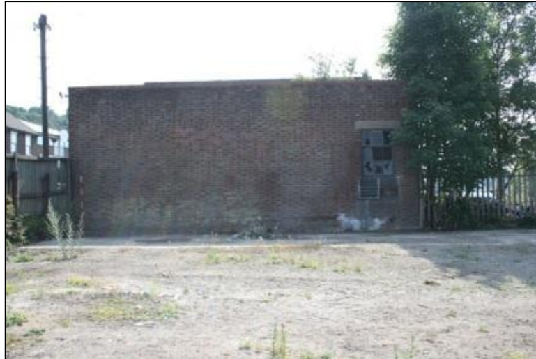
Plate 8: Building 1, west elevation looking east
