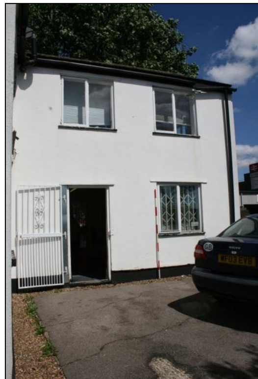
Plate 4: Station House, south elevation of extension, looking north
