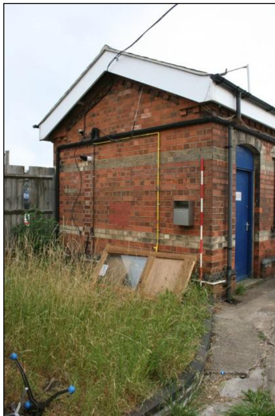
Plate 24: Building 3, south elevation looking north-west
