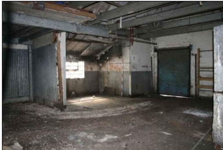
Plate 12: Building 1, interior looking south
