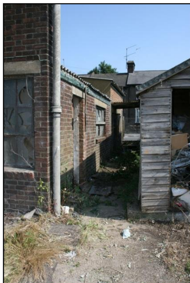
Plate 10: Building 1, east elevation looking north
