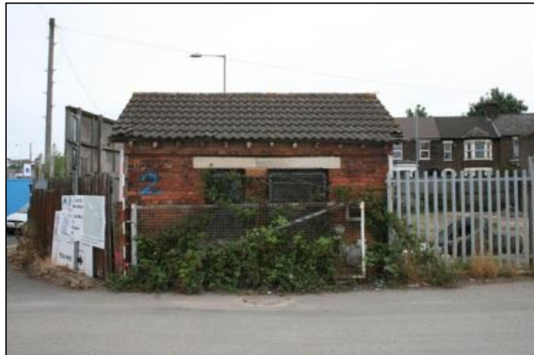
Plate 18: Building 2, south elevation looking north
