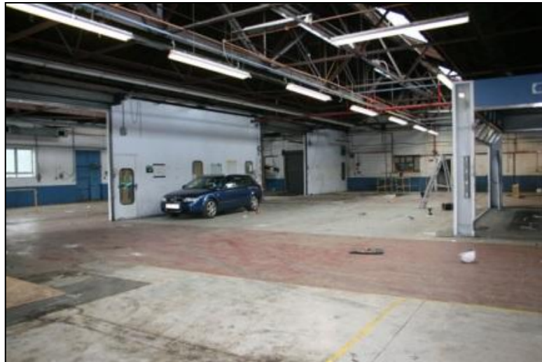
Plate 35: Cougar Garage, central bays, looking south
