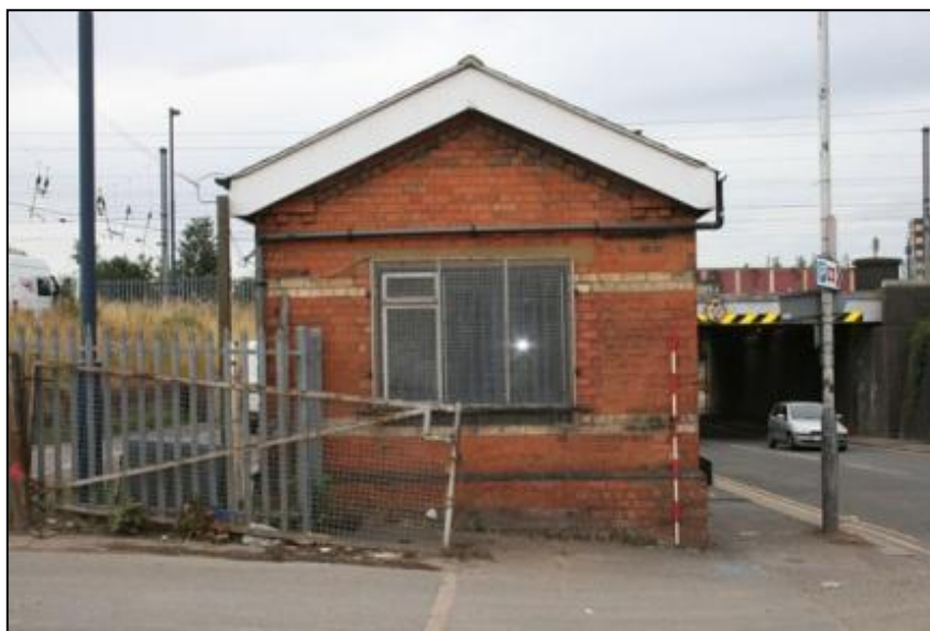
Plate 22: Building 3, north elevation looking south
