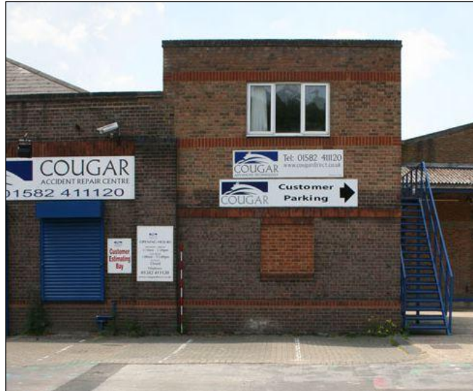
Plate 28: Cougar Garage, north-east frontage, detail of office block at north-west corner
