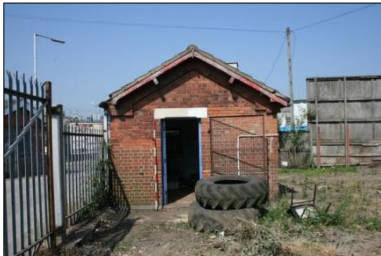
Plate 15: Building 2, east elevation looking west
