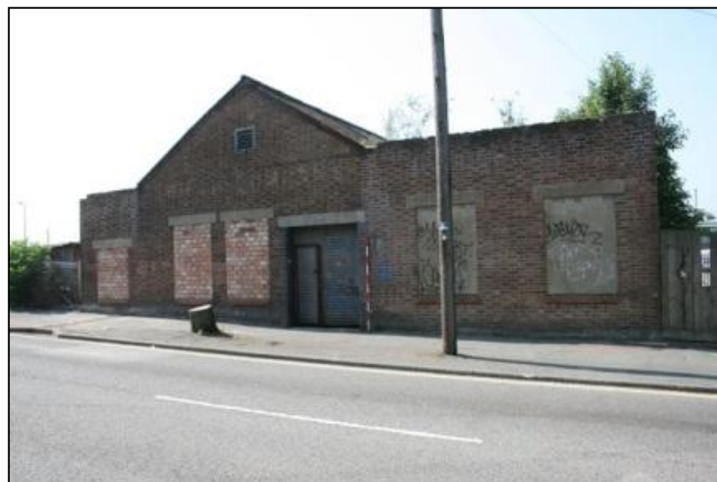
Plate 7: Building 1, north elevation looking south east
