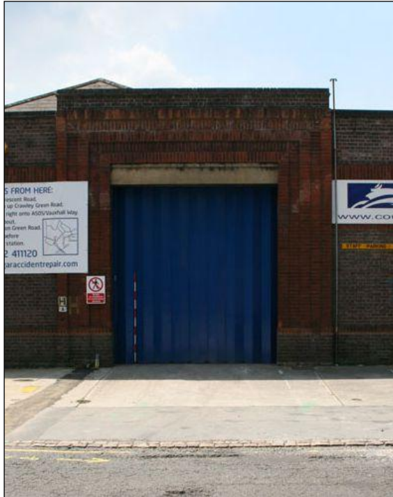
Plate 25: Cougar Garage, north-east frontage, detail of vehicle access
