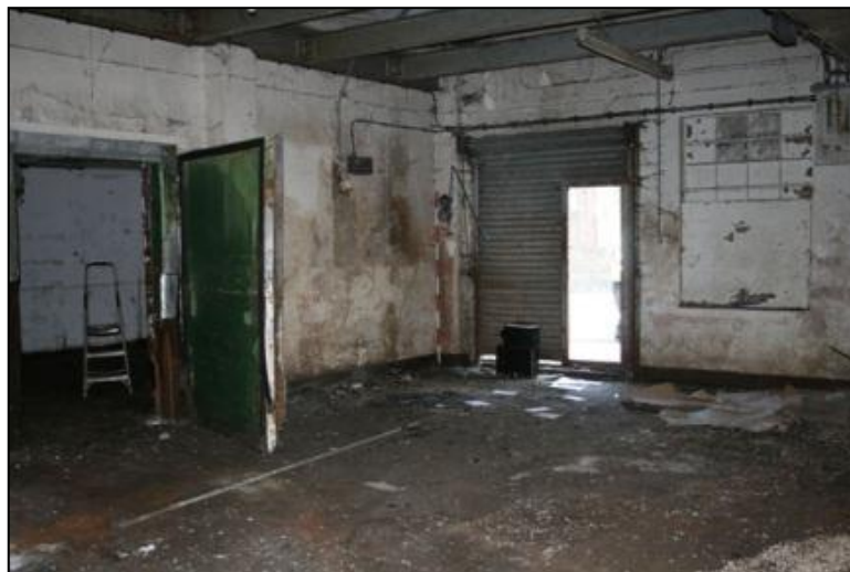
Plate 13: Building 1, interior looking north
