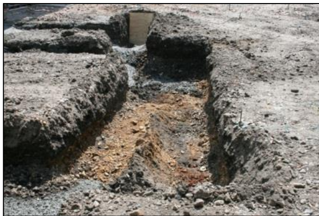
Plate 10: Footing trench in the northwest part of the site, looking south
