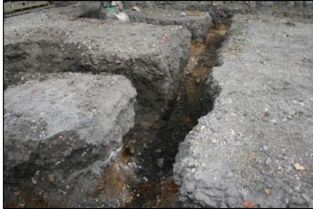
Plate 9: View of footing trenches in the vicinity of Trench 1, looking north
