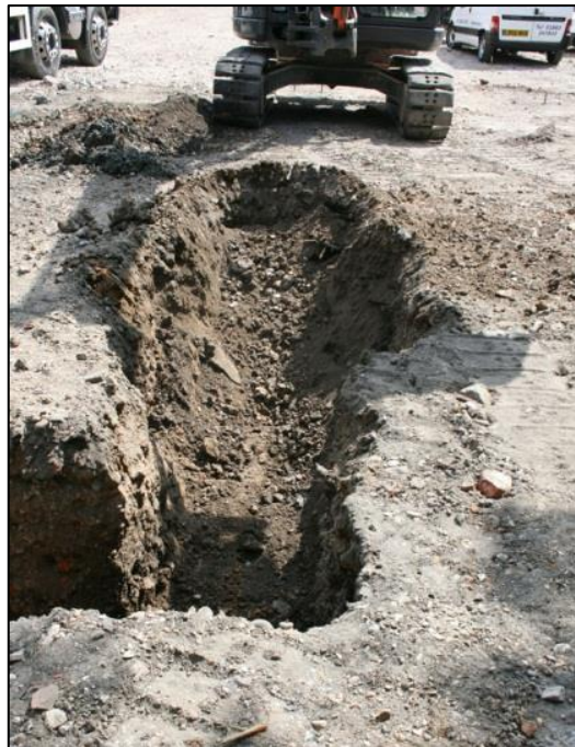
Plate 11: Westernmost footing trench, looking south
