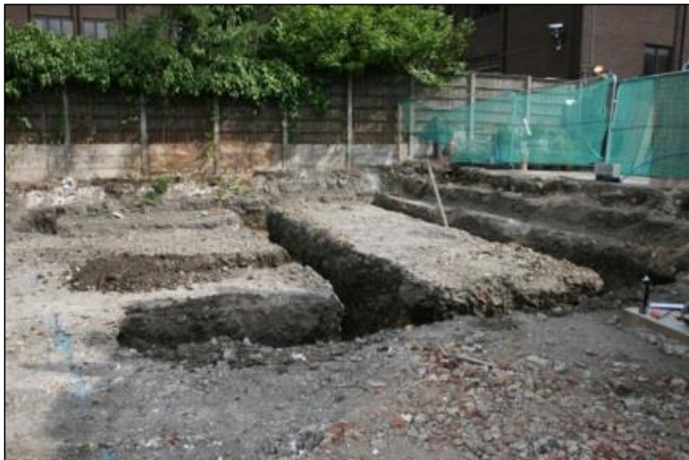
Plate 8: General view of the footing trenches, looking northeast
