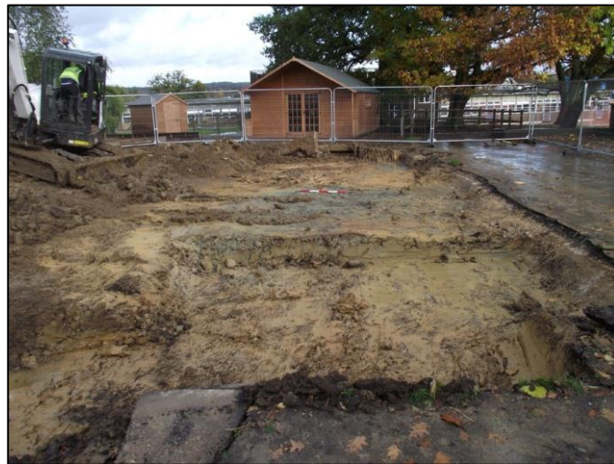
Plate 4: Ground reduction for infant school extension looking NE ( scale 1m )
