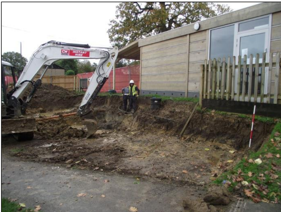
Plate 2: Ground reduction for nursery hub building extension, looking SE ( scale 1m )
