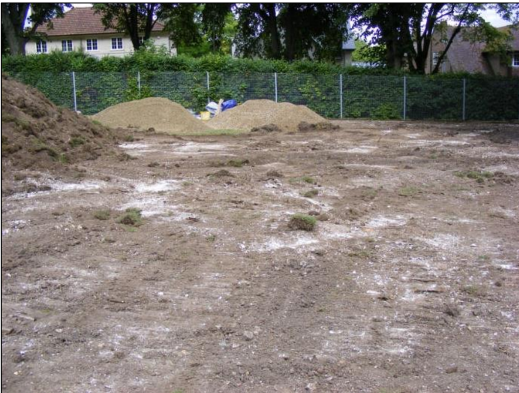
Plate 2: East half of WB2, facing east
