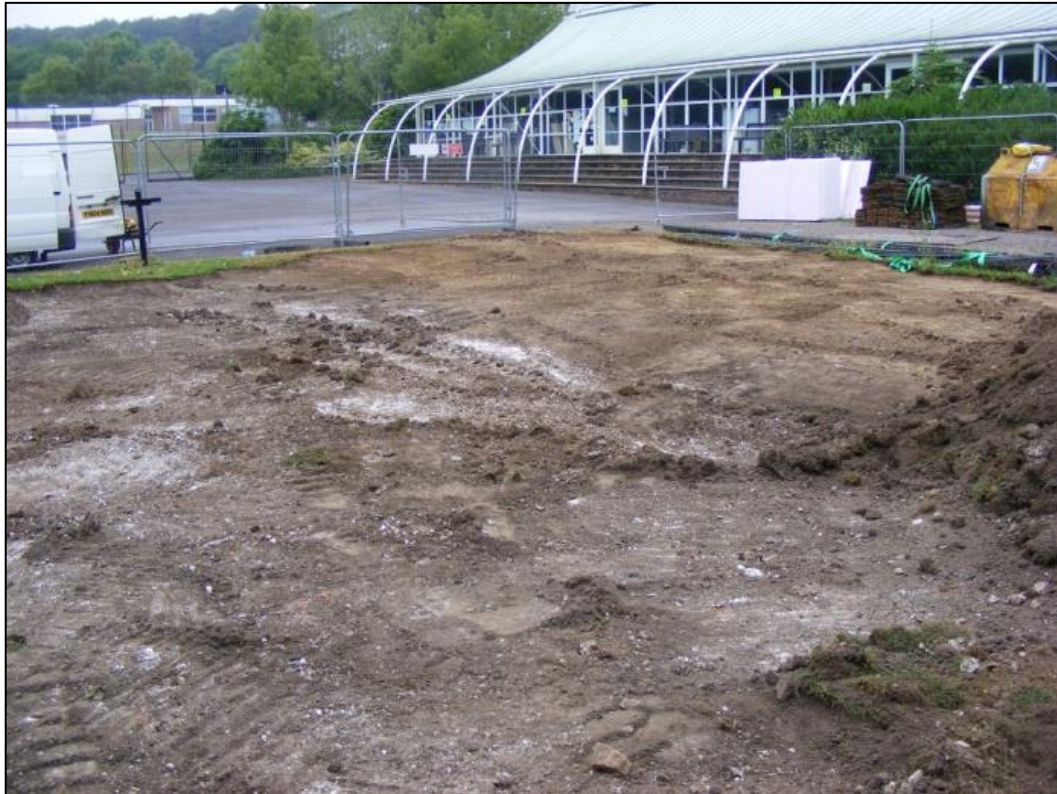
Plate 3: West end of WB2 showing made-ground layers, facing west
