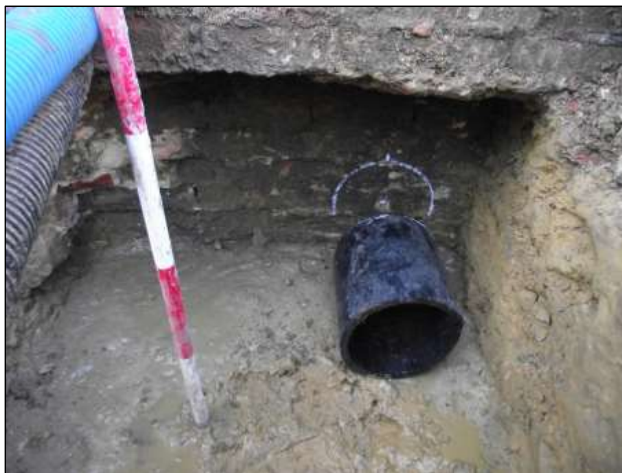
Plate 13: Cellar wall prior to drilling, looking S ( scale 800mm )
