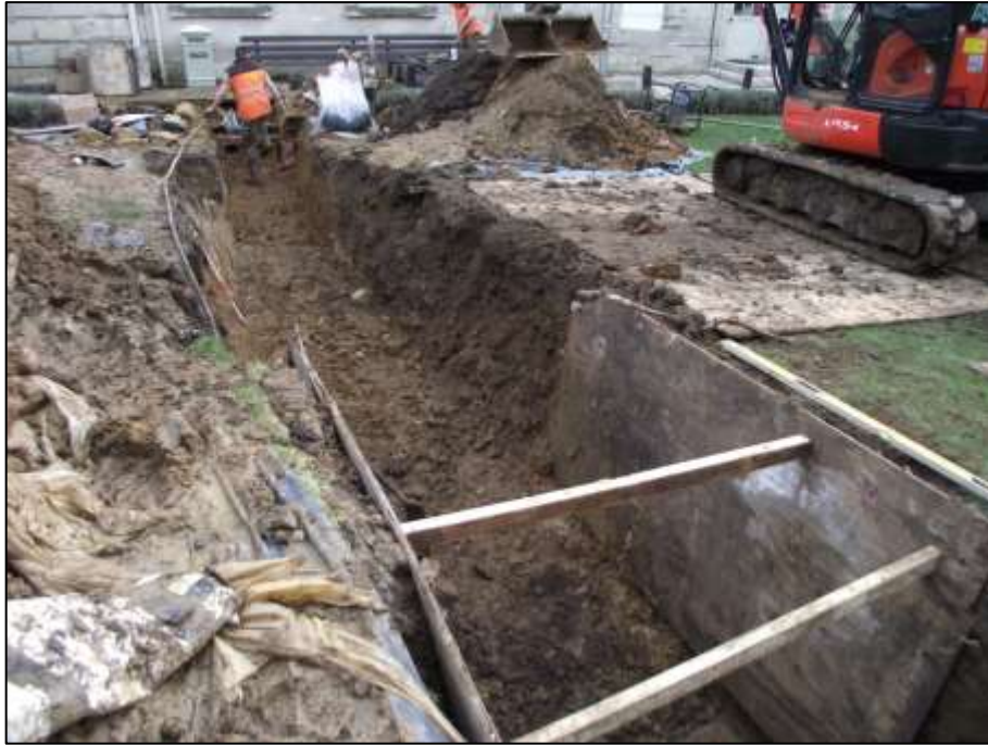
Plate 3: West face of trench, looking SE
