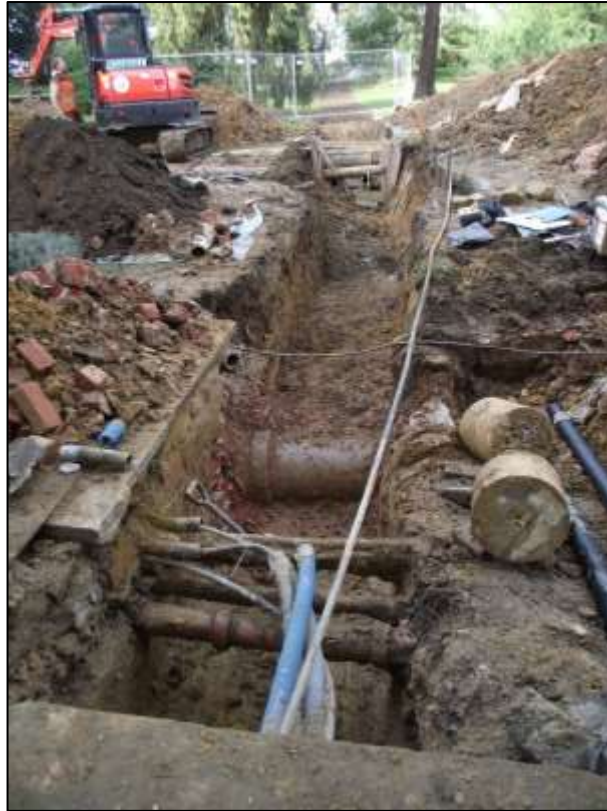
Plate 1: General shot of trench, looking N
