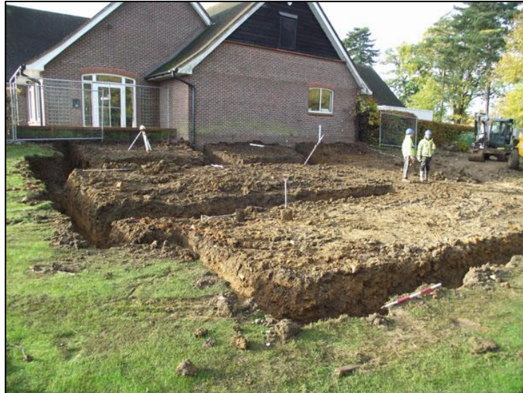
Plate 1: Foundation trenches looking southwest
