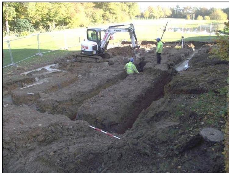
Plate 2: Foundation trenches looking northeast
