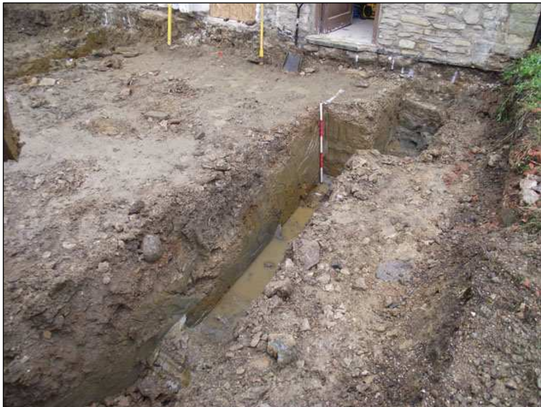
Plate 2: Northern arm of footing trench, looking southwest
