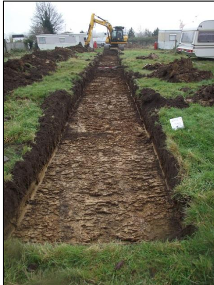
Plate 1: Trench 12, looking north west, 1m scale
