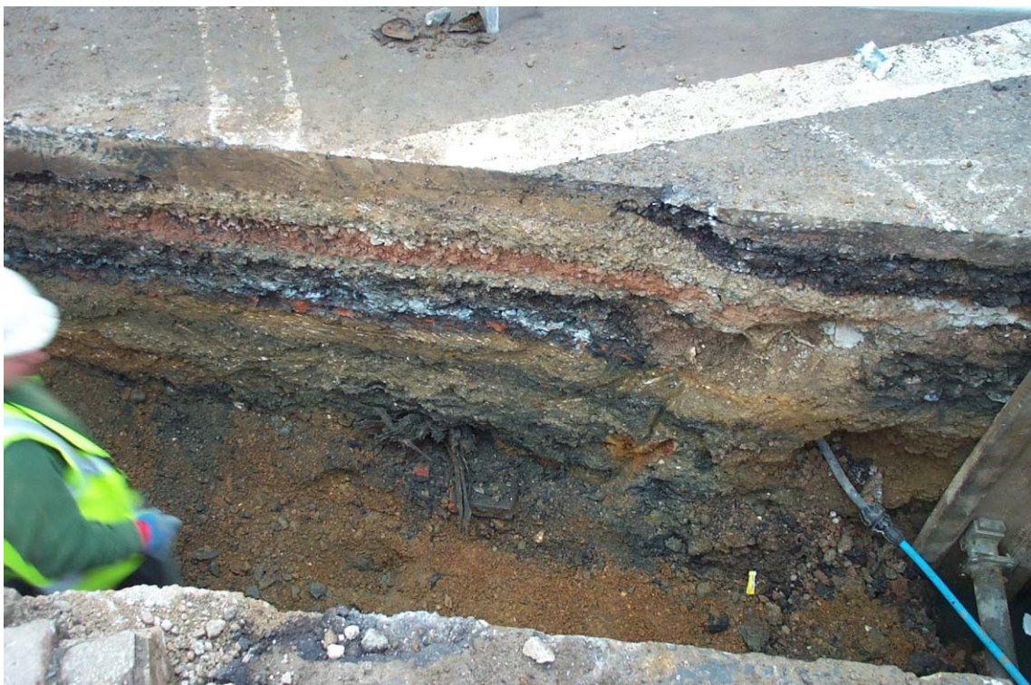
Plate 2: The succession of 20 th century High Street surfaces and 19 th century drain
