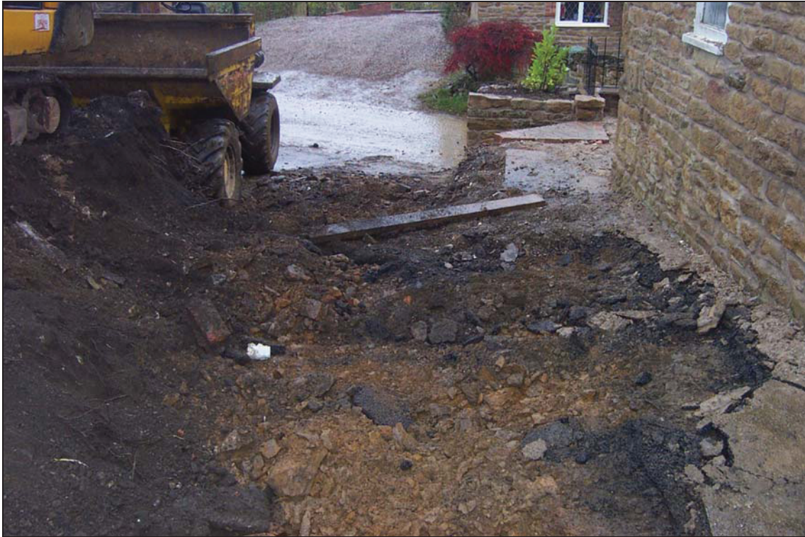
Plate 3: Excavation of the garage footprint
