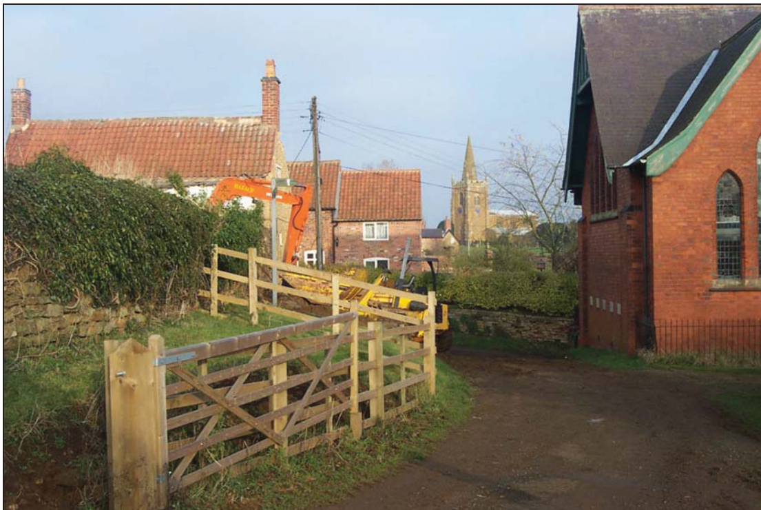
Plate 4: Terracing on the south-east side of the site
