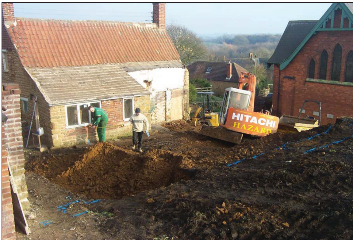
Plate 2: Excavation of the footprint of the extension
