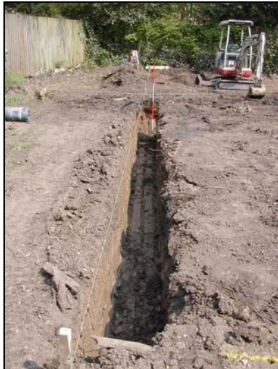
Plate 1: Northern footing looking eastwards
