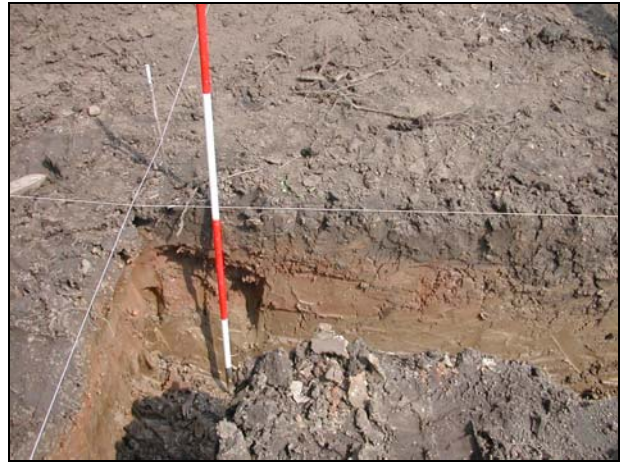
Plate 2: North west corner of foundations
