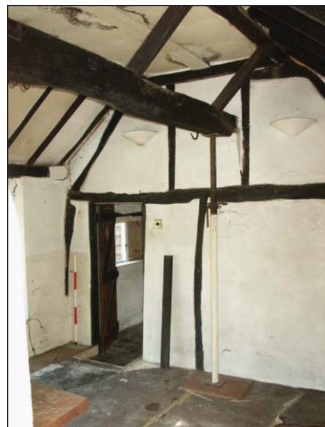
Plate 12: Ground floor, south room, view north
