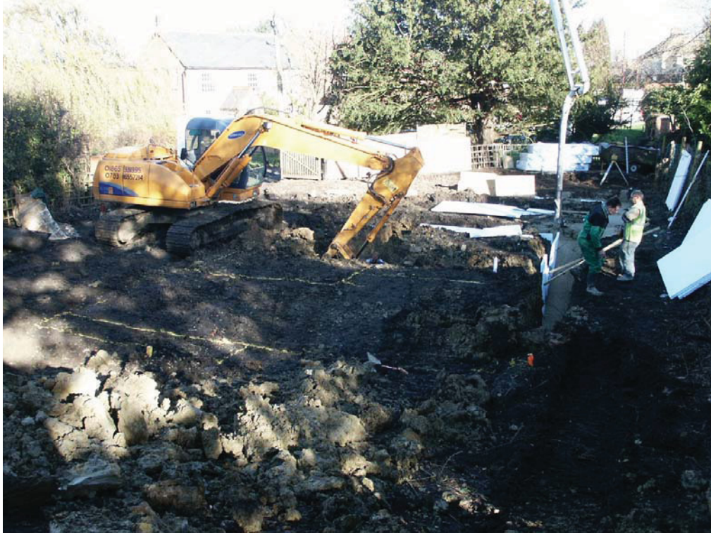
Plate 13: General view of site during groundworks
