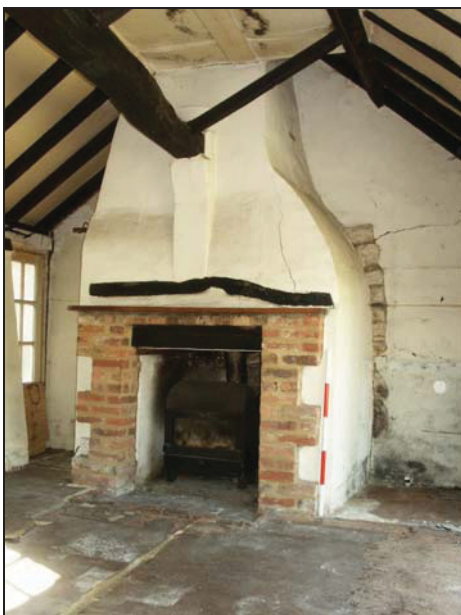
Plate 11: Ground floor, south room, view south.
