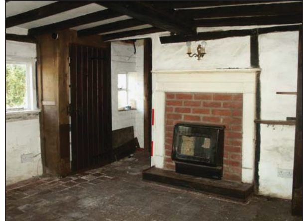
Plate 4: Ground floor, north room, view NW
