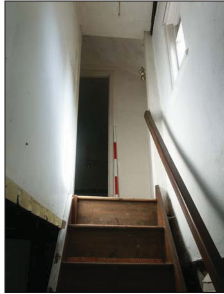
Plate 8: Stairs and landing
