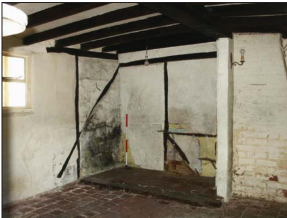
Plate 5: Ground floor, north room, view SE
