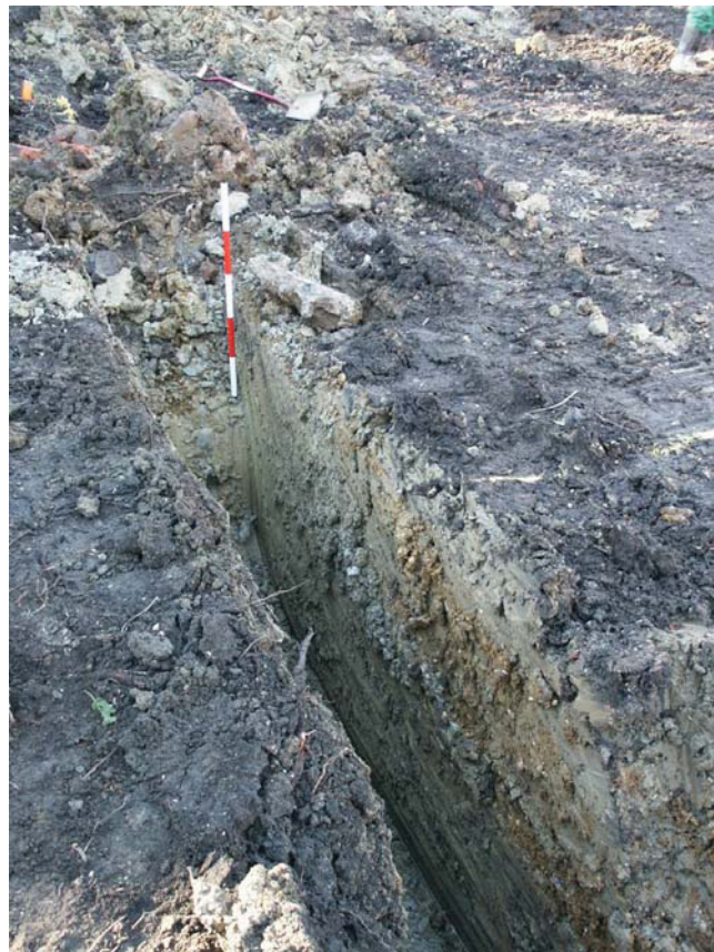
Plate 14: Typical soil profile in footing trench (east side)
