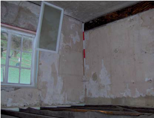
Plate 9: Room 3, looking north west
