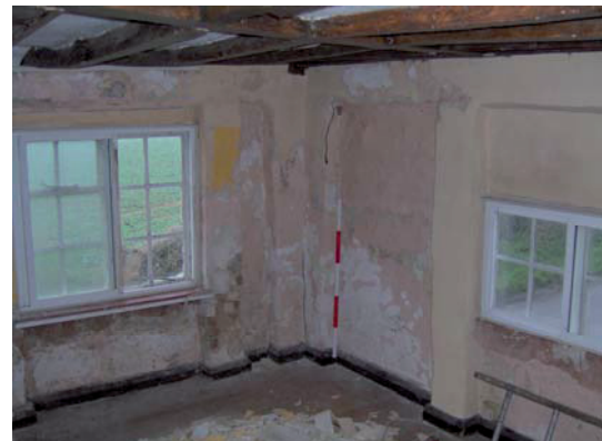
Plate 12: Room 4, looking north west
