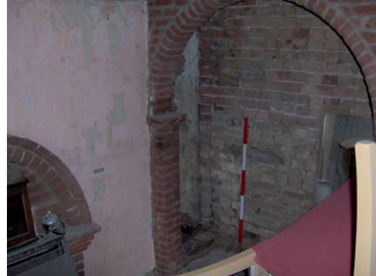
Plate 8: Room 2, looking north east
