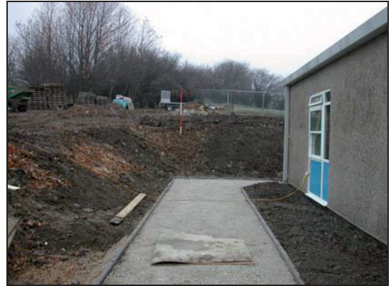
Plate 2: New terraced area looking north towards location of the ditch.
