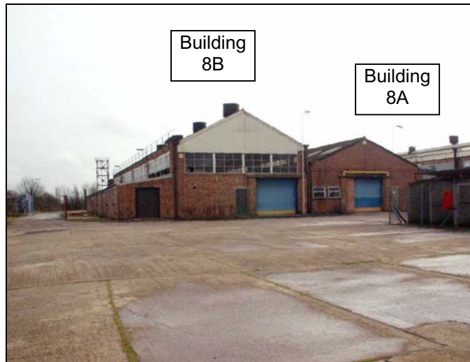
Plate 111: The west elevation of Building 8. February 2005
