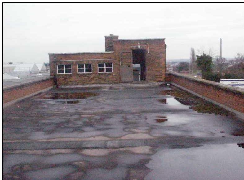
Plate 74: Roof of the Service Sales Division. February 2005
