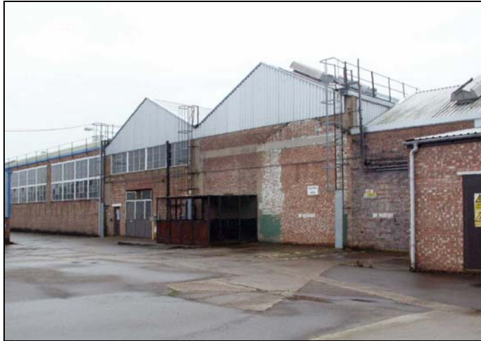
Plate 36: Central area of north wall of Building 2
