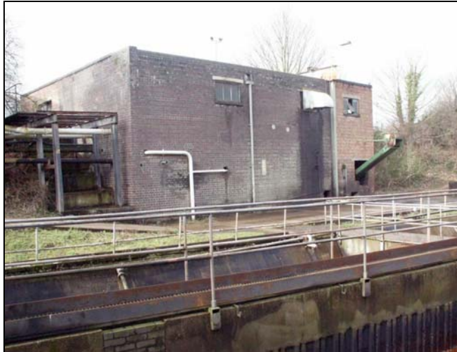
Plate 123: North East elevation of Building 10 (later Extension visible to right). February 2005
