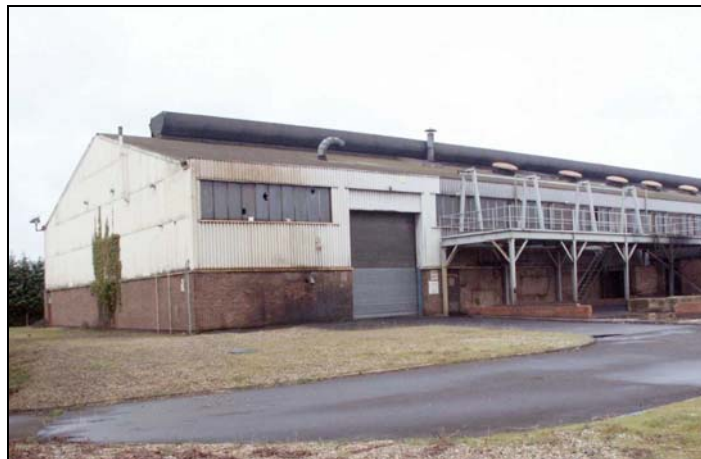
Plate 76: The south side of Building 3. February 2005
