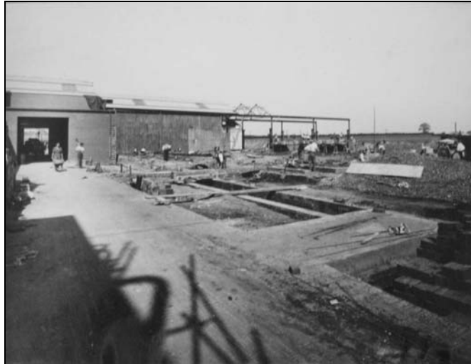
Plate 27: Hardening Shop and Press Shop during construction. 9 th June 1942
