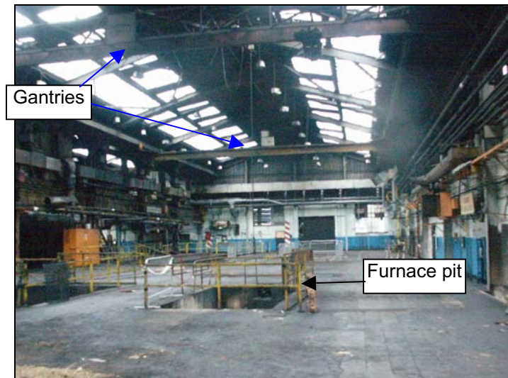
Plate 98: The east bay (Heat Treatment Works) in Building 5. February 2005
