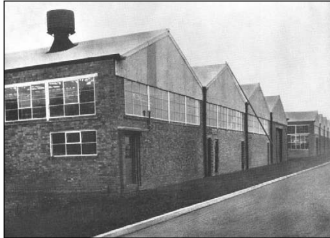
Plate 60: West elevation of the Hardening Shop following completion of the 1950 extension
