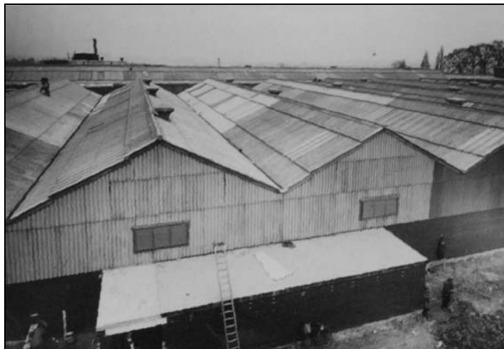
Plate 22: The southwest area. 21 st April 1942. Grinding Shop
