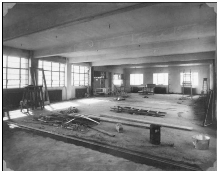
Plate 6: Dining Room 2 and the Kitchen under construction (5 May 1942)
