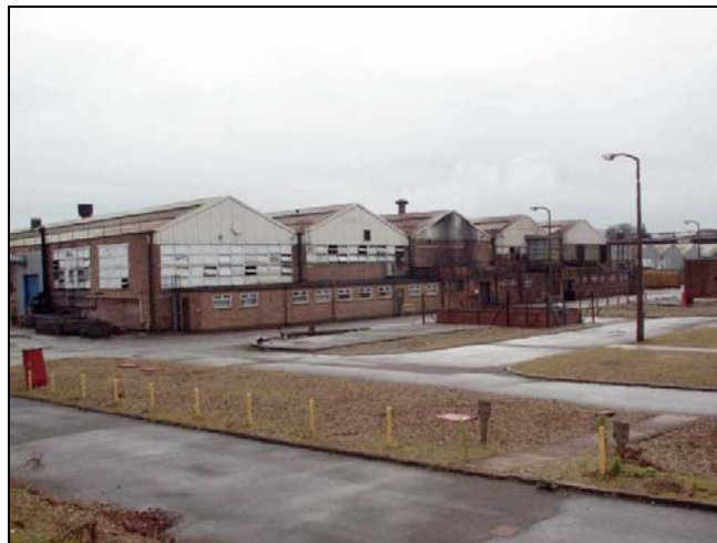
Plate 61: West elevation of the Hardening Shop in its final form. February 2005
