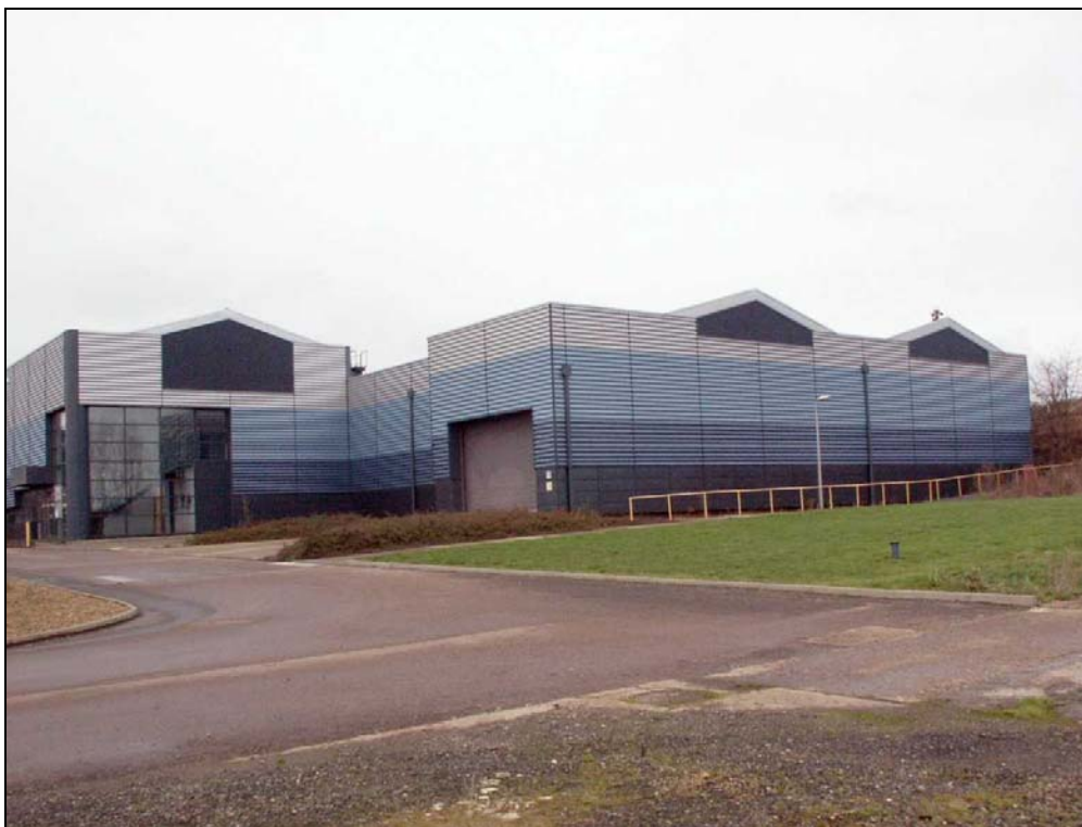
Plate 101: View of the east end of Building 6. February 2005
