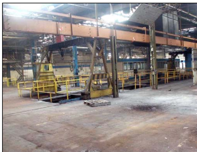
Plate 62: Site of the Pit Furnaces showing Gantry and Crane. February 2005
