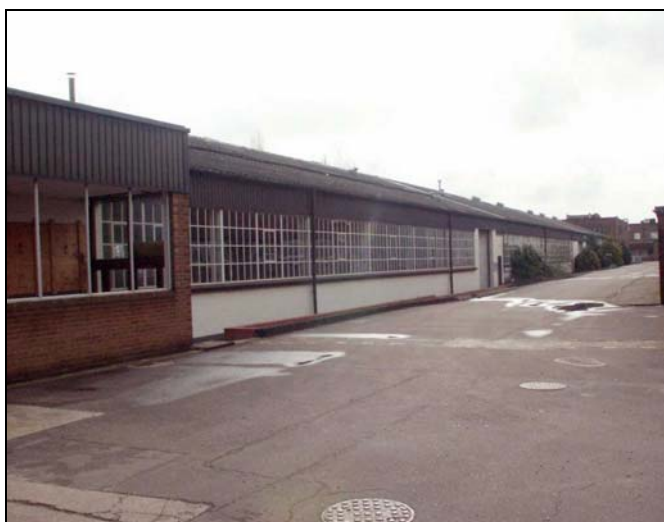
Plate 116: West elevation of Building 9. February 2005
