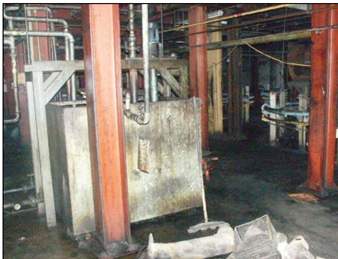
Plate 81: The cellar in Building 3. February 2005
