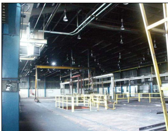
Plate 82: The south part of Building 3. February 2005
