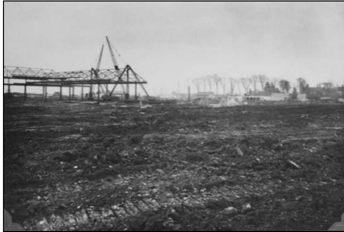
Plate 18: Building 2 during the early part of construction. 5 th December 1941
