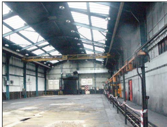
Plate 99: West bay of Building 5. February 2005
