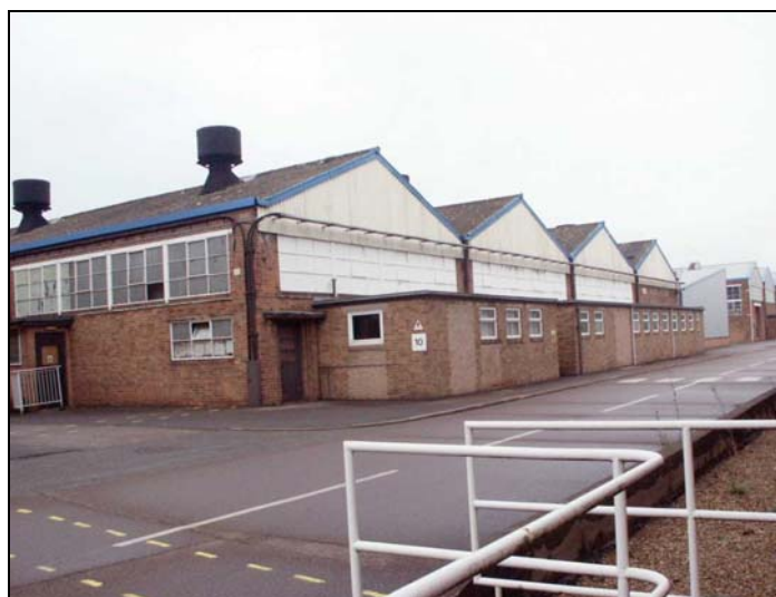
Plate 38: East elevation of Building 2. February 2005
