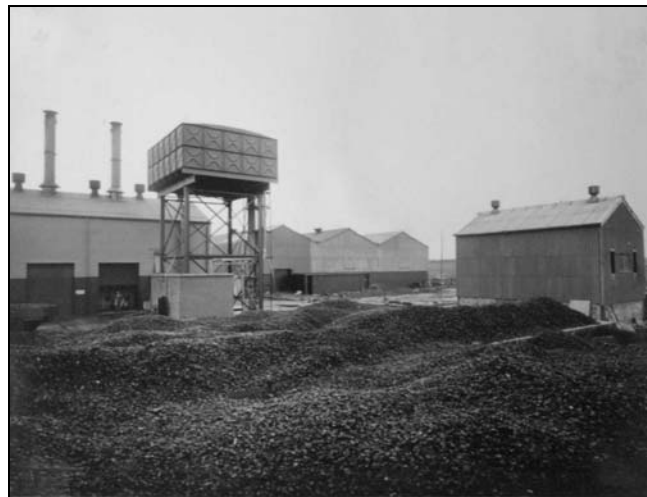
Plate 46: View towards west end of the northeast area. Gas Producer House on left, water tower central and boiler house to left. 3 rd November 1942
