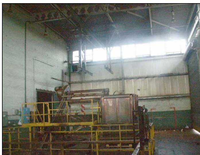
Plate 83: The Suds House in Building 3. February 2005
