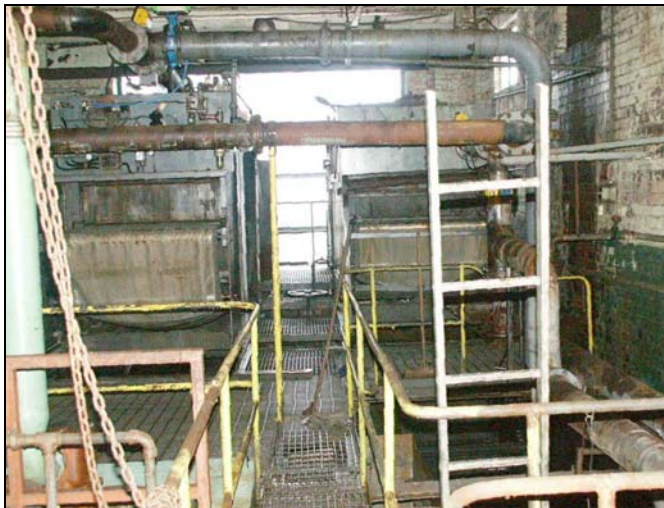
Plate 124: Internal detail of Building 10. February 2005
