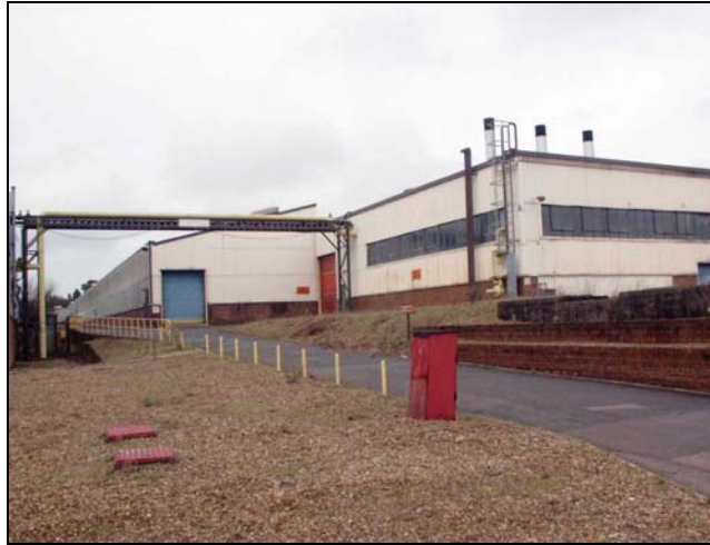
Plate 85: East end of Building 4 showing the southern extension. February 2005
