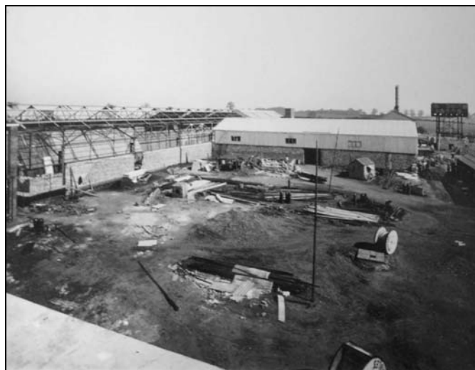
Plate 25: Tool Shop construction 9 th June 1942
