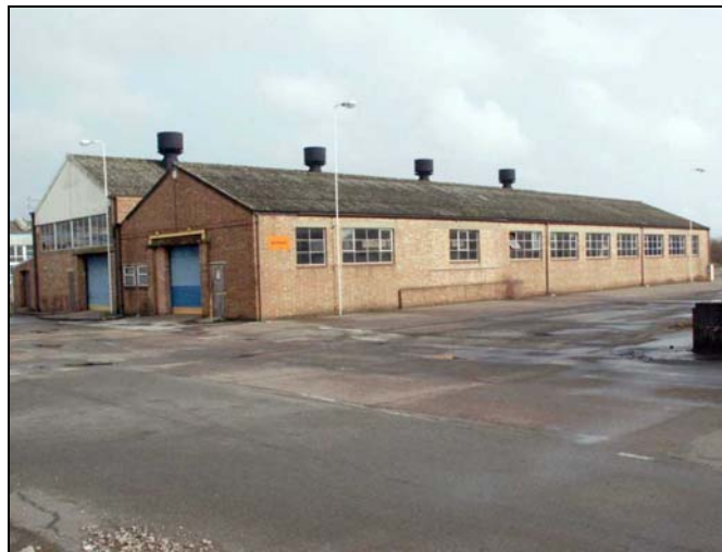
Plate 112: Building 8 south and west elevations. February 2005
