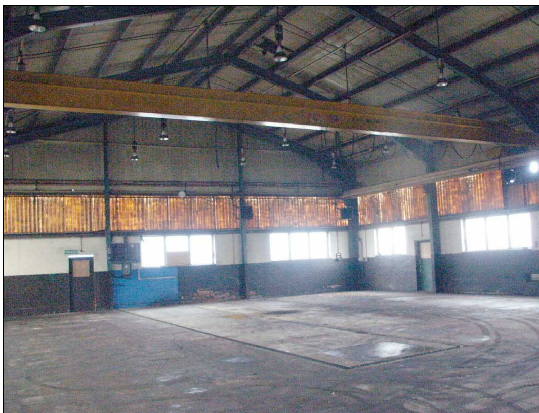
Plate 93: Storage Building between Buildings 4 and 5. February 2005
