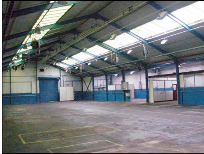
Plate 114: Building 8 internal view looking west. February 2005
