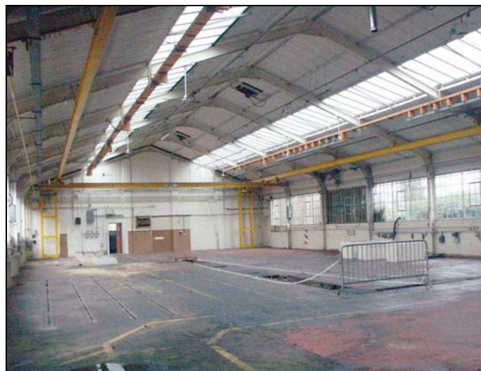
Plate 119: North room in Building 9. February 2005
