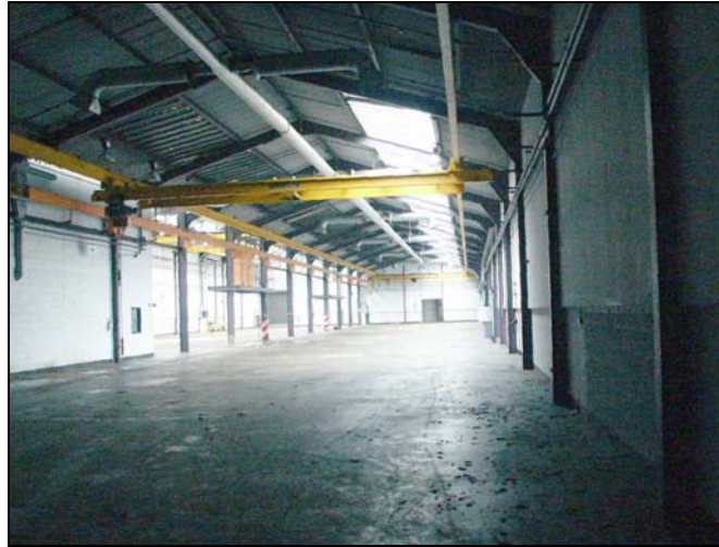
Plate 102: Internal view of Building 6, looking west. February 2005
