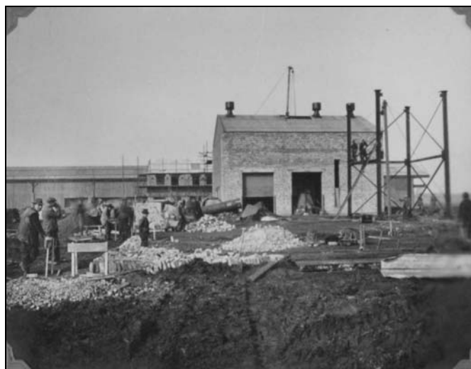
Plate 44: The Boiler House and Water Tower. 10 March 1942
