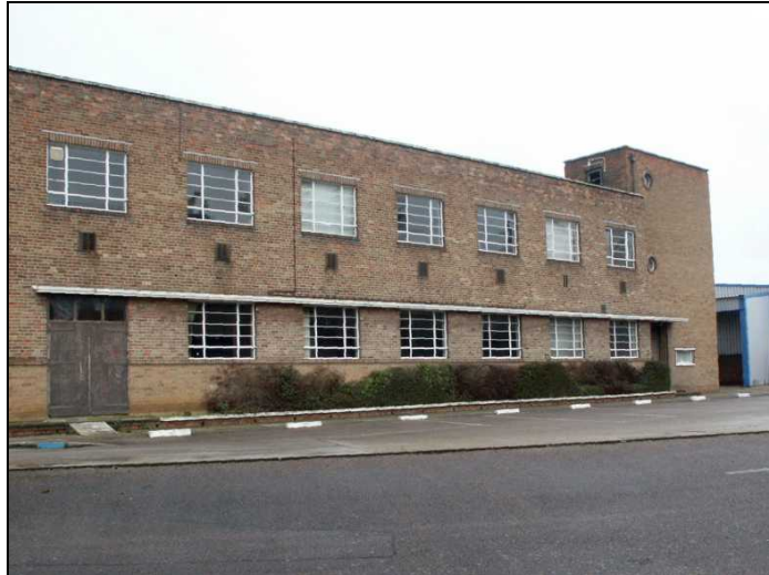
Plate 69: South elevation of the Service Sales Department. February 2005
