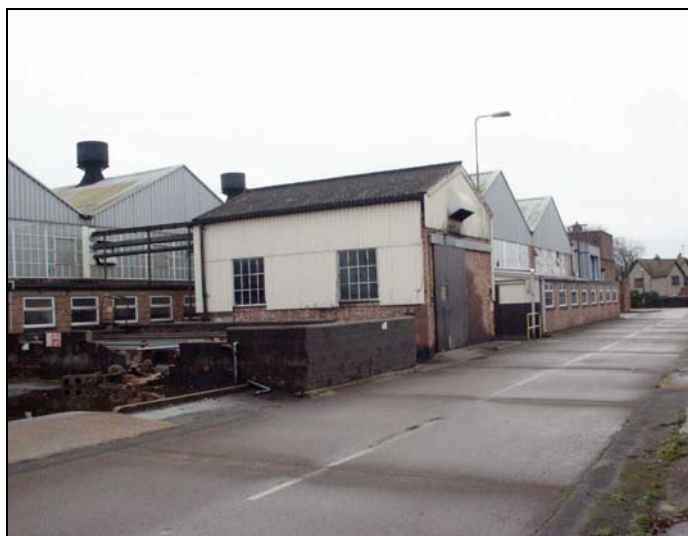
Plate 35: General view of the west side of Building 2. February 2005
