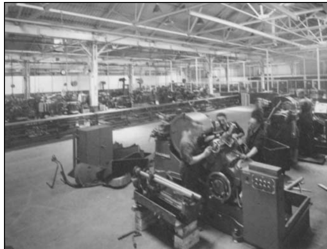
Plate 31: View of the Grinding Shop I in August 1943
