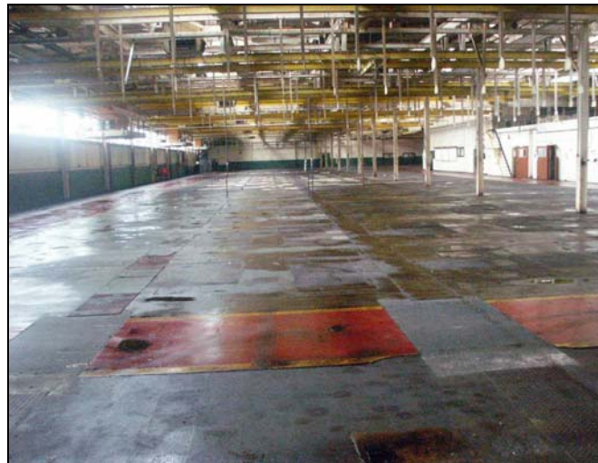
Plate 86: Internal view of Building 4, looking east. February 2005
