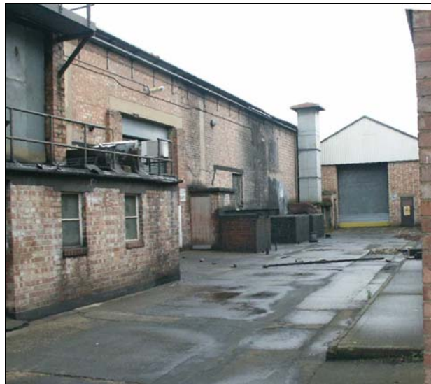
Plate 55: South elevation of the Hardening Shop. February 2005
