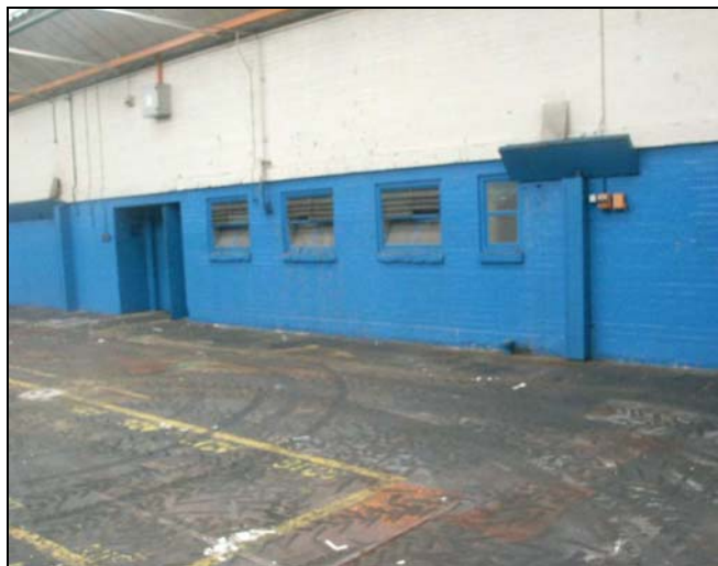
Plate 43: The Green and Black Store, showing detail of the service rooms along the original west wall of the Press Shop
