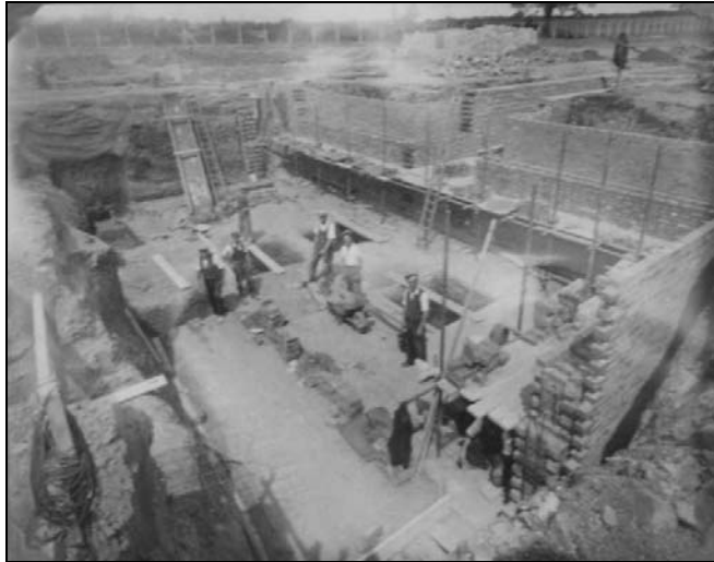
Plate 57: Constructing the Hardening Shop. The excavations for the Substation. 30 June 1942
