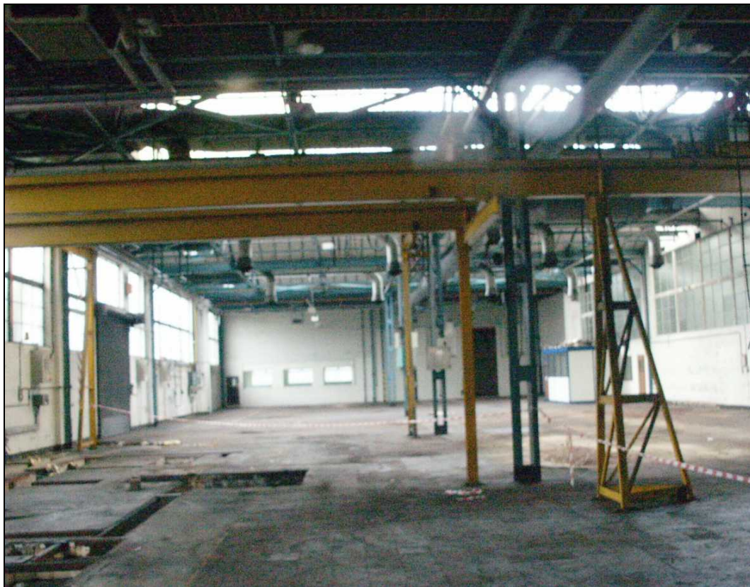
Plate 107: The Auto Shop in Building 7. February 2005
