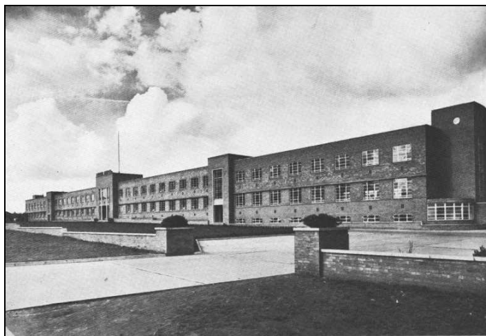
Plate 13: South façade of the Admin Block after completion of the 2 nd extension in 1957
