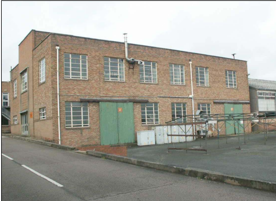
Plate 120: External view of the Metallurgical Laboratory. February 2005
