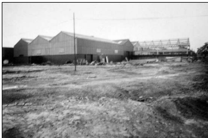
Plate 20: The northeast area during construction 3 rd November 1942
