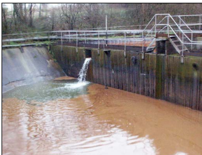
Plate 125: The Catchment Pits. February 2005
