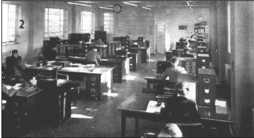
Plate 72: Main Office on the First Floor (1949)
