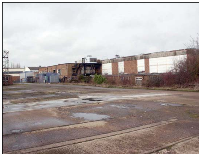
Plate 104: Building 7. View of the south facing elevation. February 2005
