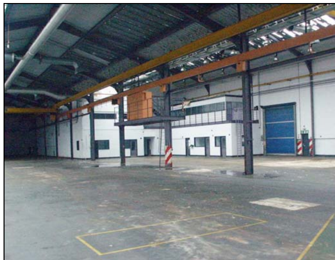
Plate 103: Internal view of Building 6, looking east. February 2005
