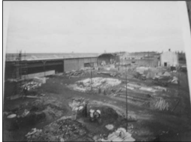
Plate 24: Southeast area (Tool Shop), during construction. 24 th February 1942
