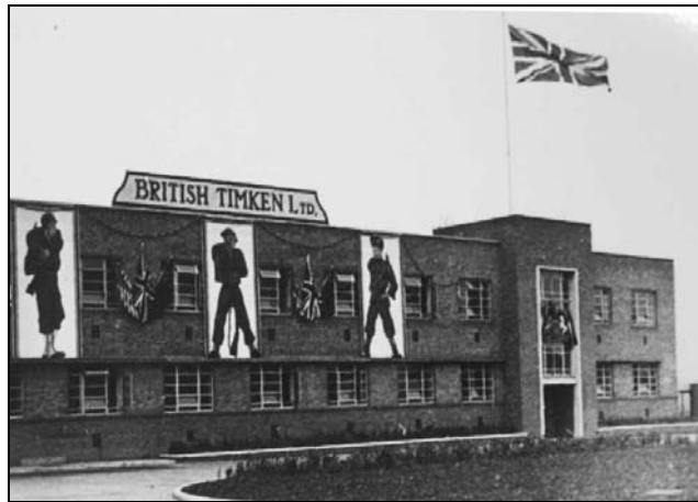
Plate 8: VE Day decorations on the Administration Block (May 1945)
