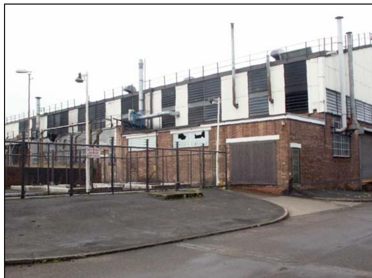
Plate 97: East elevation of Building 5. February 2005
