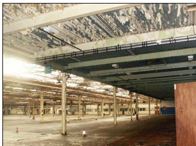
Plate 50: The Grinding Shop with flat roofed extension to right. Feb. 2005
