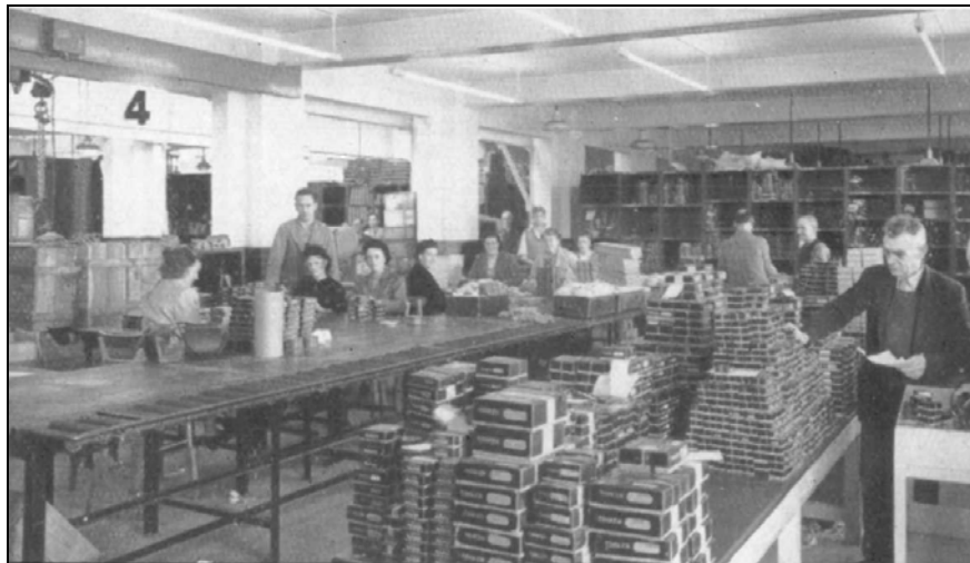
Plate 73: Receiving and Wrapping Department on the Ground Floor (1949)
