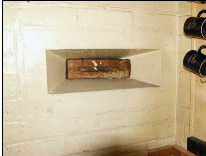
Plate 5: Gun slit at the base of the Administration Block Tower (Feb 2005)
