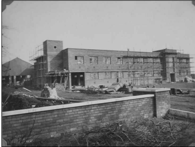
Plate 3: The Administration Block during construction in 1942
