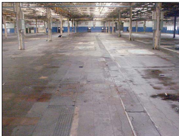
Plate 41: View west through the Grinding Shop. February 2005
