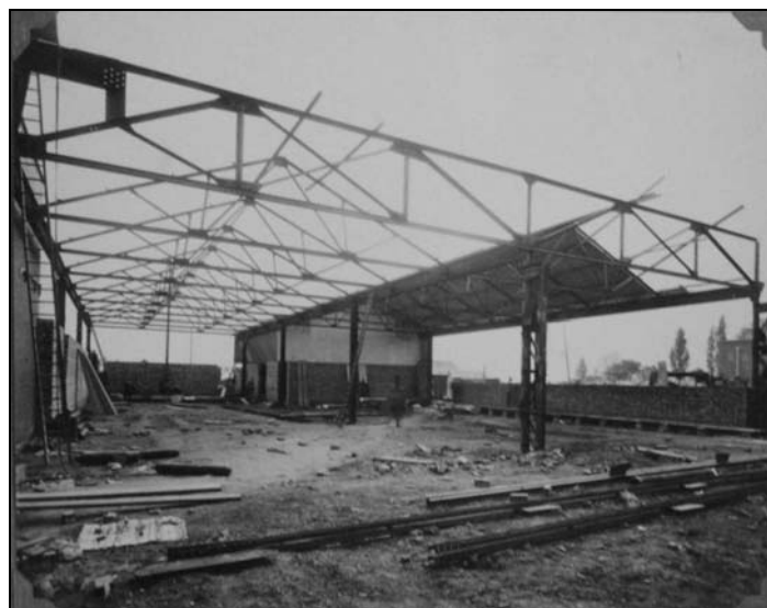
Plate 26: Tool Shop construction. Internal view. 26 May 1942
