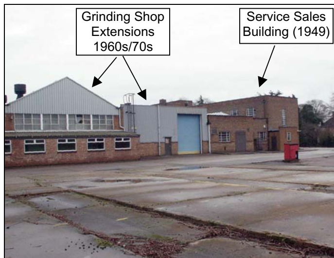
Plate 34: The south west corner of Building 2. February 2005
