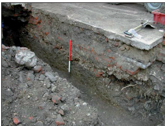
Plate 11: New western N-S foundation of new building (Section 3)
