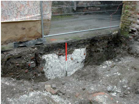
Plate 3: Detail of new eastern foundation
