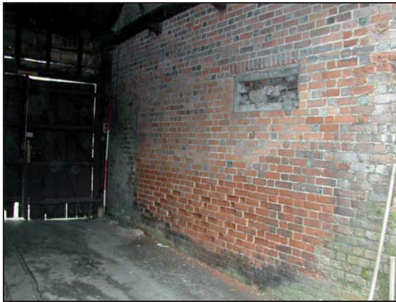
Plate 9: Detail of external east wall of existing building
