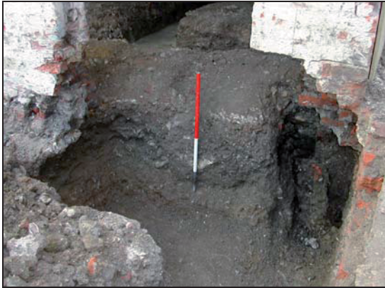
Plate 13: NW foundation of existing building (Section 5)
