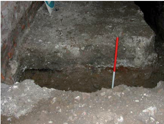
Plate 21: Detail of eastern end of internal E-W foundation (Section 1)
