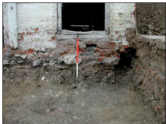
Plate 18: Original NW foundation of building (note the puddingstones in the footings)
