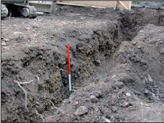
Plate 19: Detail of eastern end of E-W foundation (Section 4)
