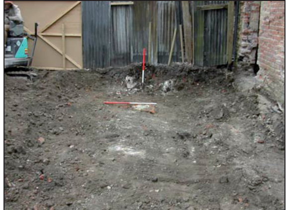
Plate 2: Detail of end of new extension
