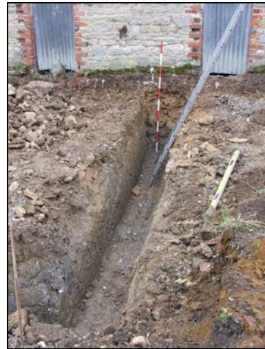
Plate 4: Western footing trench of extension
