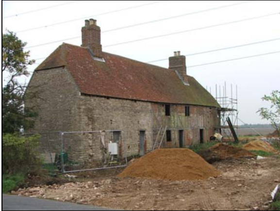
Plate 1: View of cottages, looking southwest
