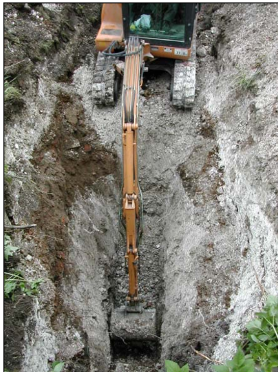
Plate 1: View looking south along the axis of the trench
