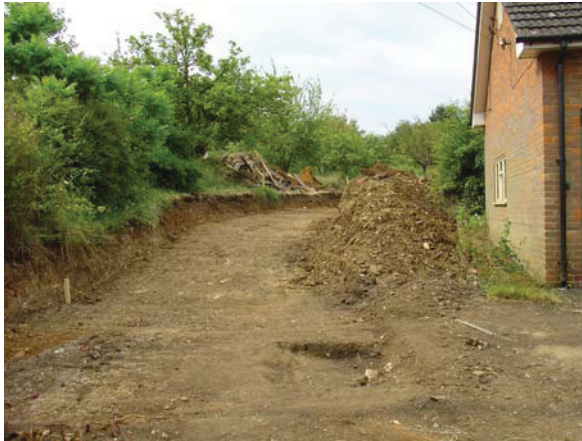
Plate 1: Trench from Chapel Lane, facing southwest
