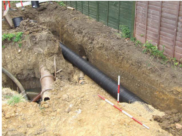
Plate 4: Storm drain trench, facing WSW
