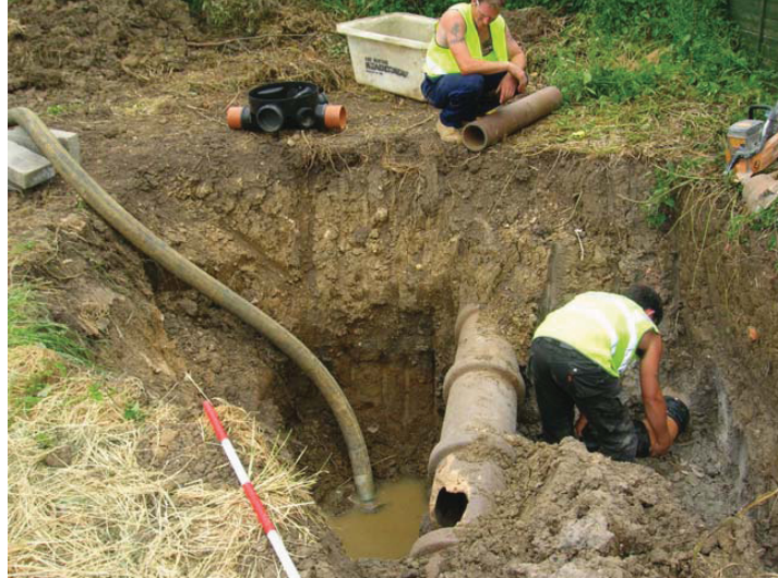
Plate 1: Pit 1, facing SW
