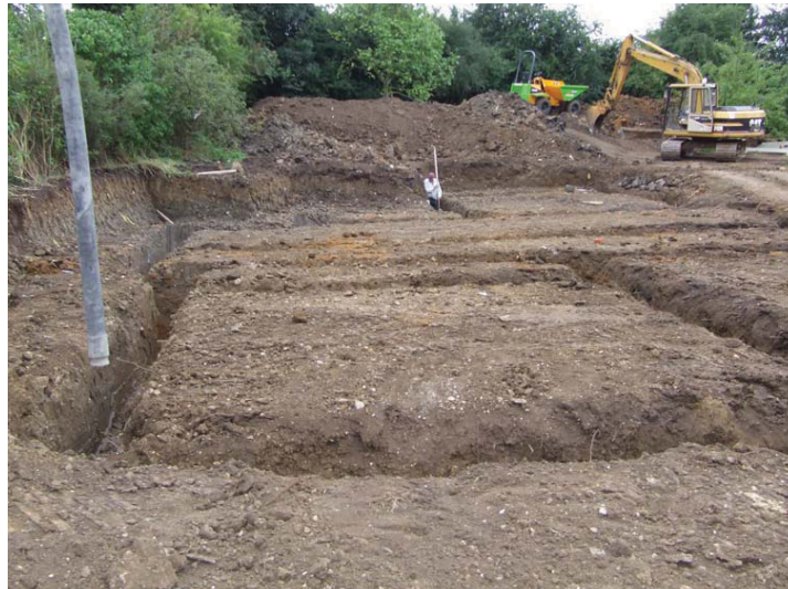
Plate 11: Plot 1 after levelling and excavation of footings, facing SW
