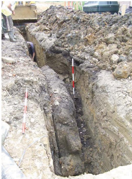
Plate 7: Northern part of eastern sewer trench, facing WSW
