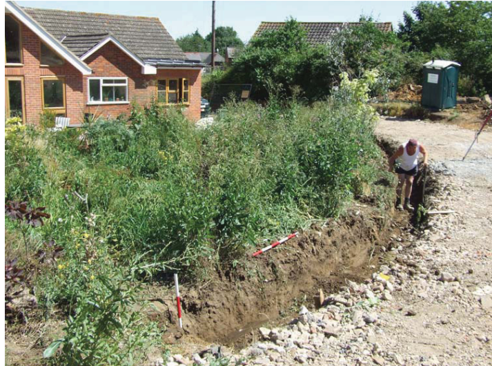
Plate 10: Boundary wall footing trench, facing NE
