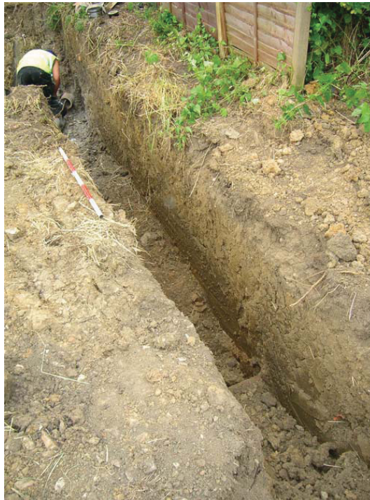
Plate 2: Western sewer trench, facing WSW
