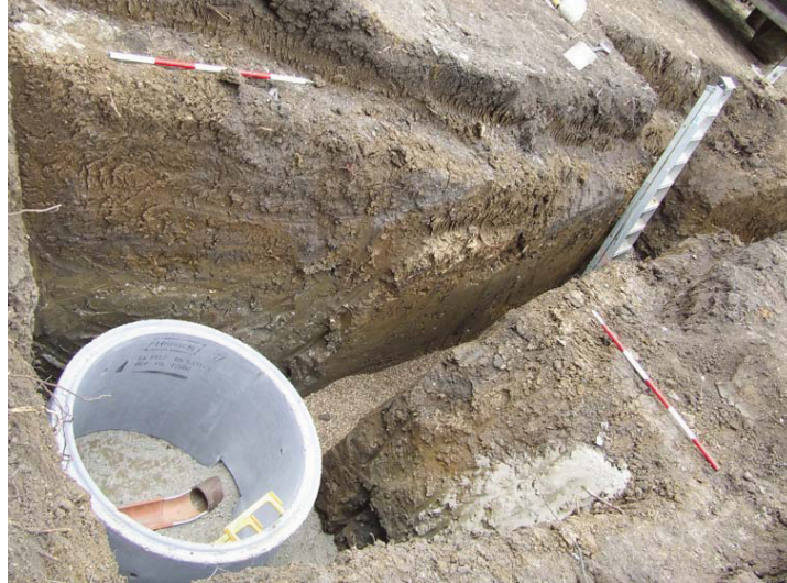
Plate 6: Southern part of eastern sewer trench and Pit 5, facing NW
