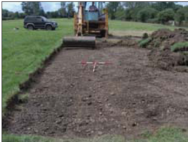
Plate 6: North west end of site, looking west
