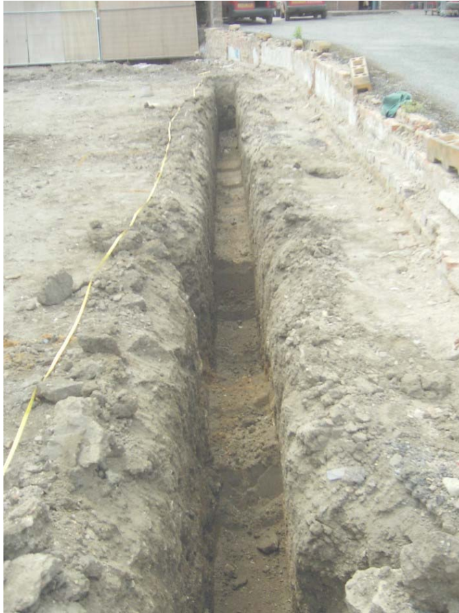
Plate 1: General view of footing Trench 1
