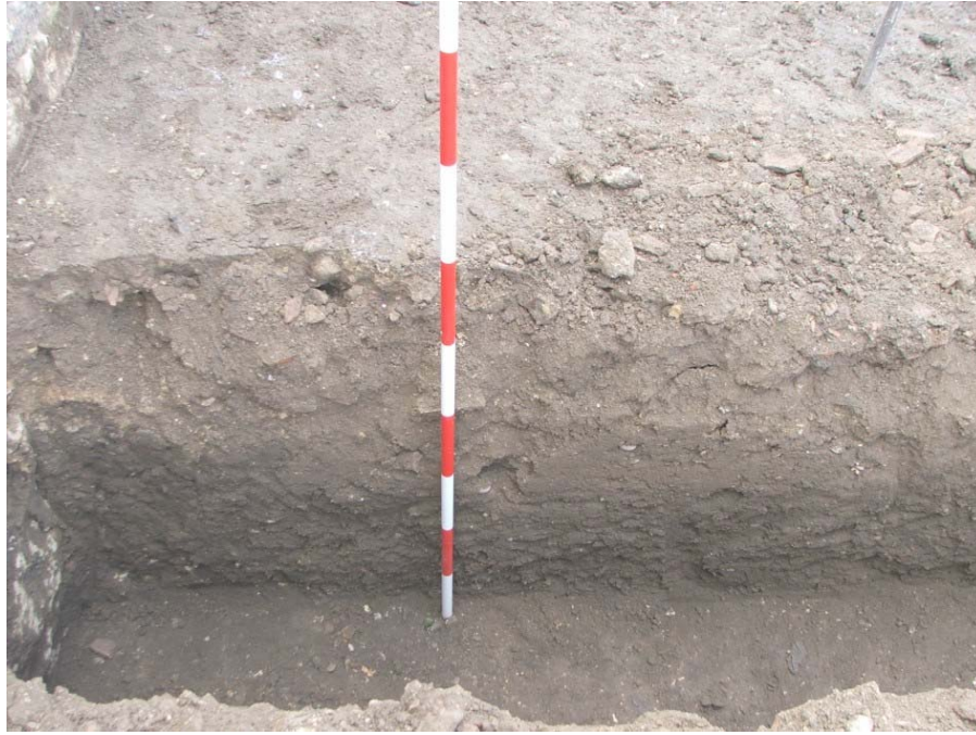
Plate 3: Footing Trench 2 showing the depth of overburden
