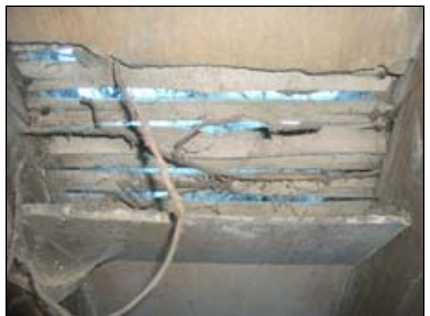
Plate 24: Internal view of the lath & plaster
