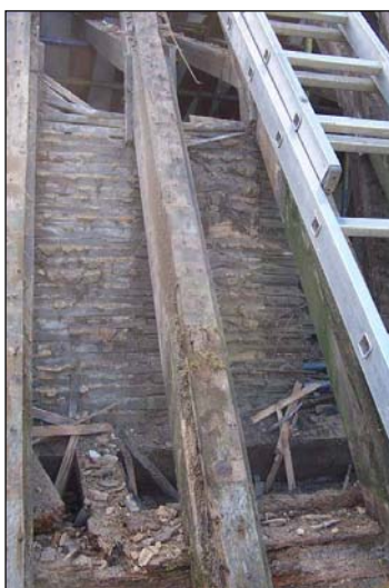
Plate 23: External view of the lath & plaster
