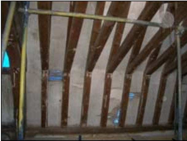
Plate 13: Ceiling over the chancel
