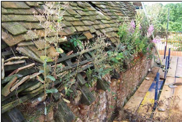
Plate 21: Chancel roof, north side
