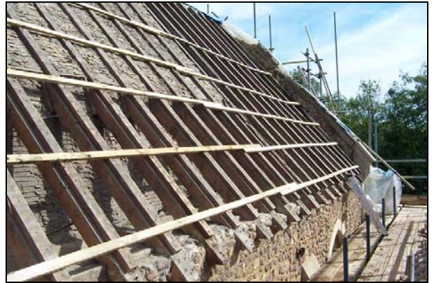
Plate 20: Stripped chancel roof, south side
