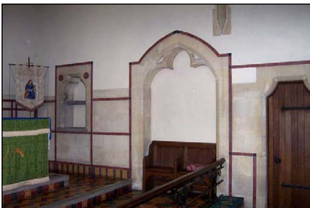
Plate 35: South-east corner of Hadstock chancel
