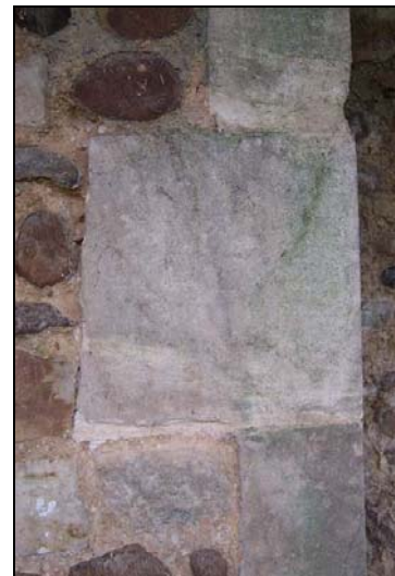
Plate 10: Stone dressing to chimney
