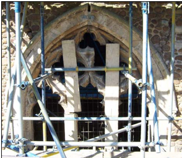
Plate 9: Hood mould over the East window
