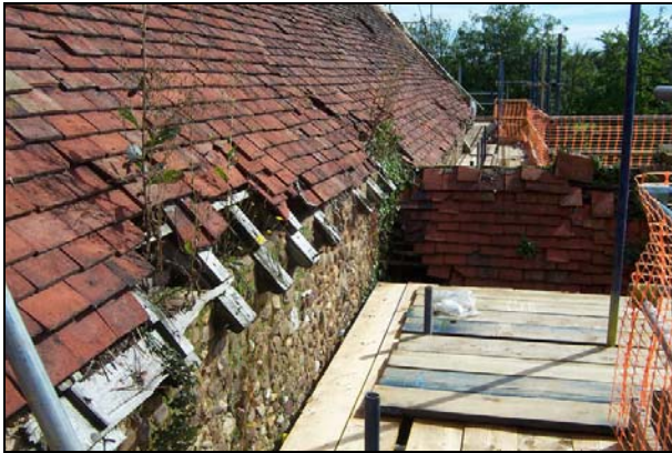
Plate 19: South side of the roof
