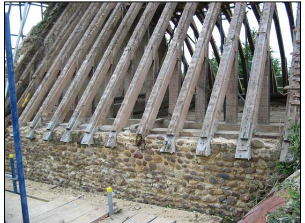
Plate 22: Stripped nave roof west of the porch
