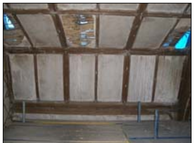
Plate 12: Panelling in the Sanctuary ceiling
