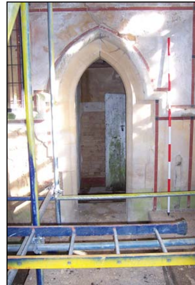
Plate 16: Wall decoration around the vestry door
