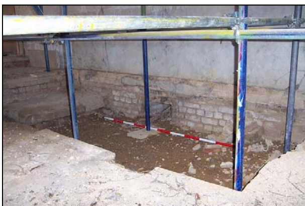
Plate 11: Brickwork at the base of the south chancel wall
