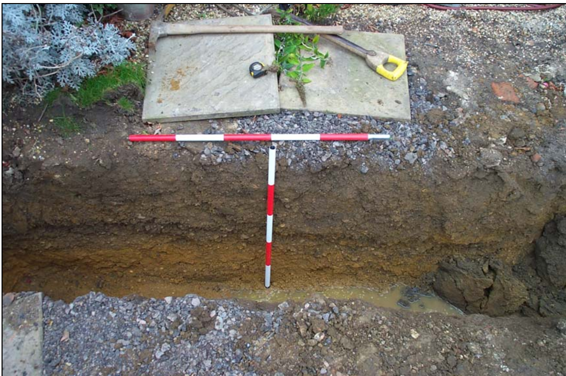
Plate 2: Typical Section of Foundation Trench ( Scales: 1m )
