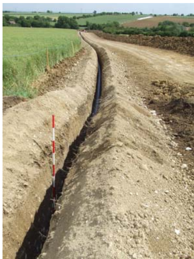
Plate 5: Pipe trench facing SE toward site compound
