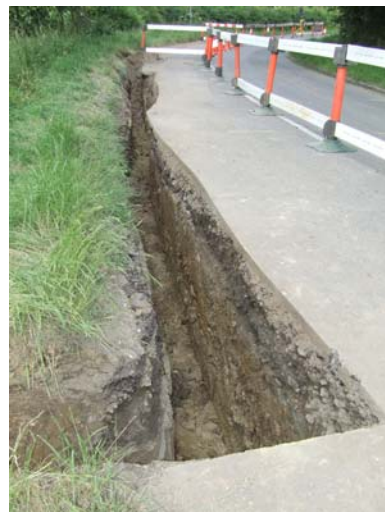
Plate 6: Pipe trench on Wilden High Street facing E
