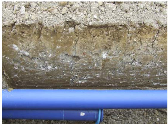
Plate 4: Natural strata and 280mm water main
