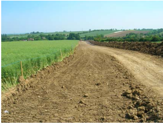
Plate 1: Pipeline easement stripped of topsoil facing SE toward site compound
