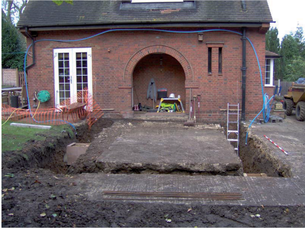
Plate 1: The foundation trench, looking north west
