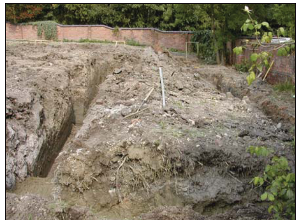
Plate 6: Footing trench for Stud Cottage, view east 09/09/05
