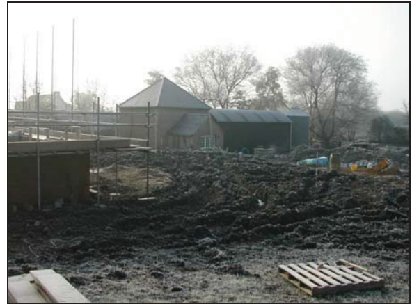
Plate 2: Stud Cottage site, view south east
