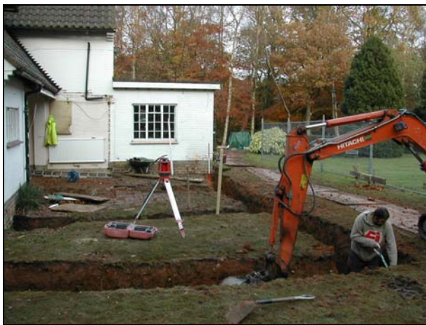
Plate 5: Trench 4 looking NE
