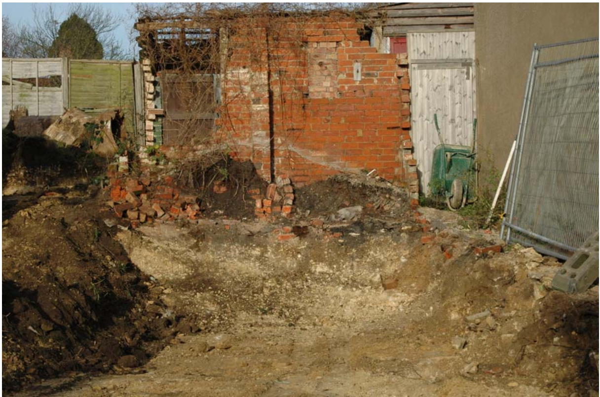
Plate 2: The extant north wall of the cottage.
