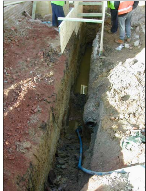
Plate 2: North footing trench
