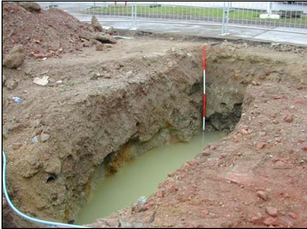
Plate 1: East footing trench
