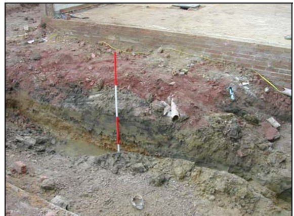
Plate 4: South-west footing trench
