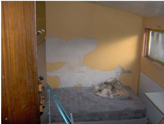
Plate 11: Room 3, looking north
