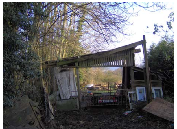
Plate 8: Shed to north east of house
