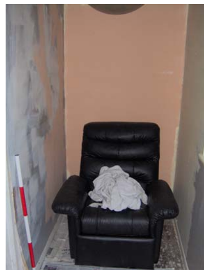
Plate 14: Room 5, looking south
