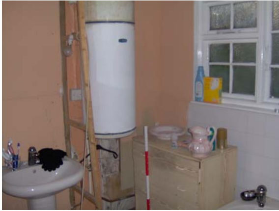
Plate 15: Room 6, looking south west
