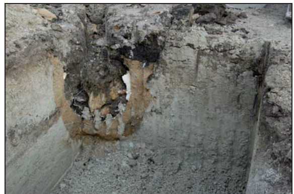
Plate 12: Pit in NW corner of Plots 7&8 soakaway
