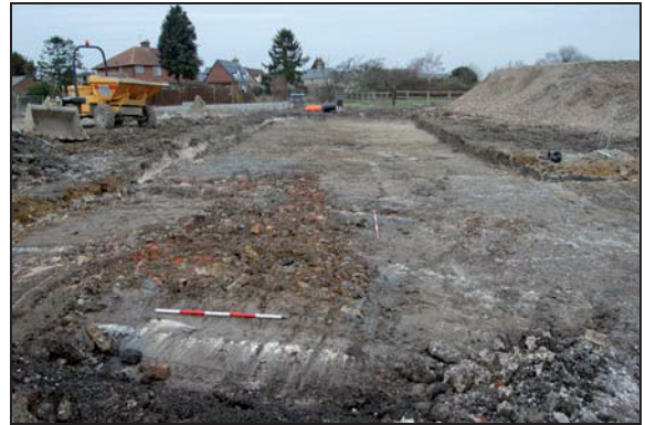
Plate 2: Soakaway 514 in Plots 5 & 6 (looking north)
