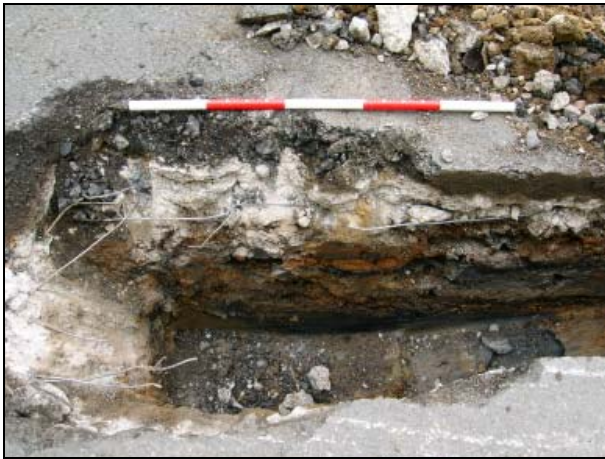
Plate 2: Trench section towards SE end of Earl Street showing layers of ash and brick rubble (1m scale).
