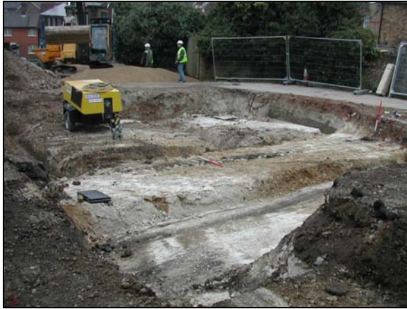
Plate 13: Location of old N-S foundation
