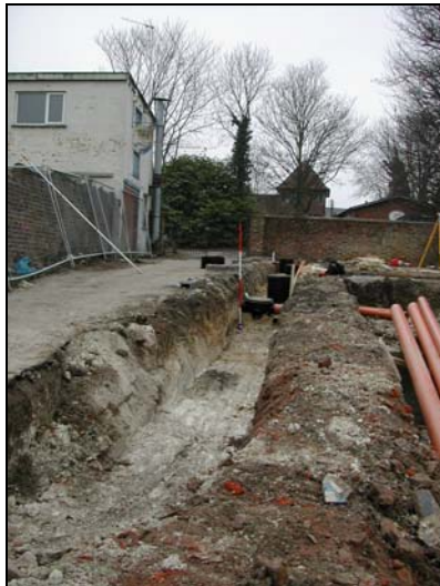
Plate 15: Service trench looking west
