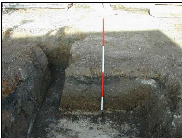
Plate 5: Detail of footings of plot 1 looking north
