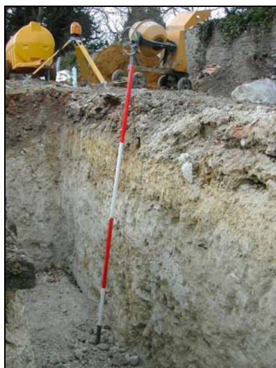
Plate 17: Detail of foundations on north side of 3 rd plot
