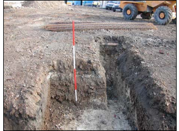
Plate 2: Detail of footings of plot 1 looking east
