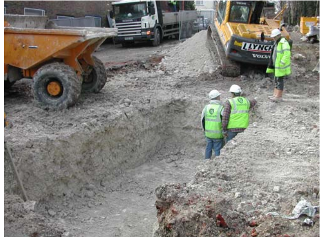
Plate 20: Foundations below footprint of Old Harrow
