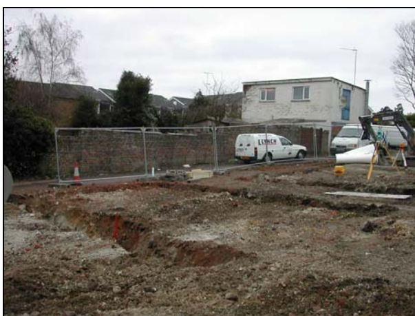
Plate 11: General view of plot 3 looking SW
