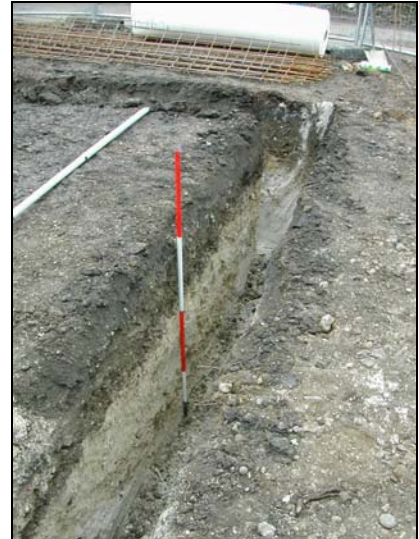
Plate 8: Detail of foundations looking south
