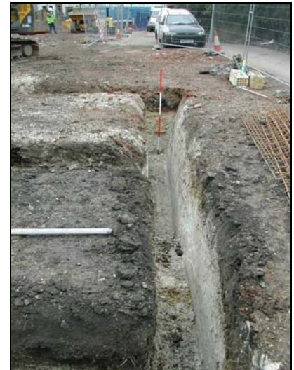
Plate 10: Detail of foundations looking east
