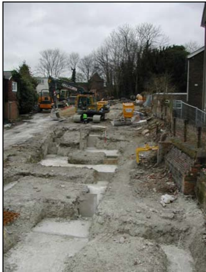
Plate 21: Footings on east side of site
