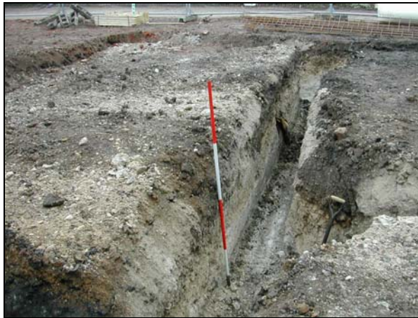
Plate 9: Detail of foundations looking south
