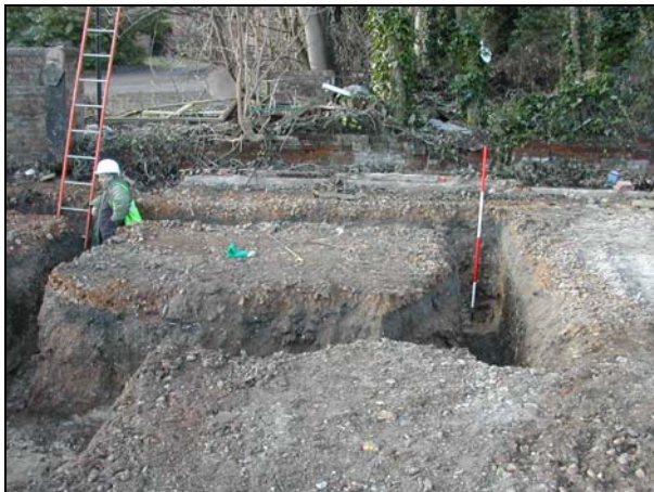
Plate 3: Detail of footings of plot looking west
