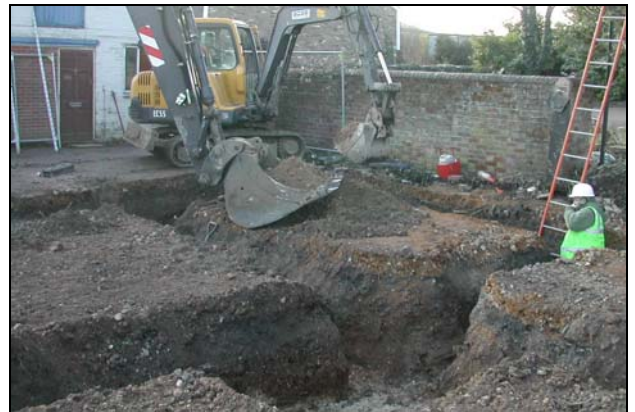
Plate 4: Detail of footings of plot 1 looking SW
