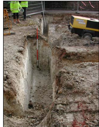
Plate 16: Foundation trench on the east side of 3 rd plot
