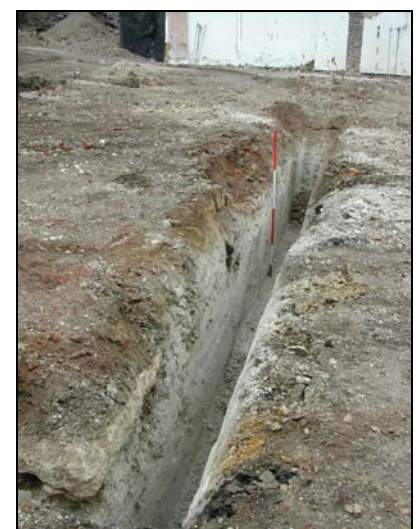
Plate 12: Detail of foundation trench looking north
