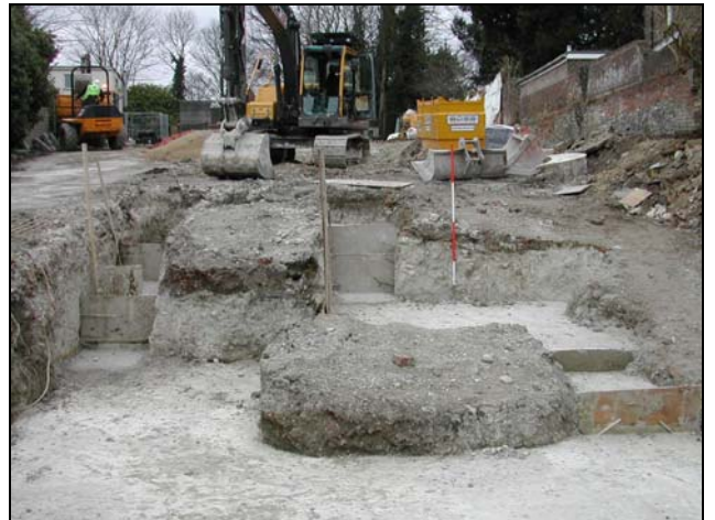
Plate 22: Footings on east side of site
