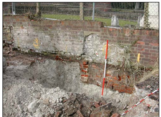
Plate 24: Underpinning of northern boundary wall
