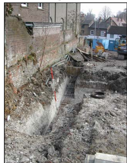
Plate 18: Detail of foundations on north side of 3 rd plot
