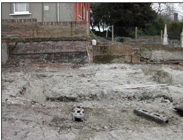
Plate 23: View north across boundary foundations by Baptist chapel
