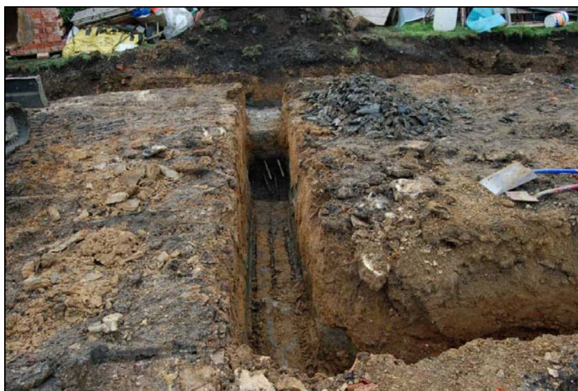
Plate 1: Example of one of the footing trenches
